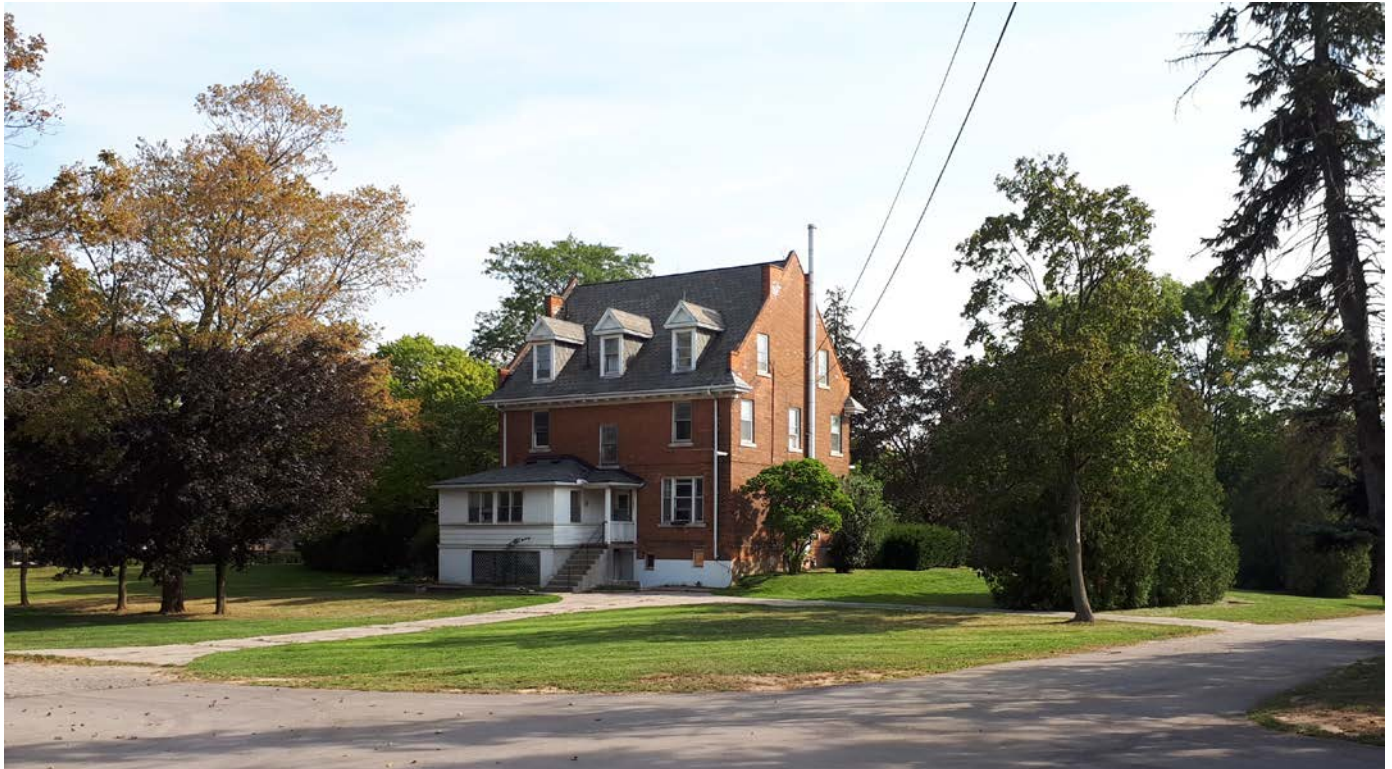
Figure 4: View of the rear of the building (north and west elevations) showing a matching profile with equivalent pedimented dormers. An early one-and-a-half storey aluminum and wooden-clad addition is shown on the eastern portion of the rear façade (2017).
