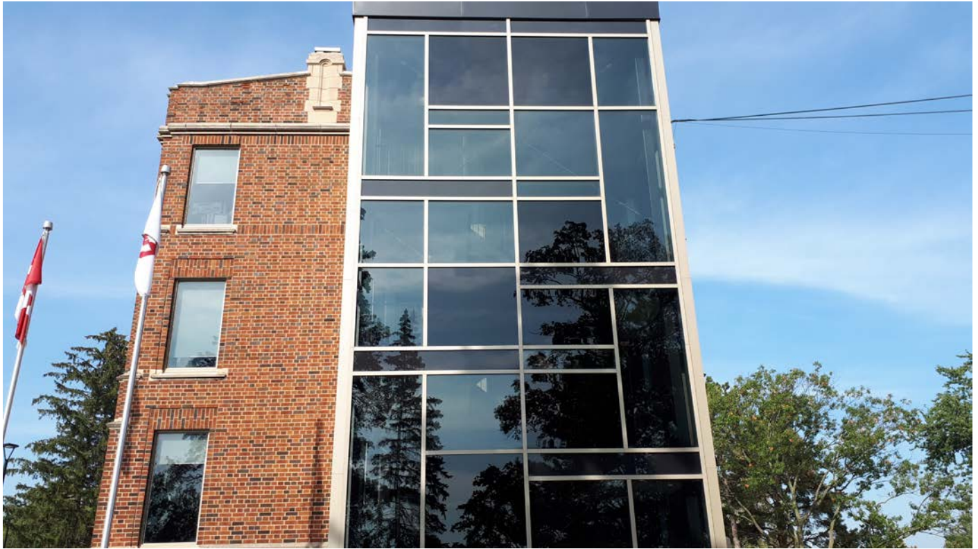
Figure 14: The southern end of the rectangular Patterson Building with a projecting modern glass addition housing a connecting stairwell (2017).
