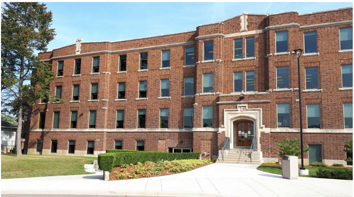
Figure 13: The northern end of the front façade. The building displays a restrained application of the Gothic Collegiate style with roofline enhanced with open stone niches (2017).
