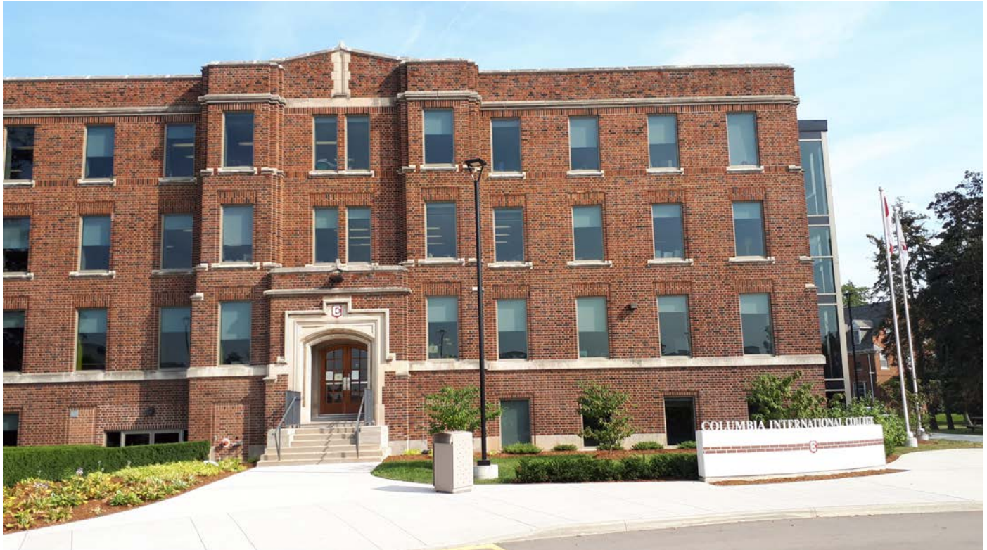
Figure 12: The southern end of the front (west) façade of the Patterson Building now owned and adaptively-reused by Columbia International College. The projected entrance features a subtle ogee arch peak and an attractive hood moulding made of stone (2017).
