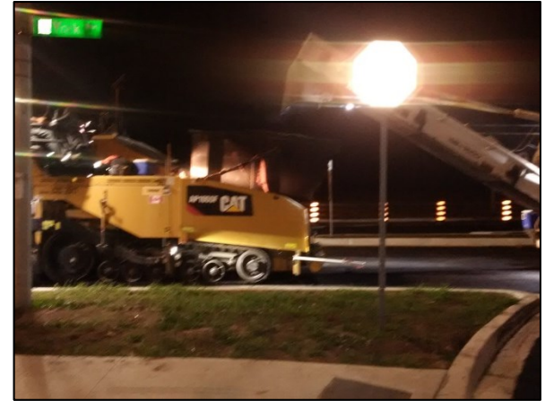
York Boulevard Reconstruction
