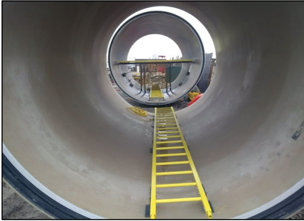
Centennial Sewer Trunk
