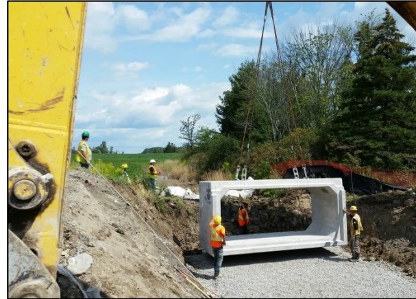
Bell Road Culvert Replacement
