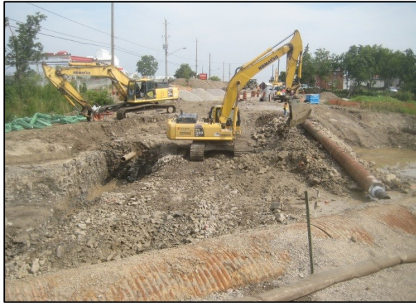
Dartnall Road Culvert
