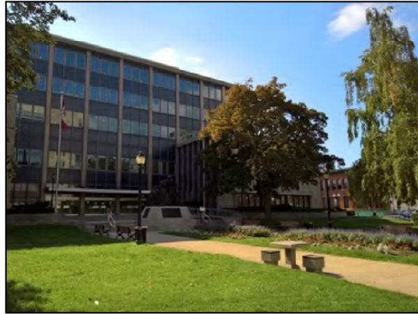
Provincial Offences Building
