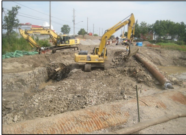
Dartnall Road Culvert
