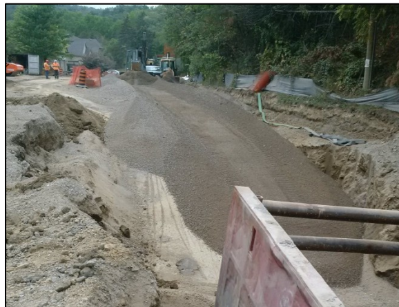
Montgomery Drive Reconstruction
