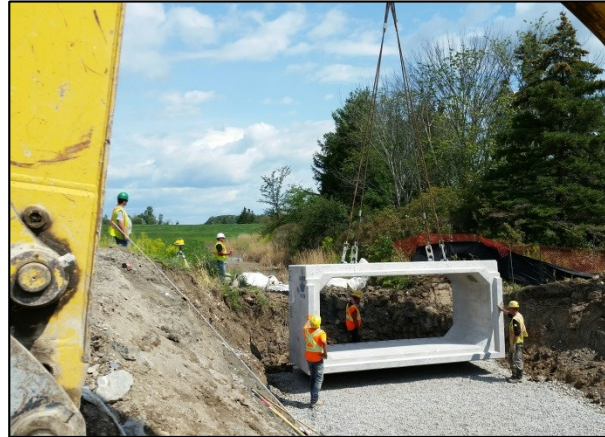
Bell Road Culvert Replacement
