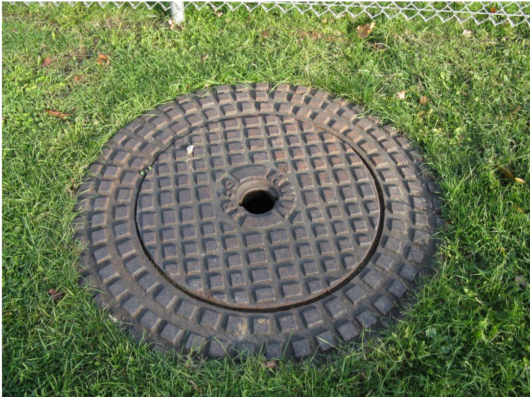
The manhole cover located in front of 201 Robert Street, Hamilton.
