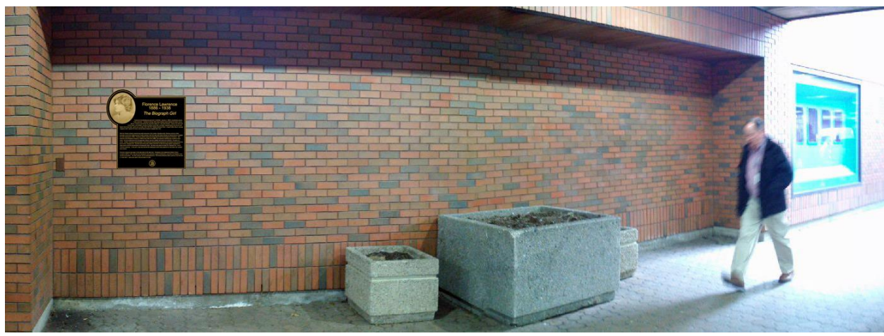
Example of a possible location
