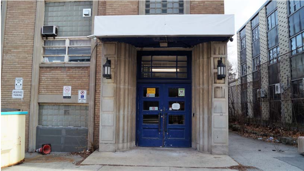
Fig. 73 Entrance into wing
