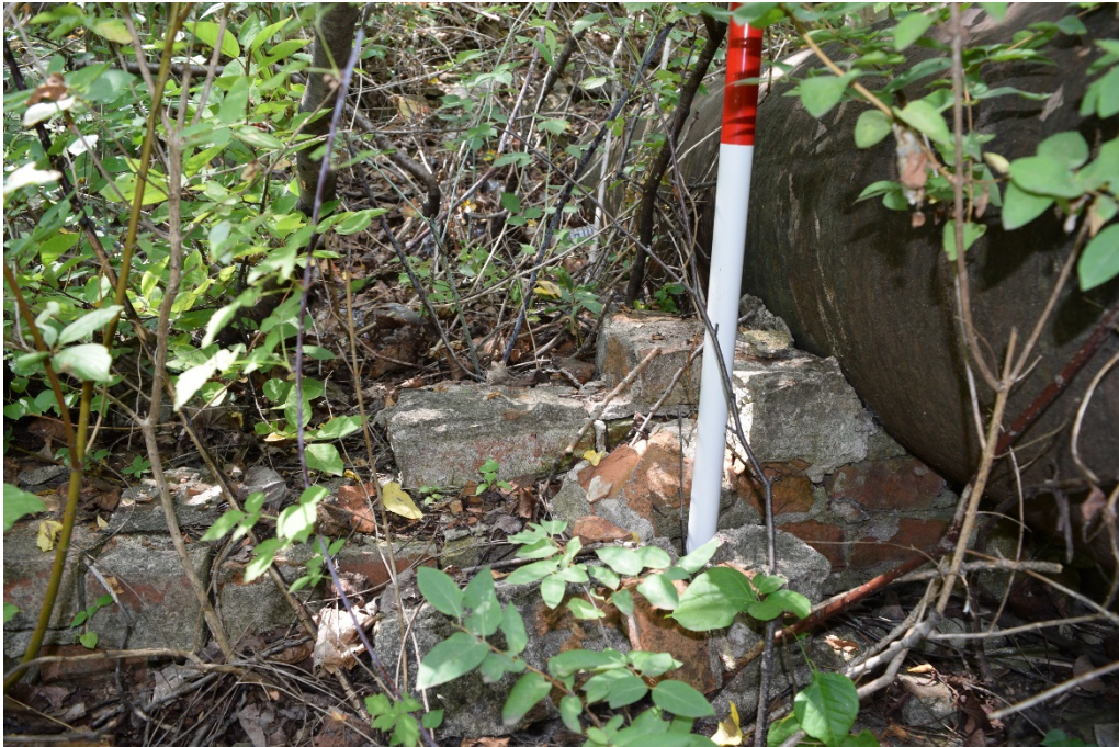
Figure 33: Brick base of the west main pipe.
