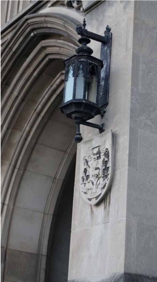
Fig. 33 Cast-iron lamp mounted on buttress framing portal, with carved crest below
