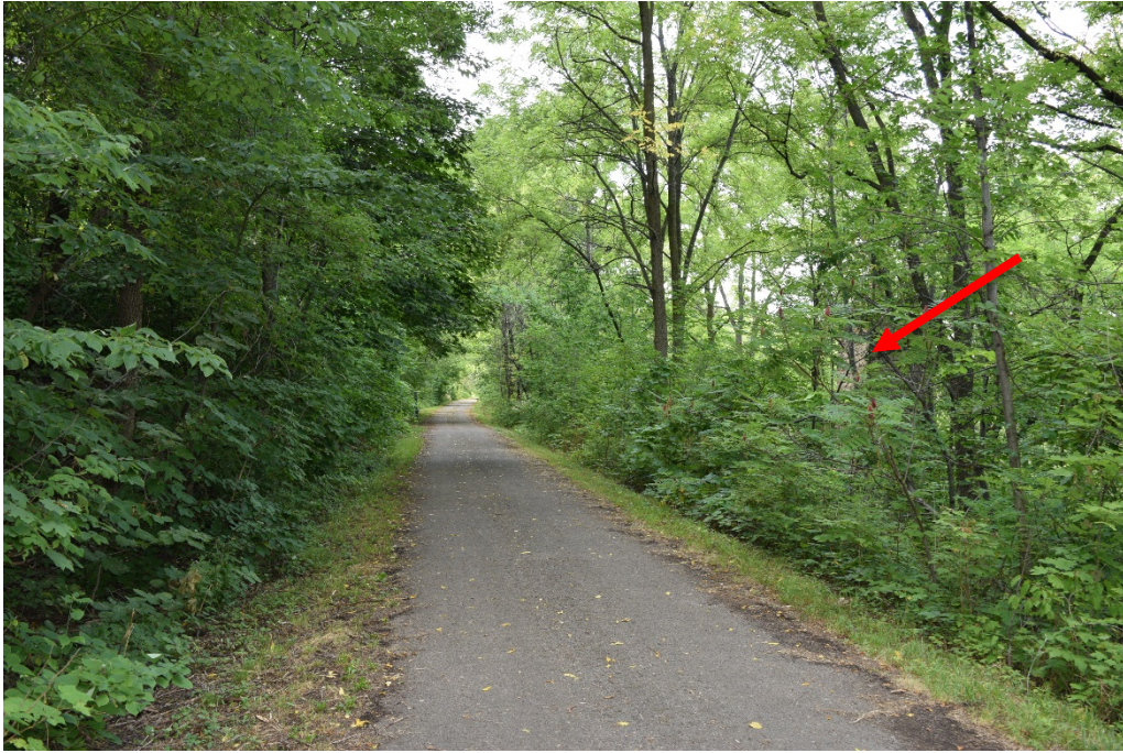
Figure 20: View facing west of the Escarpment Rail Trail. The masonry of the Standpipe is partially visible on the right of the trail (red arrow).
