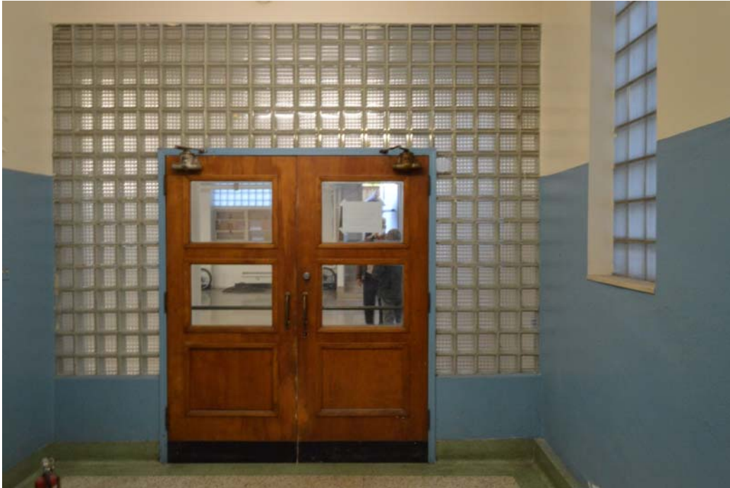
Fig. 149 Basement entrance at foot of stairs
