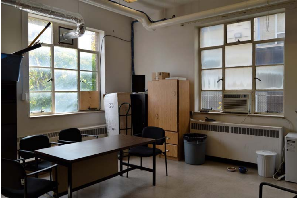
Fig. 137 Ground-floor room in wing's southeast corner, looking south. Note the operable steel sash windows with bronze hardware and travertine marble sills.
