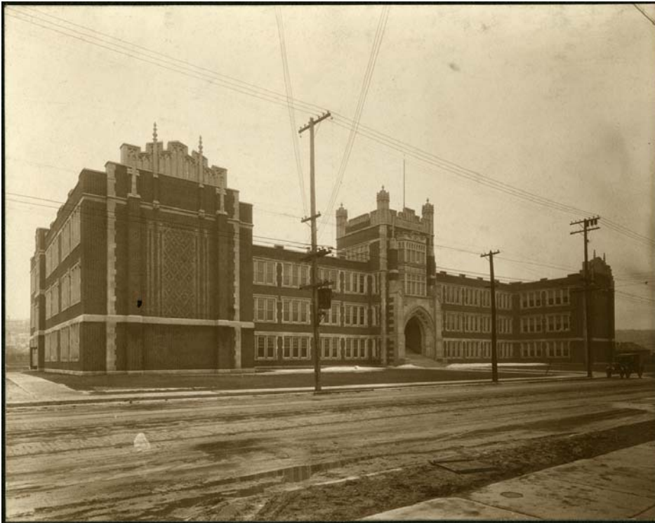
Fig. 25 Hutton & Souter, "Delta Collegiate," photograph of front facade, n.d., Archives of Ontario, C 12-2-0-1, Container B-868, Barcode B230391.
