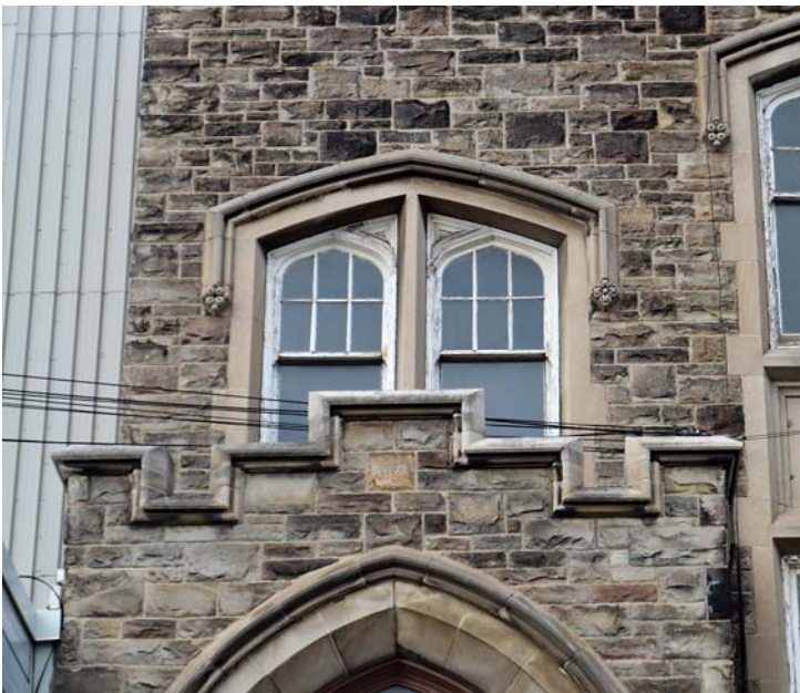
Fig. 56 Pair of windows in east entrance bay
