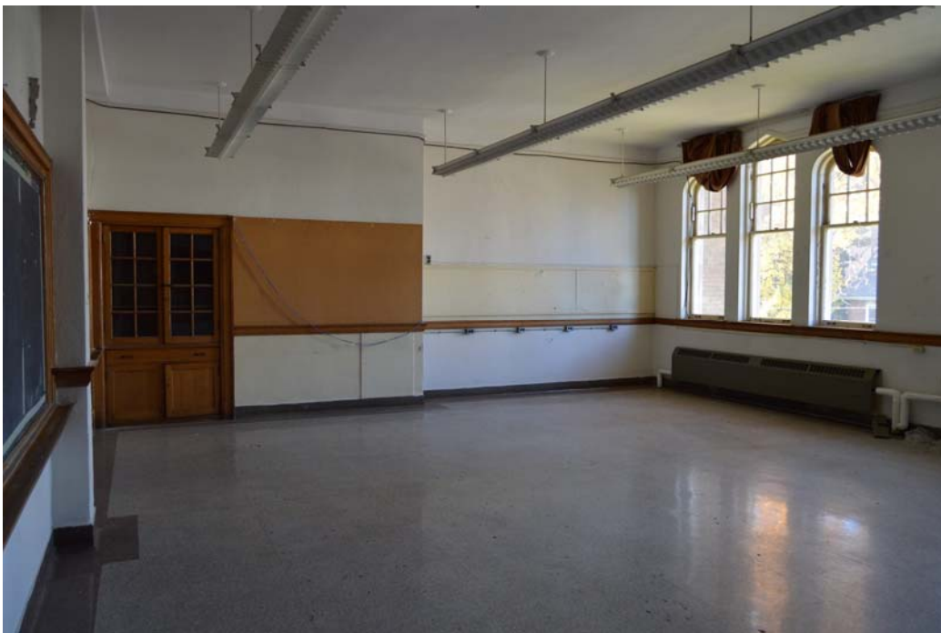
Fig. 116 Room 25 on south side of east-west corridor
