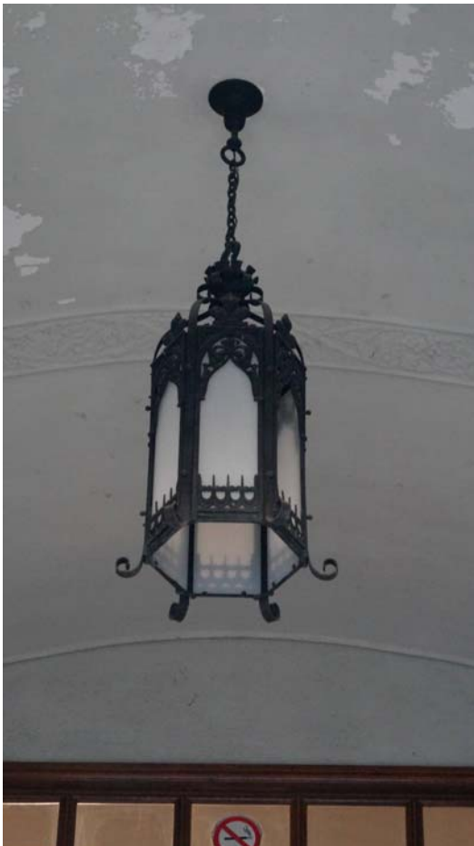
Fig. 38 Entry's porch lamp hanging from vaulted ceiling. Note how pointed arches have been incorporated into the cast-iron lamp.
