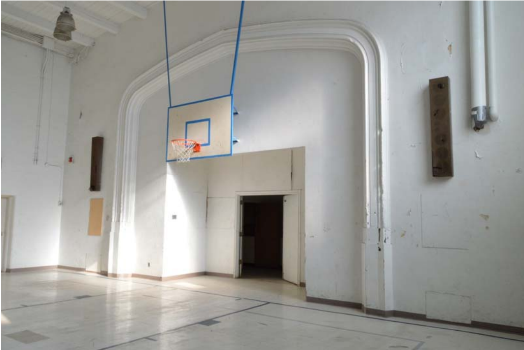
Fig. 125 Another view of the arch
