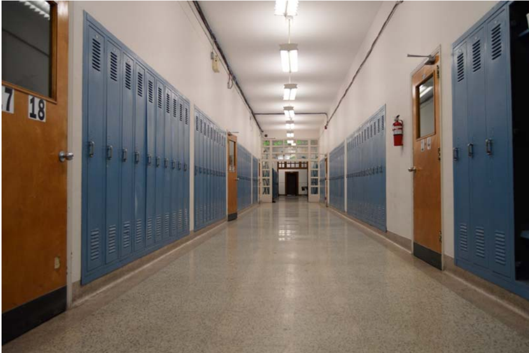
Fig. 139 Ground-floor north-south corridor, looking north. Note grey terrazzo floor with brownish terrazzo border and base and metal-and-glass frame of sidelights and transom light crossing the corridor.
