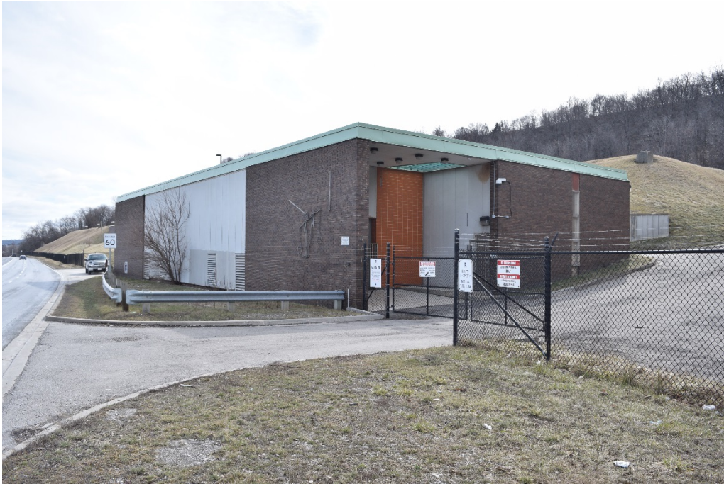
Figure 65: The pumphouse at the northwest corner of the reservoir.
