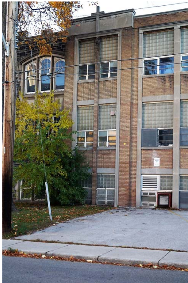
Fig. 70 Detail showing where stone-clad west facade meets wing's brick-clad west facade
