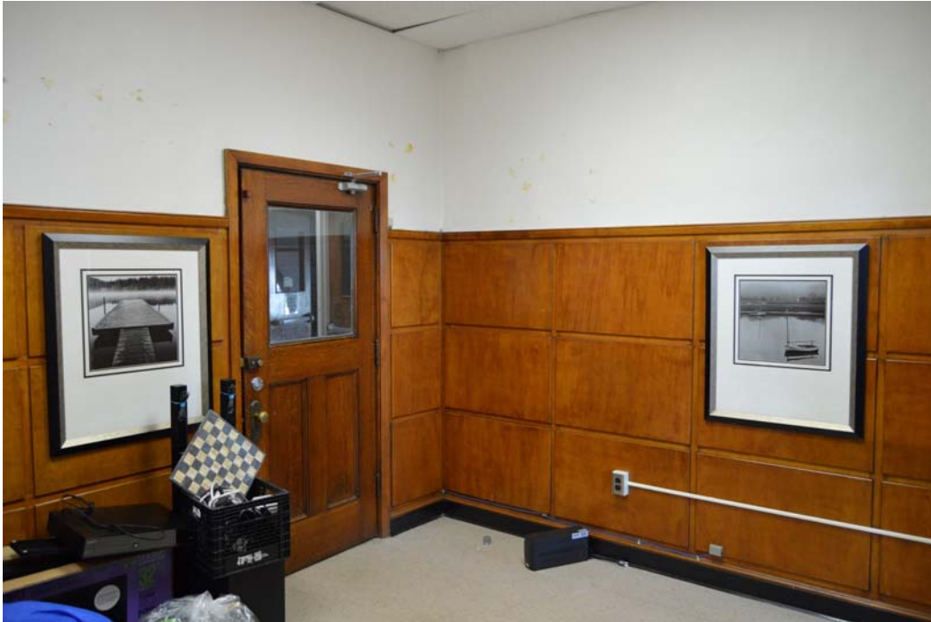
Fig. 82 Channelled plywood wainscoting in administration office
