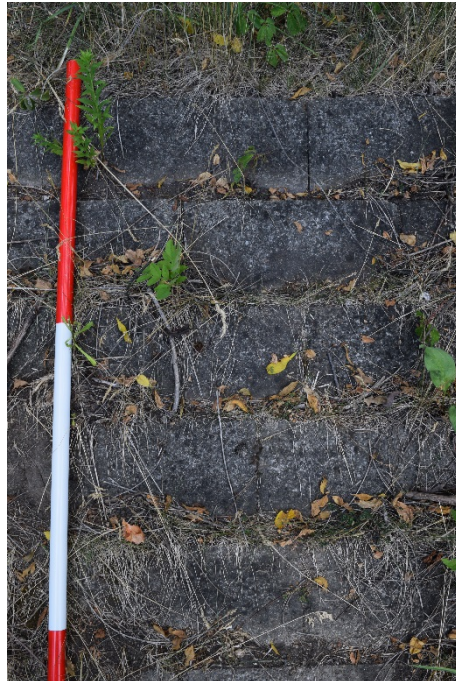
Figure 25: Detail of the ashlar clay block construction.
