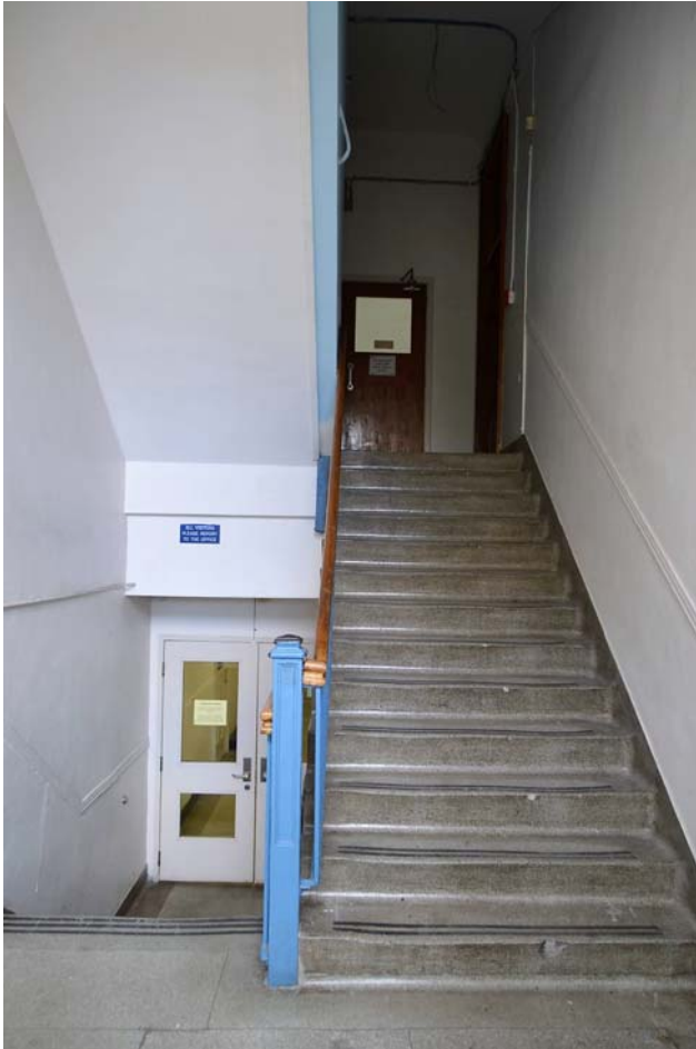
Fig. 77 West entrance staircase immediately past west entrance vestibule, looking up to the ground floor and down to the basement. Note the metal newel post, metal balusters, wood handrail and terrazzo risers and treads – all dating to the 1928 construction.
