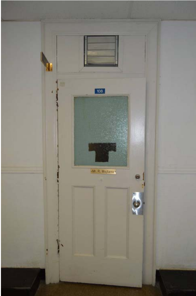
Fig. 119 Room 108 corridor door in basement
