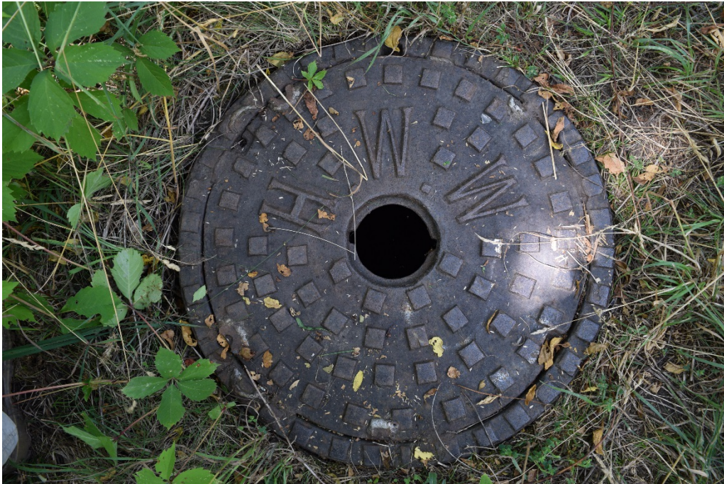
Figure 37: One of the manhole covers west of the reservoir.
