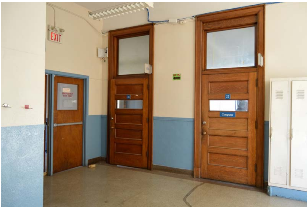
Fig. 96 Plain terrazzo floor (grey field with darker border) and oak doorways on upper floor
