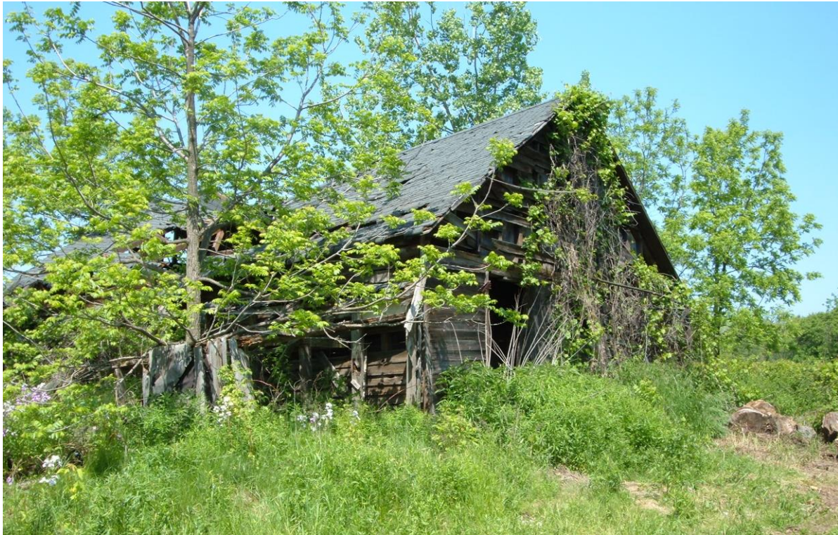
Image 5: View of one of the property's crumbling outbuildings in 2010 (Wray, 2010).
