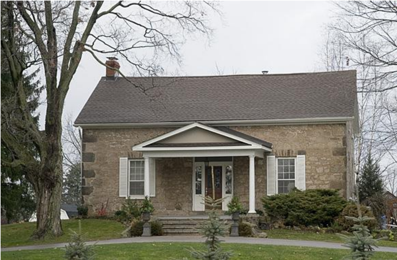
Figure 3: A closer image of the subject property. Note the location of the westerly chimney (the easterly chimney was removed sometime after 1982). The prominent, pedimented modern portico was modeled after a previous portico which was replaced sometime after 1982 (Paul Dolanjski, 2009).
