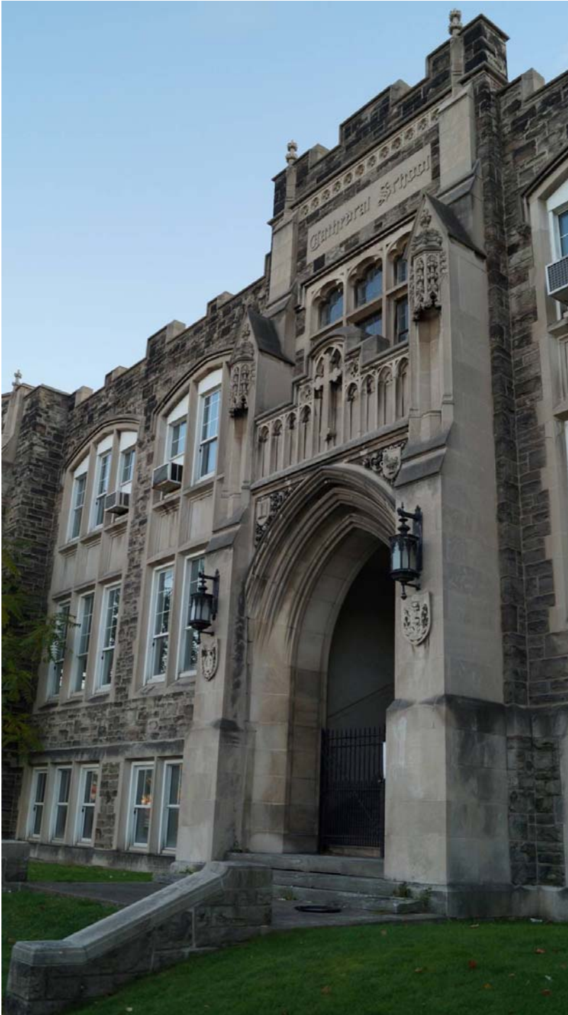
Fig. 27 Another view of entrance bay
