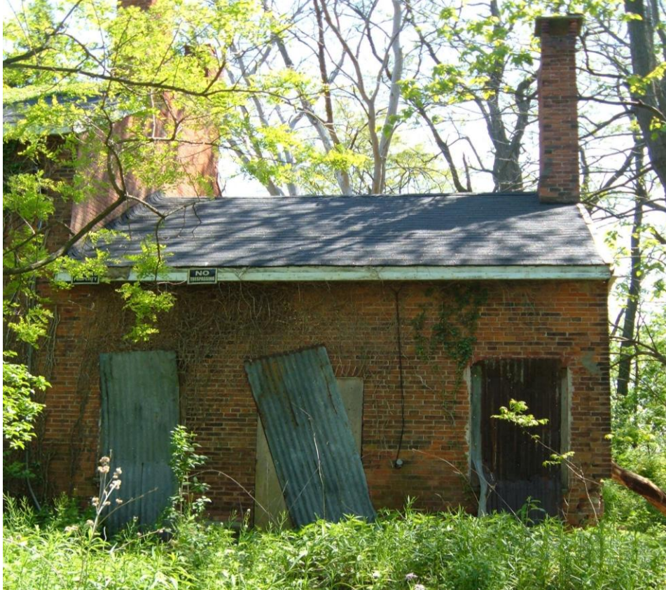
Image 7: The property contains an early or original one-storey brick wing, likely built as a kitchen, with a large chimney (Wray, 2010).
