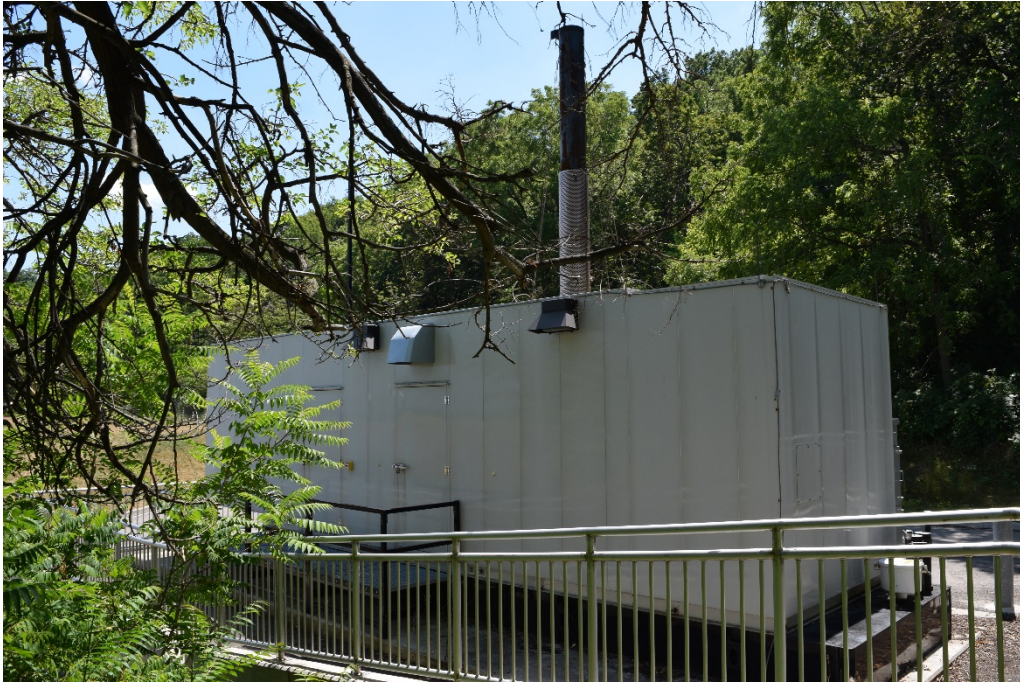
Figure 64: The electrical building near the southwest corner of the reservoir.
