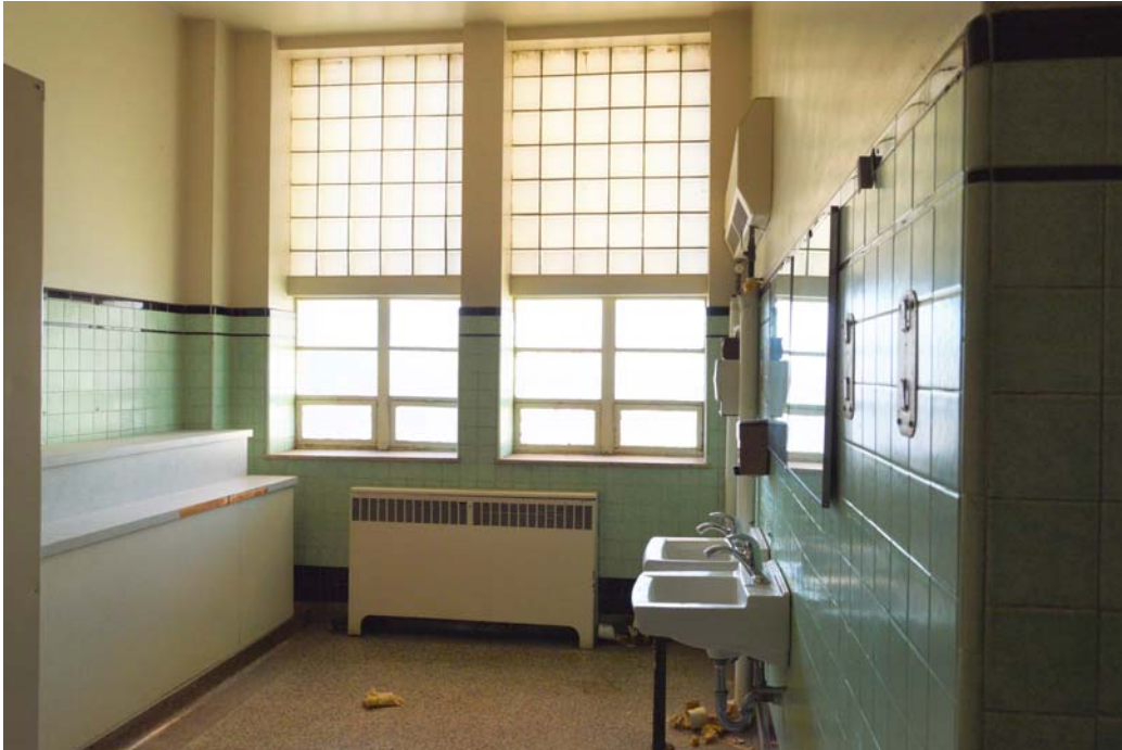
Fig. 147 Upper-floor washroom. Note the green-and-black tiled wainscoting and the window pair with glass block uppers and clear glass lowers.
