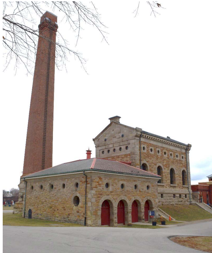
Figure 5: Left to right: the Chimney, Boiler House, and Engine House of the Hamilton Waterworks NHSC, February 2017.
