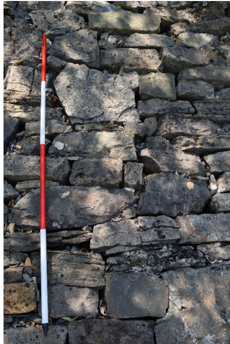
Figure 27: Detail of the coursed rubble construction.
