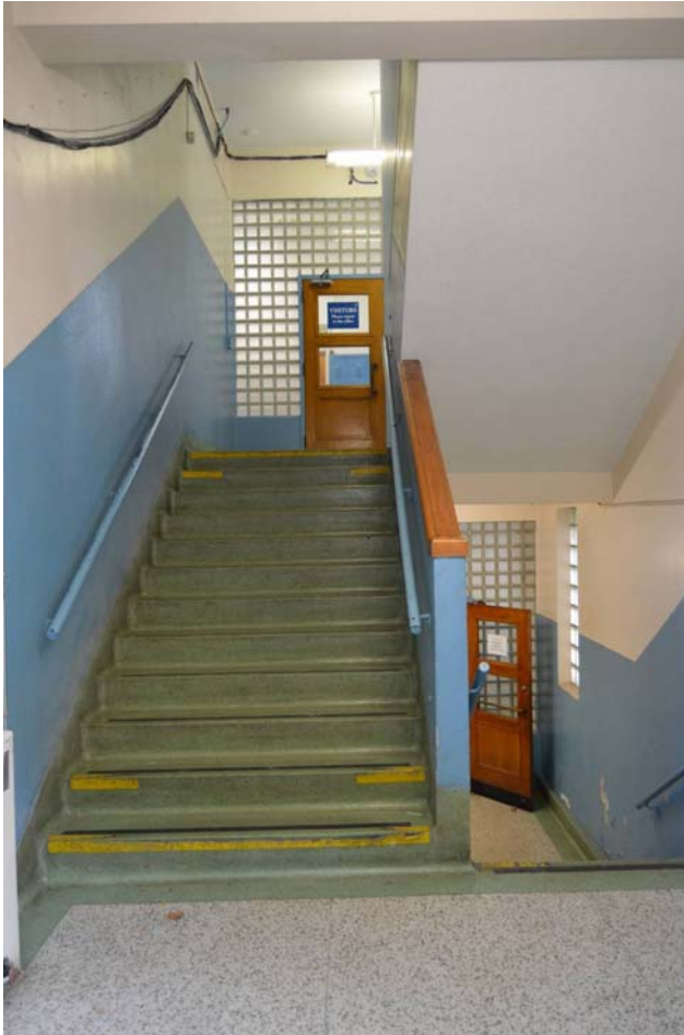
Fig. 131 Stairwell inside entry to wing, looking up to the ground floor and down to the basement
