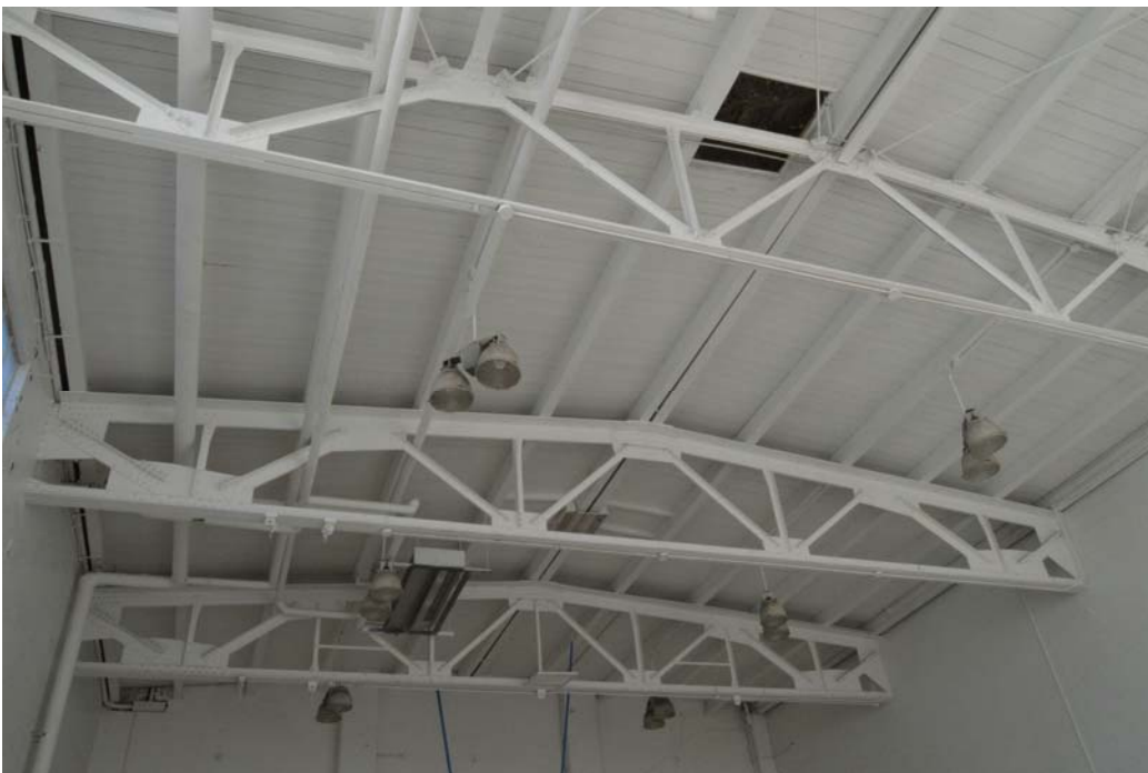
Fig. 128 Gymnasium ceiling trusses
