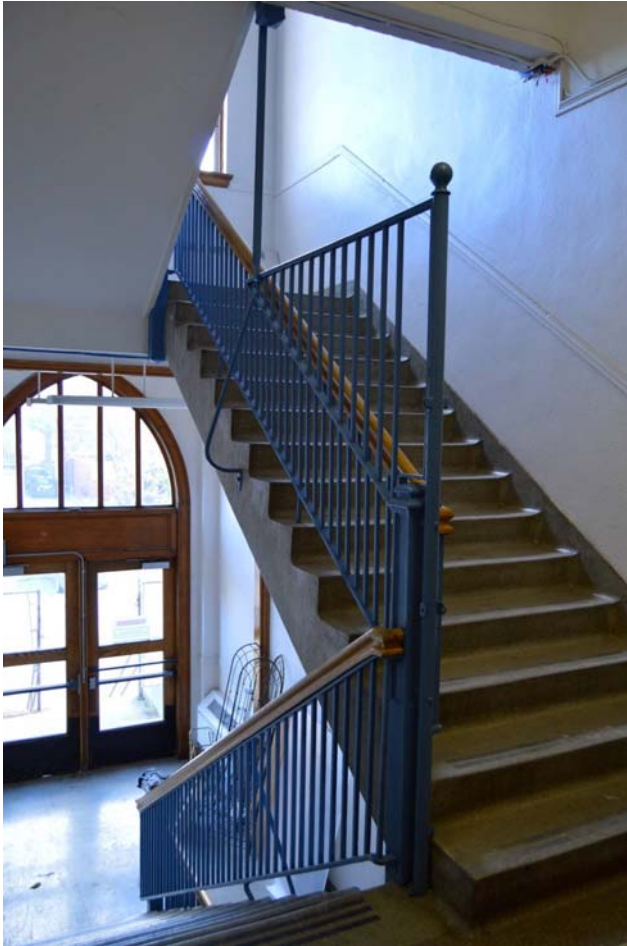
Fig. 91 East entrance stairwell and staircase
