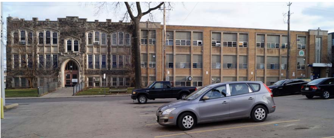
Fig. 64 West facades of 1928 building and 1951 wing facing Emerald Street South
