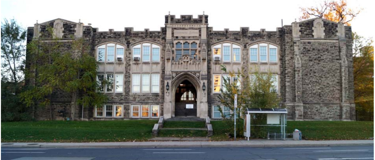
Fig. 21 Front facade of 1928 building as seen from north side of Main Street East
