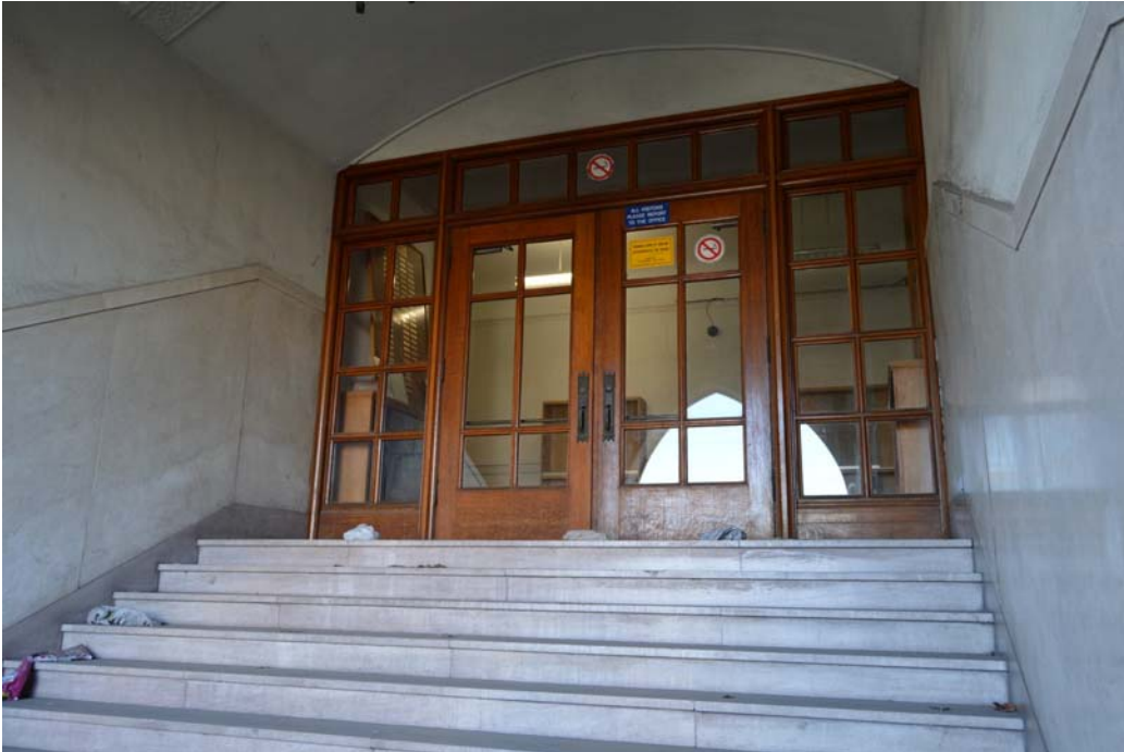
Fig. 35 View as seen inside the entry porch, looking up the marble staircase to the doorway into the school's front vestibule
