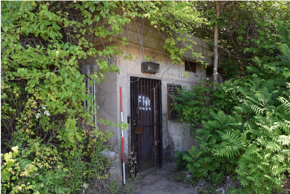
Figure 63: Concrete structure at the southwest corner of the reservoir.
