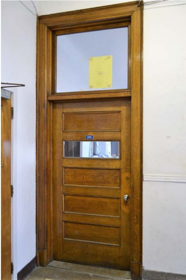
Fig. 89 Doorway to Room 215
