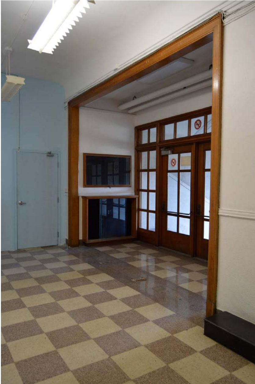
Fig. 86 Front entrance vestibule with fire separation partition on left of frame. Note holes in floor where the vestibule doors once stood.
