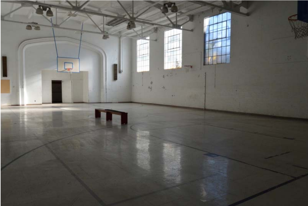
Fig. 123 Gymnasium, looking east toward altered stage. Note the industrial window sash.
