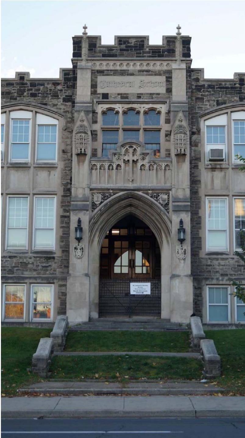
Fig. 26 Front entrance bay
