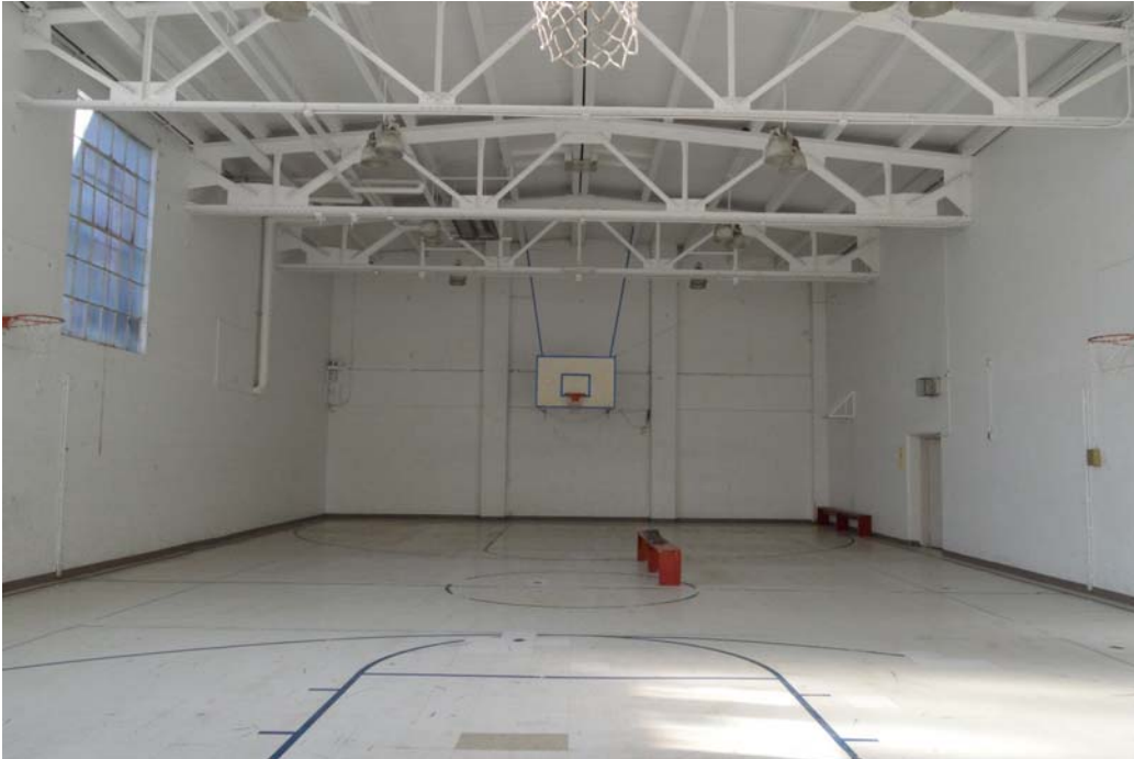
Fig. 127 Gymnasium, looking west. Note ceiling trusses.
