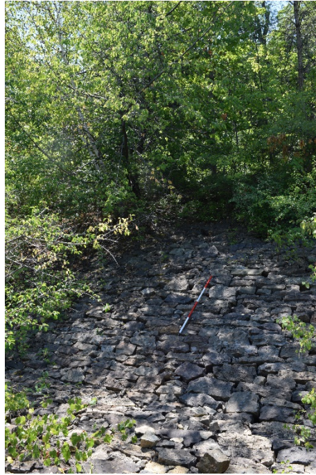
Figure 26: View facing south of the coursed rubble construction.
