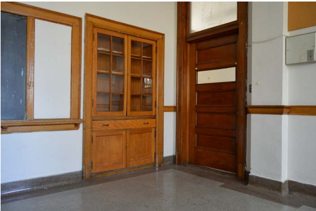
Fig. 102 Room 26 blackboard/tack board, built-in cabinet, door and chair rail
