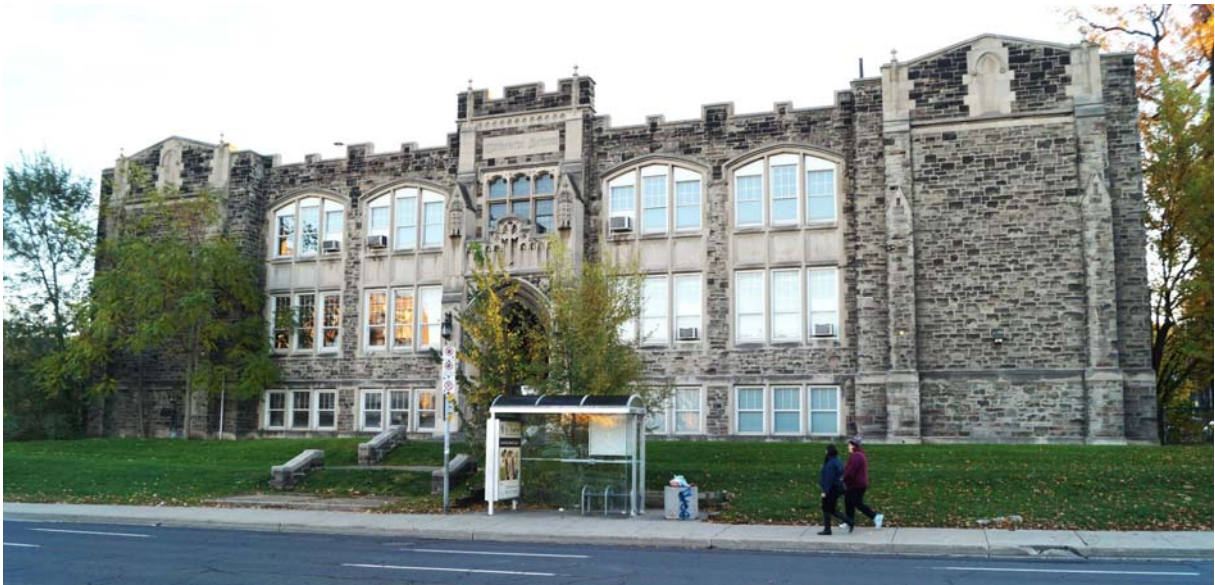
Fig. 22 Another view of front facade
