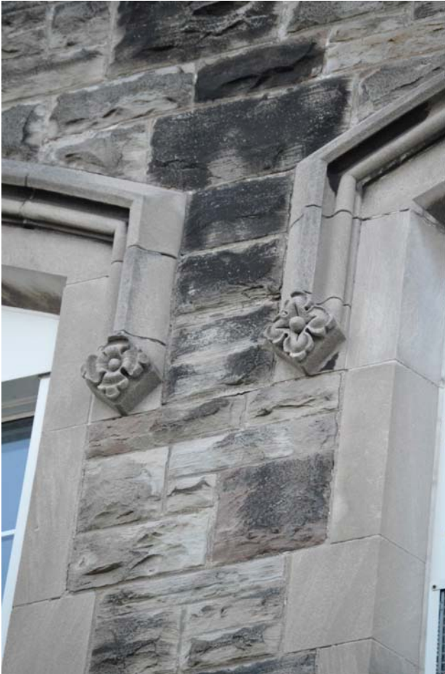
Fig. 46 A variety of bosses at the end of hood-moulds over the uppermost windows. Note the boss in the shape of a Tudor rose on the left.
