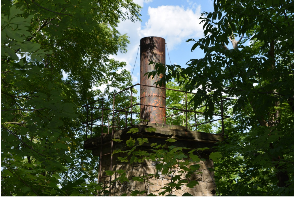
Figure 45: The platform and riveted casing of the second stage, facing north.
