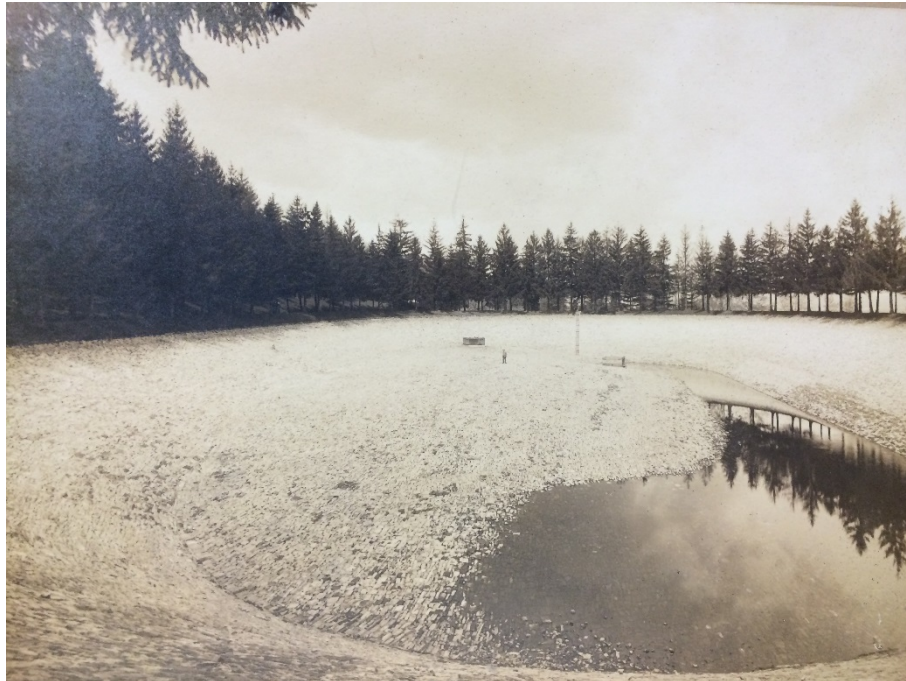
Figure 23: Circa 1912 view of the reservoir, facing west (courtesy HMST).
