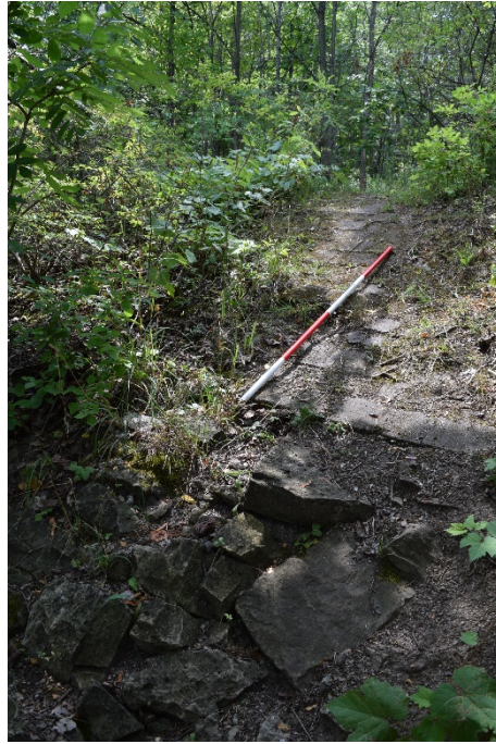
Figure 24: View facing south of the clay block section around the top of the south portion of the reservoir.
