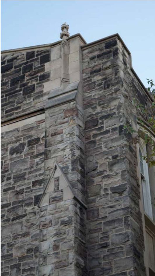
Fig. 49 Gablet on buttress and cap of buttress
