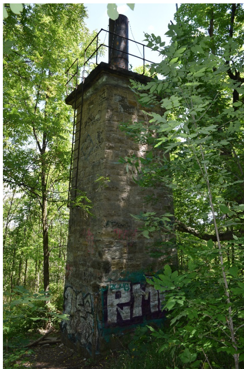
Figure 40: The west and south sides of the Standpipe.
