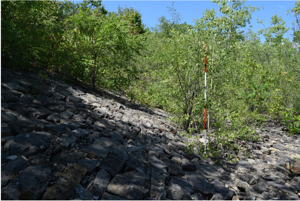
Figure 22: View facing west showing the gradual slope on the south side of the reservoir.
