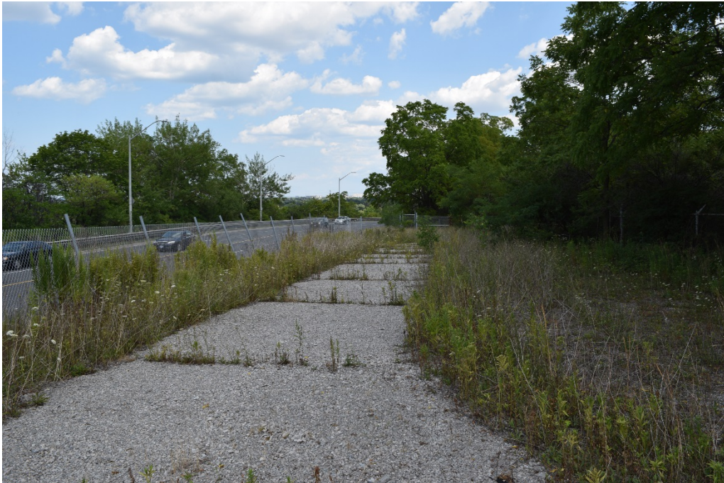
Figure 19: View facing east of the disused driveway on the west side of the property.
