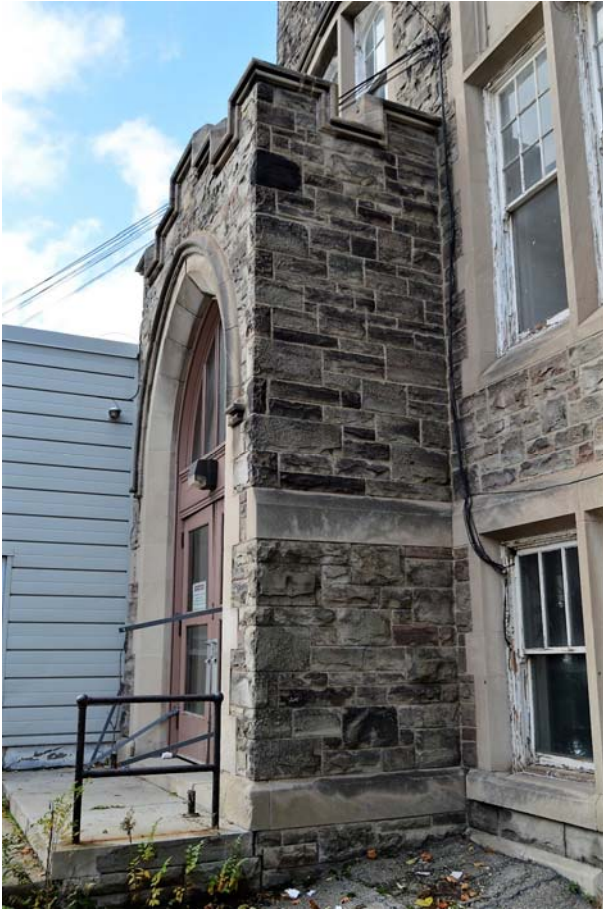
Fig. 55 East entrance vestibule, showing how it projects from the east facade
