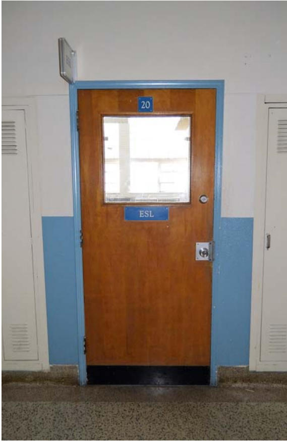
Fig. 145 Typical door to upper-floor classroom
