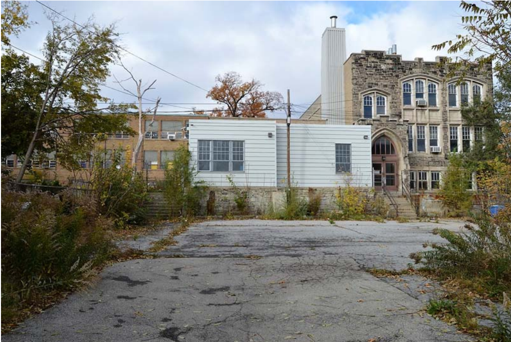
Fig. 51 Eastern view of school, showing from left to right: brick-clad wing from 1951, one-storey frame addition, re-clad chimney stack and three bays in the 1928 building
