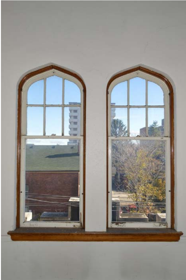
Fig. 93 East stairwell windows with original oak ledge and wood sash
