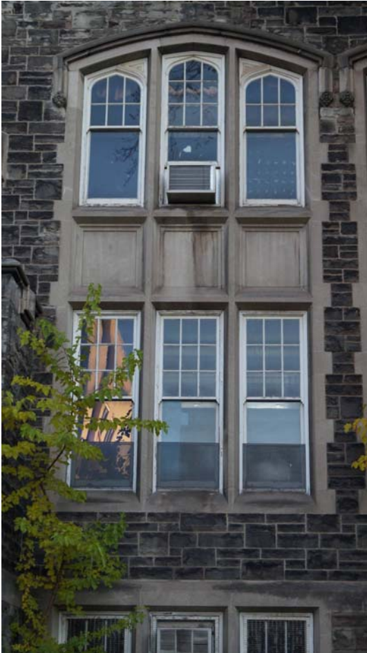
Fig. 69 Upper-floor windows in west facade
