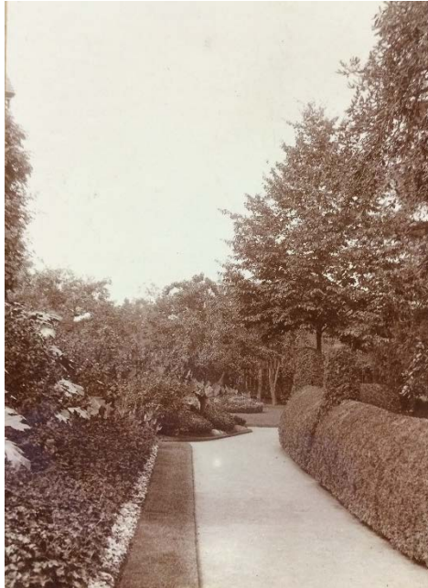
Figure 53: Circa 1912 photograph of the gardens at Reservoir Park (courtesy HMST).
