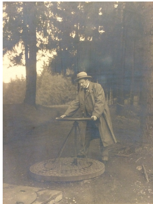
Figure 39: Circa 1912 photograph of Adam Brown turning one of the valves over a manhole cover west of the reservoir (courtesy HMST).
