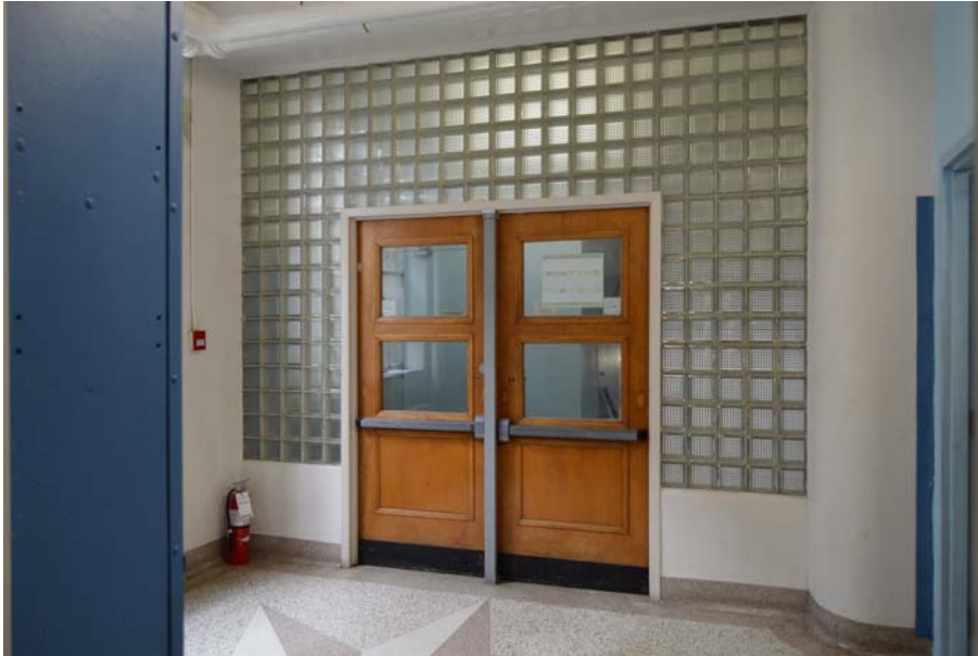
Fig. 133 Ground-floor lobby, looking west to entrance wall. Note patterning of grey and brownish terrazzo for the lobby's floor.
