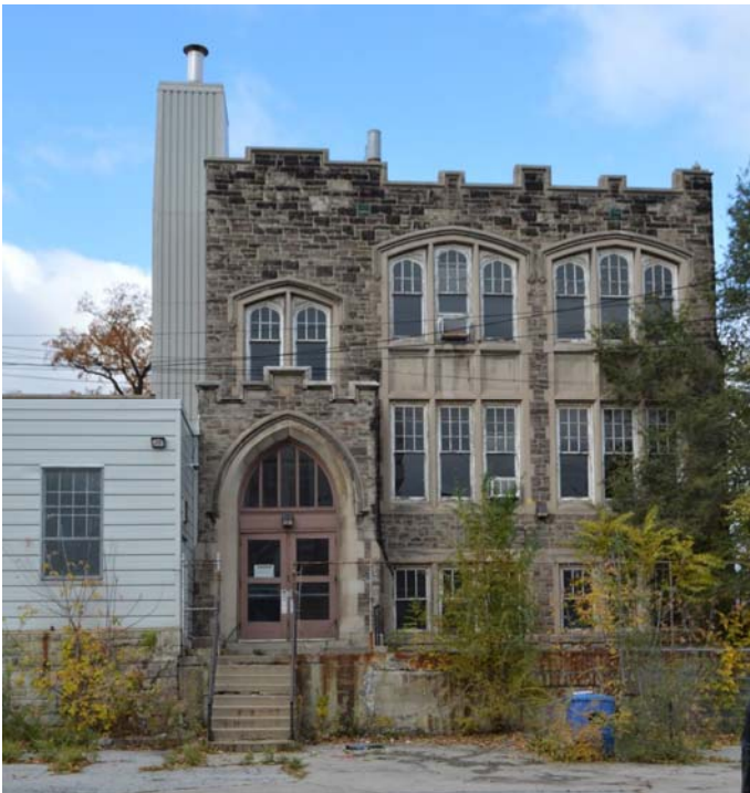
Fig. 52 East facade of 1928 building
