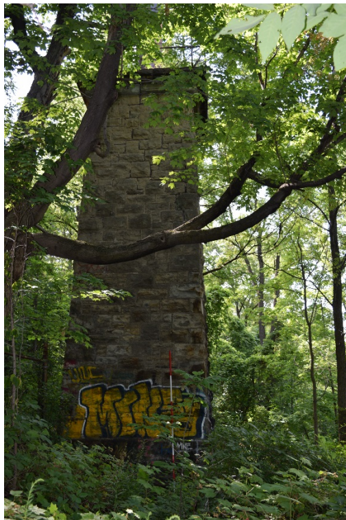
Figure 42: East side of the Standpipe.
