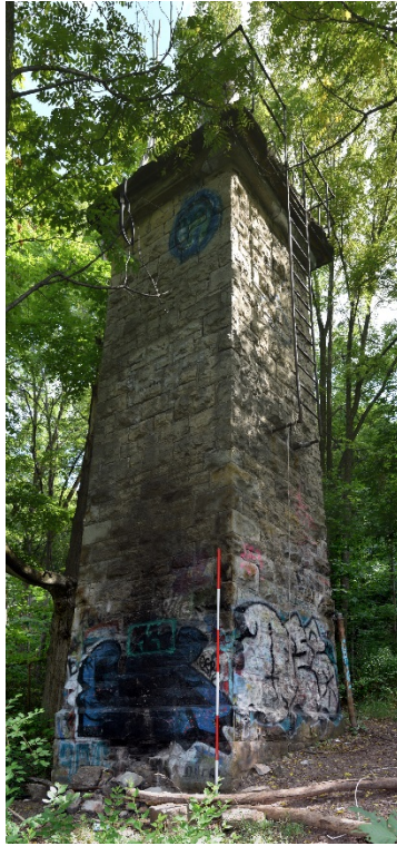
Figure 41: North and west sides of the Standpipe.
