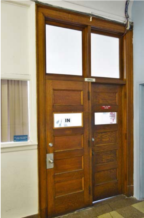
Fig. 84 Doorway to room adjoining administration office
