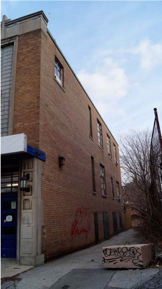
Fig. 75 South or rear elevation of 1951 wing. Note how the front doorway's stone embrasure wraps around the corner to the south elevation and how the stone cornice also does the same.
