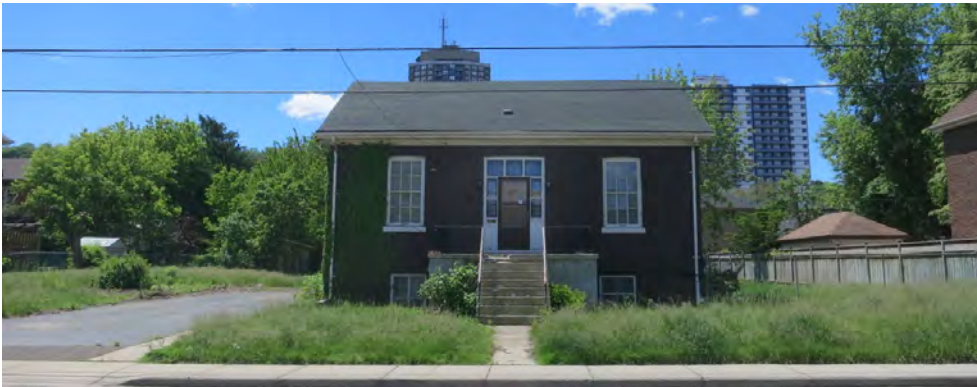
122 & 126 Augusta Street – the subject property has a large frontage on the south side of Augusta Street comprised of a vacant lot and a 1.5 storey brick dwelling constructed in the 1860s
