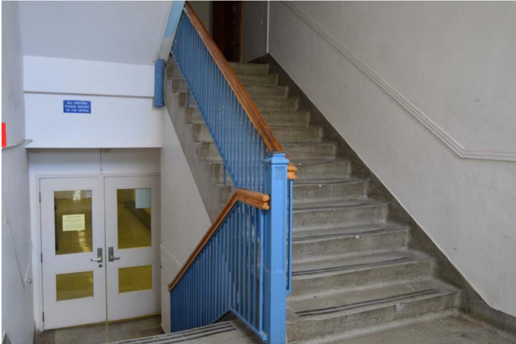
Fig. 78 Another view of the west entrance staircase
