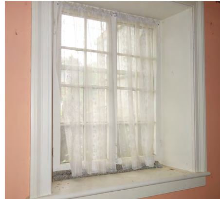
Basement – 8-pane double-casement windows
