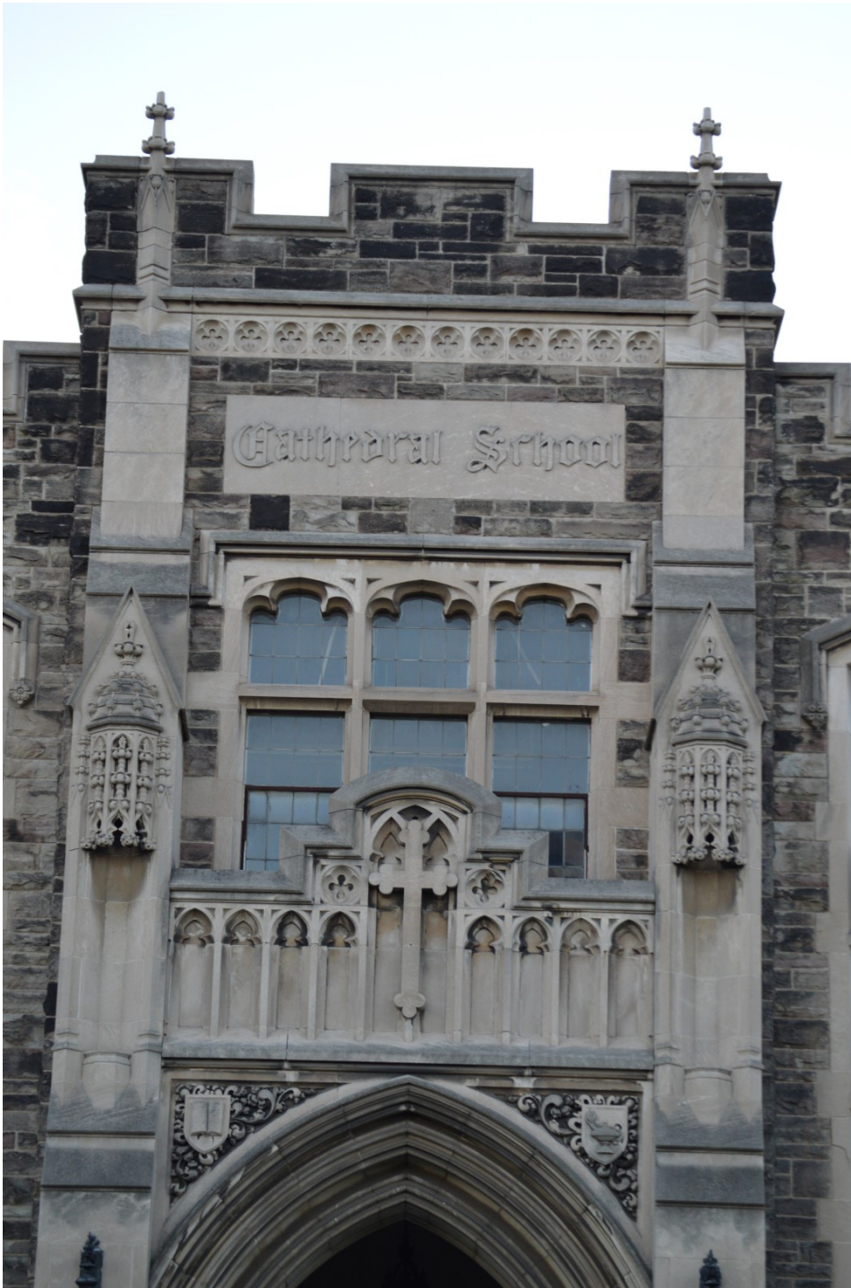
Fig. 40 Front entrance bay above portal
