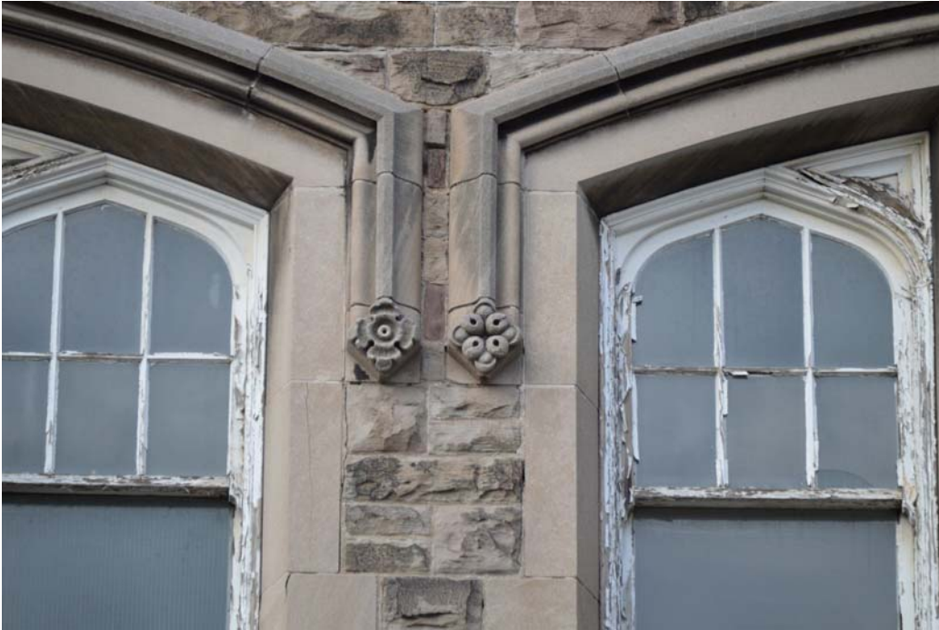
Fig. 59 Detail from upper-floor windows, showing hood-moulds that terminate in either a Tudor rose in full bloom or a rose in bud
