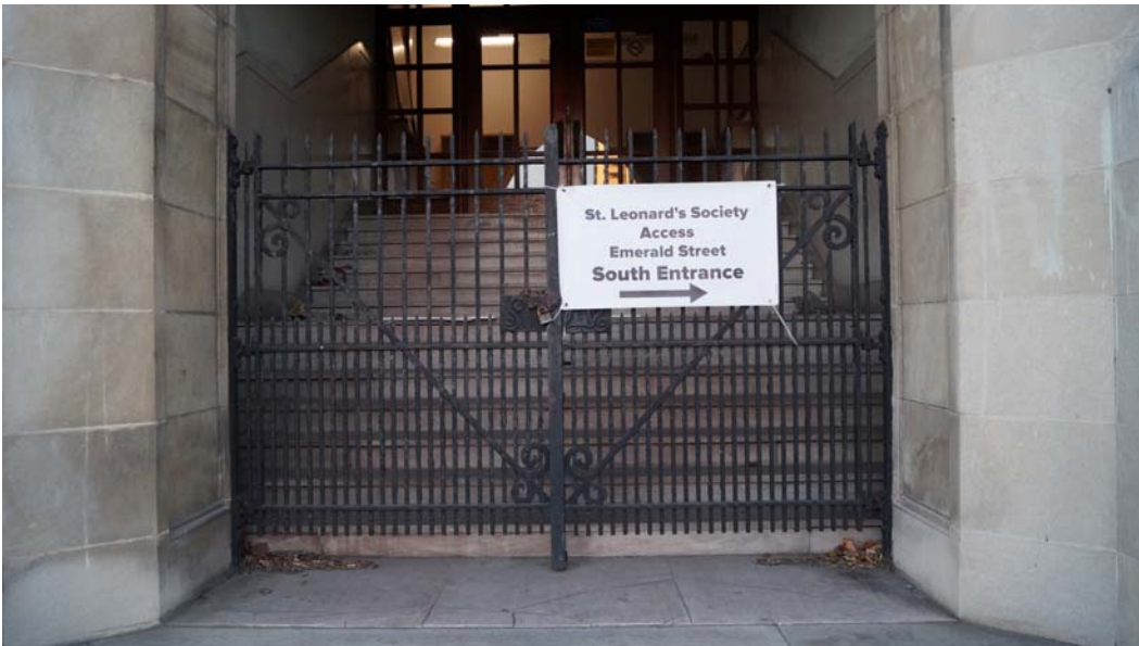
Fig. 32 Wrought-iron gate across portal
