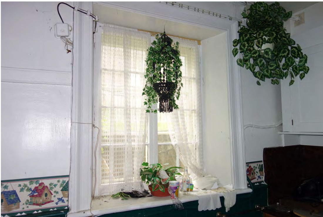
Kitchen – wood casement window
