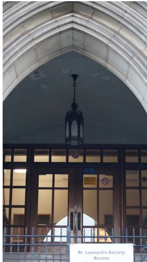
Fig. 30 Close-up view of portal, looking inside entry porch
