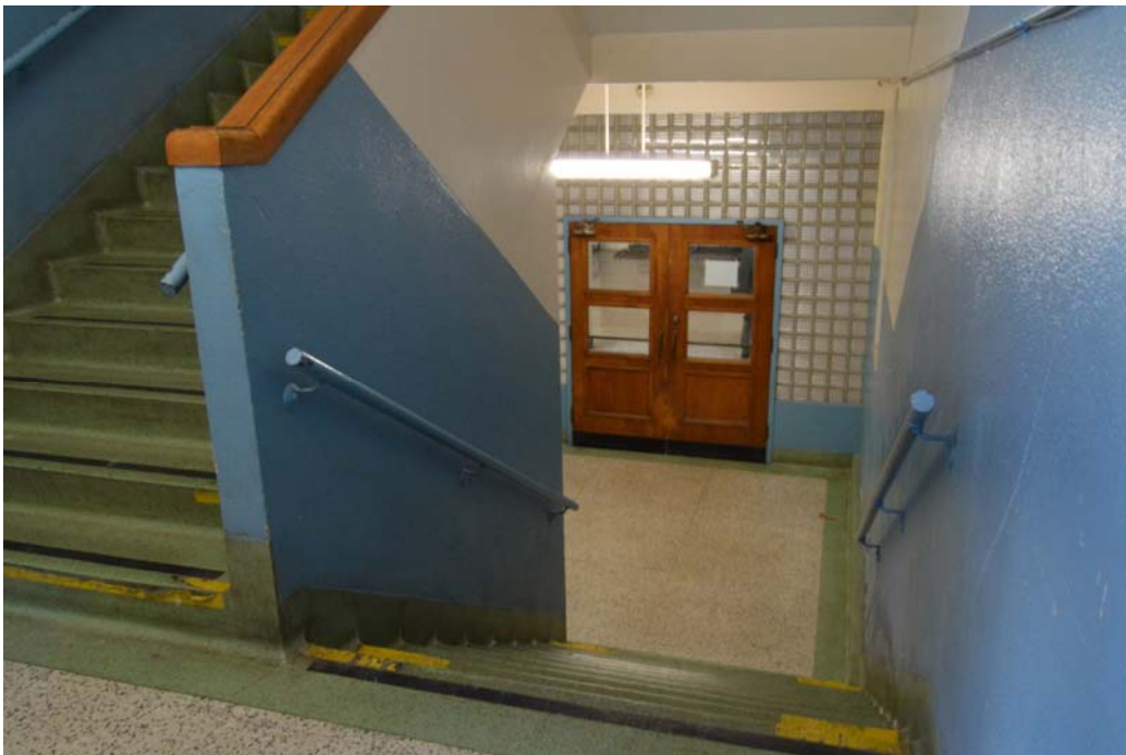
Fig. 148 Staircase down to basement
