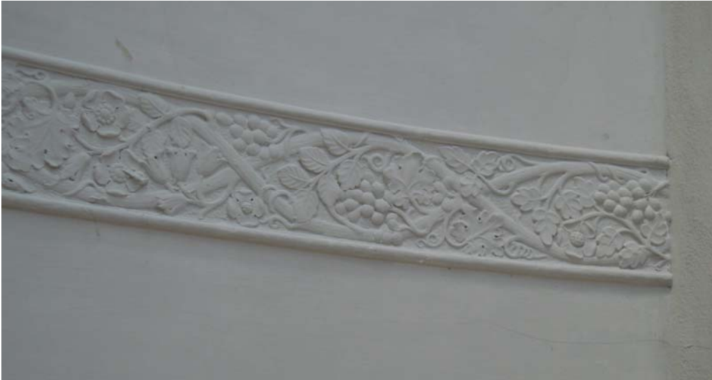
Fig. 37 Entry porch's plaster ceiling relief in a pattern of grape vines and Tudor roses
