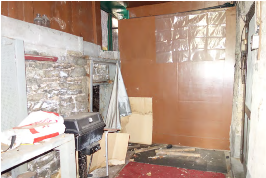
Porch - west end
