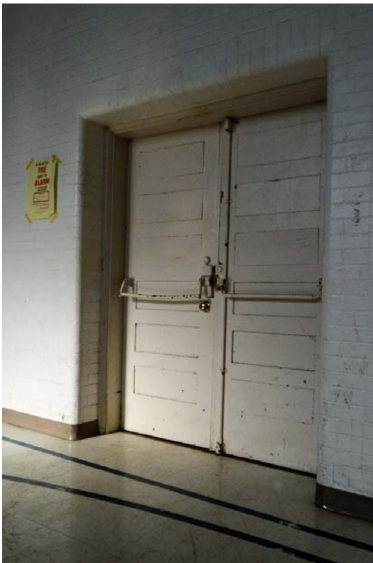
Fig. 122 Inside gymnasium doors. Note how the double doors are deep set.
