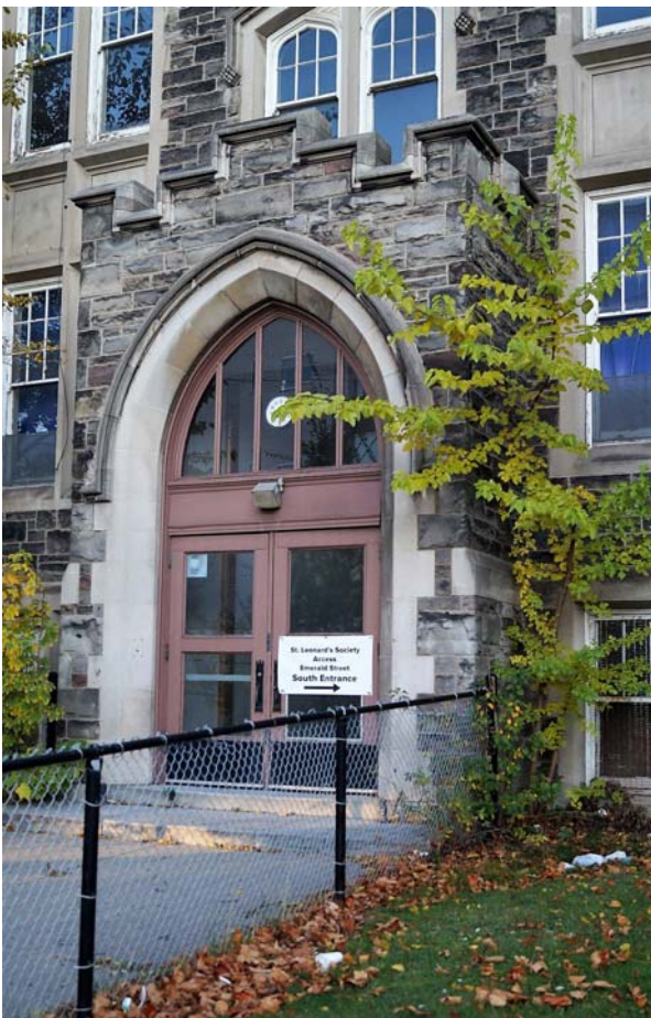
Fig. 66 West entrance vestibule
