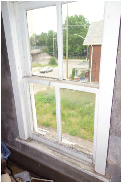
Window - 2 over 2 sash
