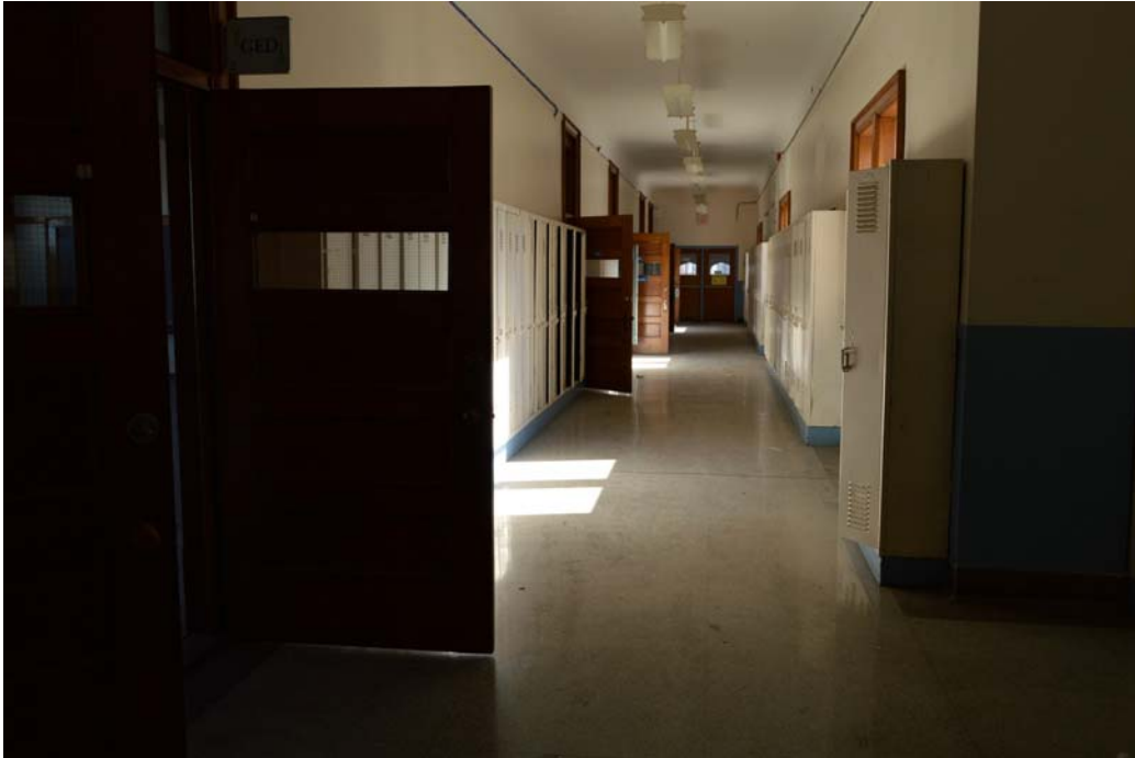
Fig. 95 East-west corridor on upper floor, looking east. Note south wall of corridor (on the right of the frame) is directly beside the external south wall.
