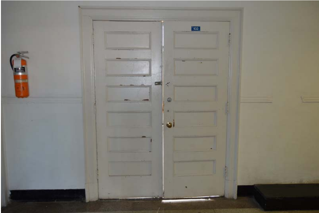
Fig. 121 Room 102 (gymnasium) corridor doors
