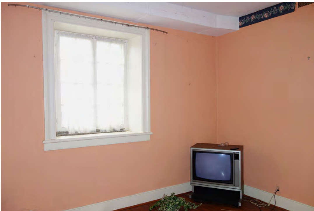
Bedroom 1 – modern drywall ceiling and modern hardwood flooring
