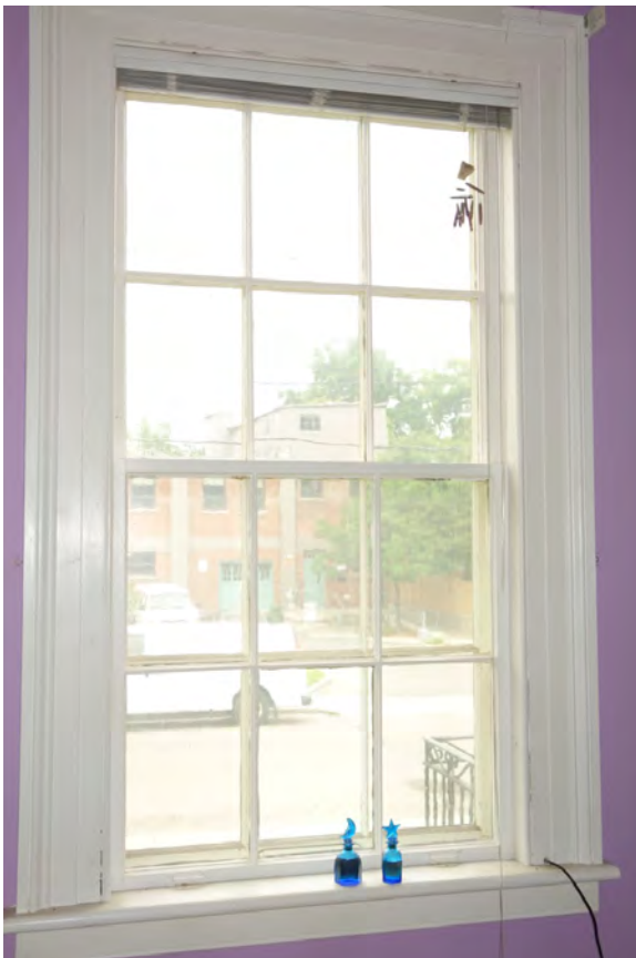
West parlour – 6 over 6 wood sash window
