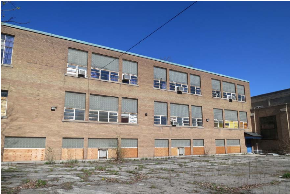
Fig. 62 East or rear elevation of 1951 wing
