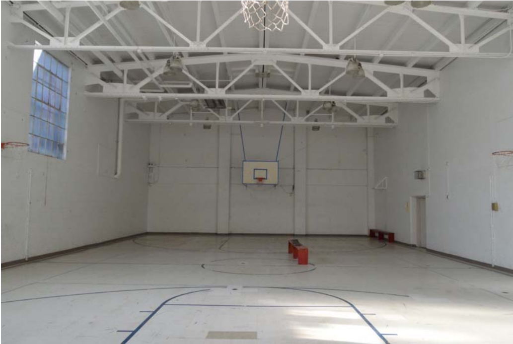
Fig. 127 Gymnasium, looking west. Note ceiling trusses.
