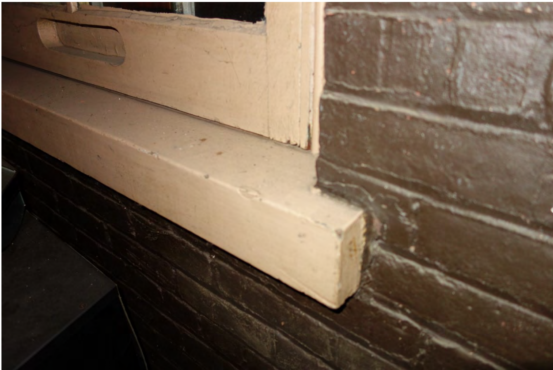
Exterior brick wall - wood window sill
