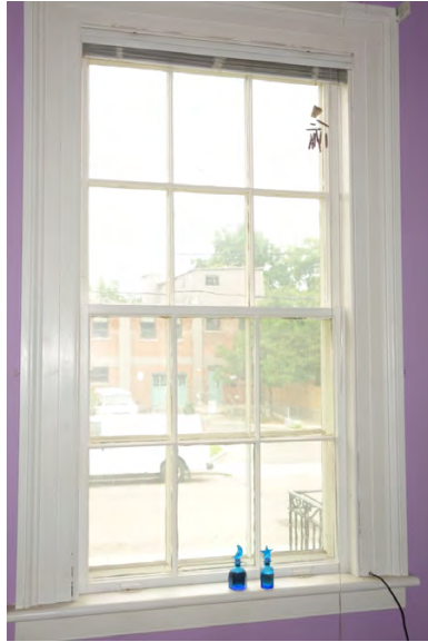
Main floor - 6 over 6 sash windows
