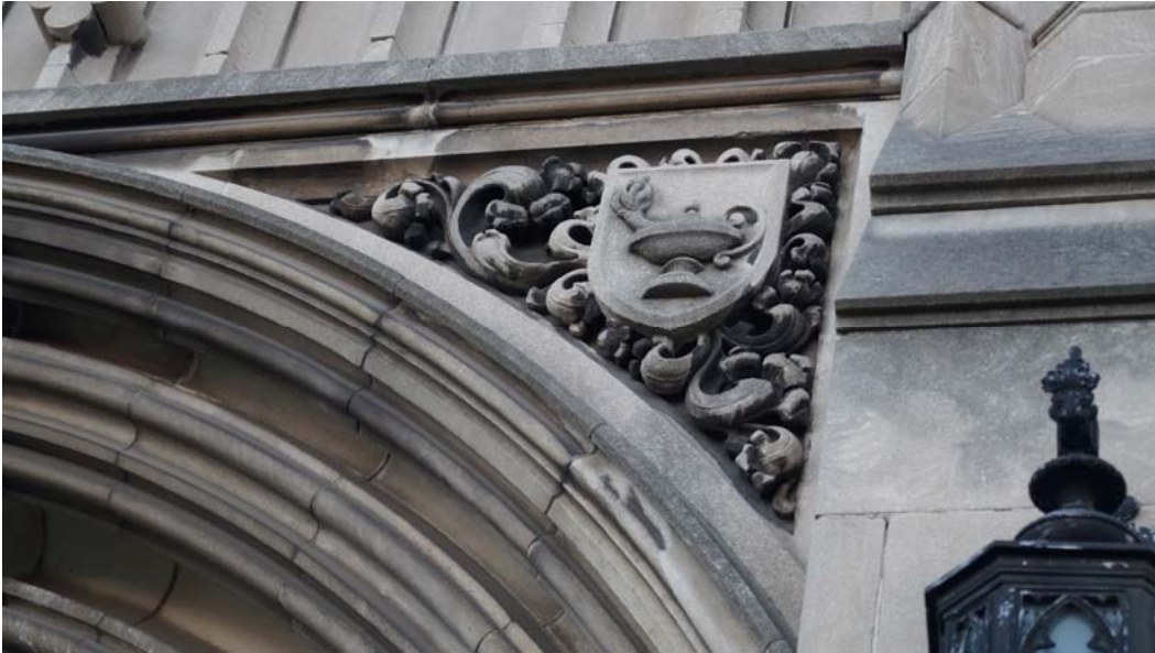
Fig. 31 Triangular stone panel (spandrel) shouldering portal's pointed arch and carved with the "lamp of learning" and foliage
