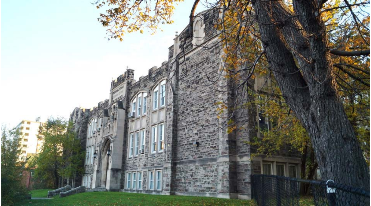
Fig. 23 Front facade as seen from Emerald Street South
