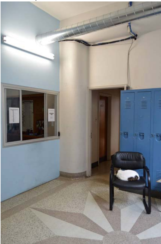
Fig. 136 Ground-floor lobby, looking east. Note rounded northeast corner and how the terrazzo border and baseboard curve around it. An alteration to the original layout, the blue wall on the north side of the lobby is a partition used to enclose a control room for the former school's present use as a halfway house for prisoners entering back into society. The door opening leads to a room in the wing's southeast corner.
