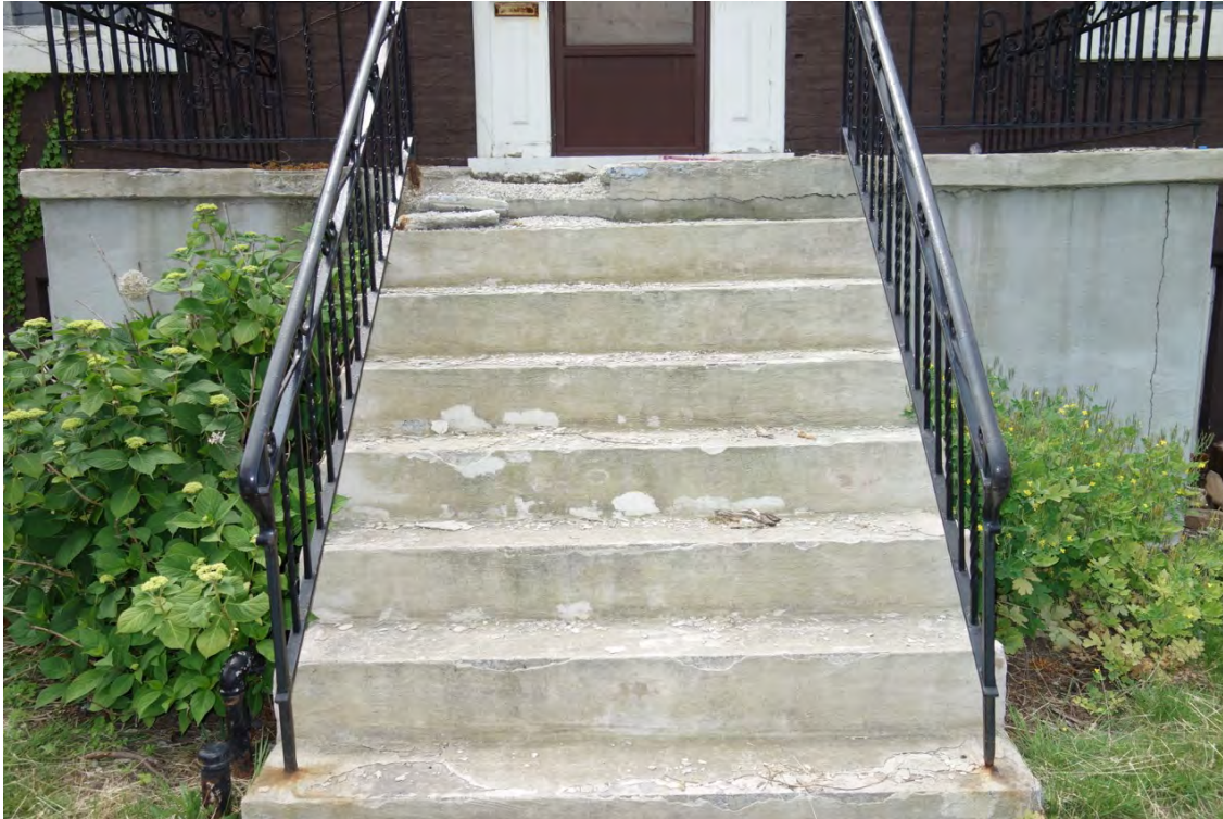
Modern concrete stoop and wrought iron railings
