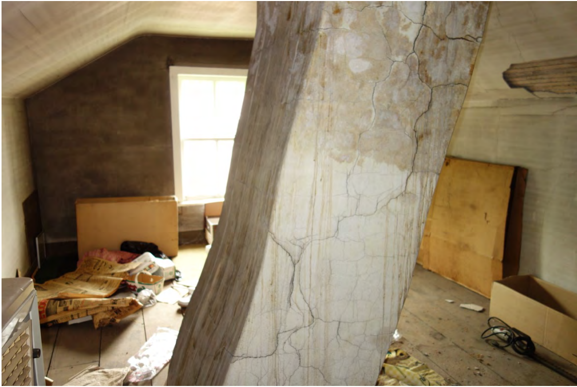
Freestanding chimney stack
