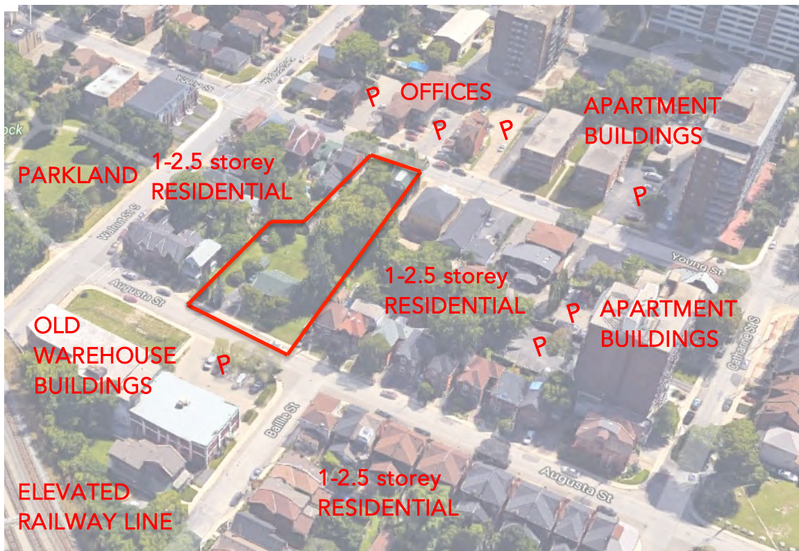
Aerial view of the subject property; 122-126 Augusta Street & 125-127 Young Street
