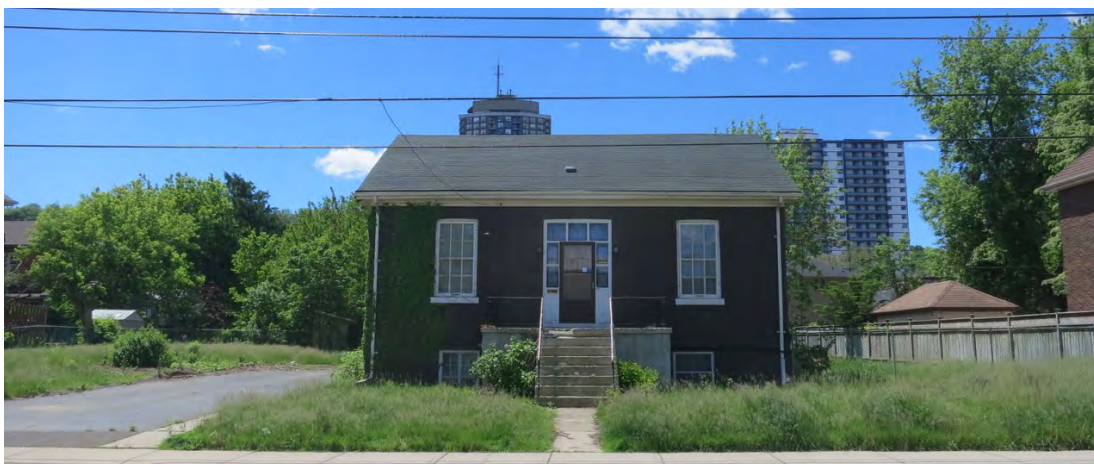
122 Augusta Street – the applicant proposes to demolish this dwelling
