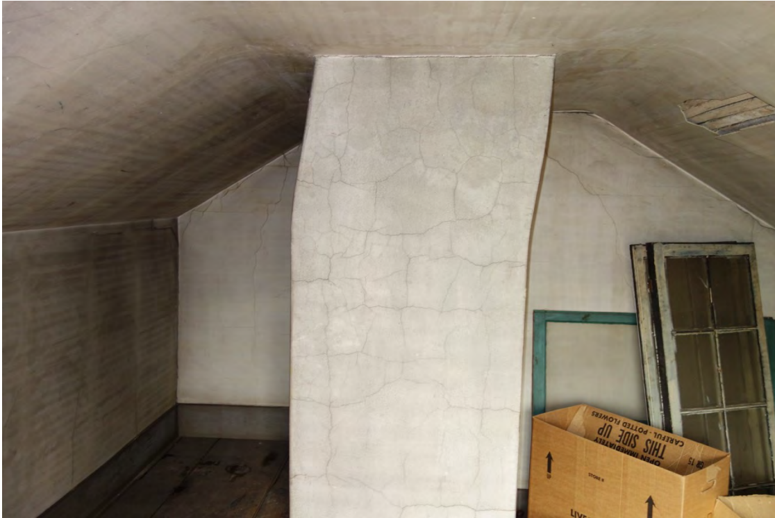
Free-standing chimney stack
