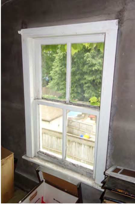
Window - 2 over 2 wood sash
