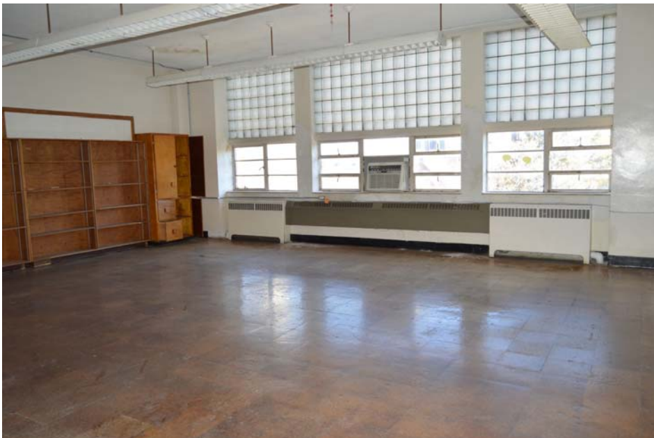
Fig. 146 Typical upper-floor classroom. Note cork floor and tripartite window with fixed glass block uppers and operable clear glass lowers.
