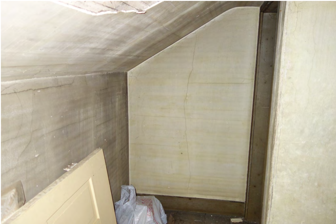
Attic hallway – east end
