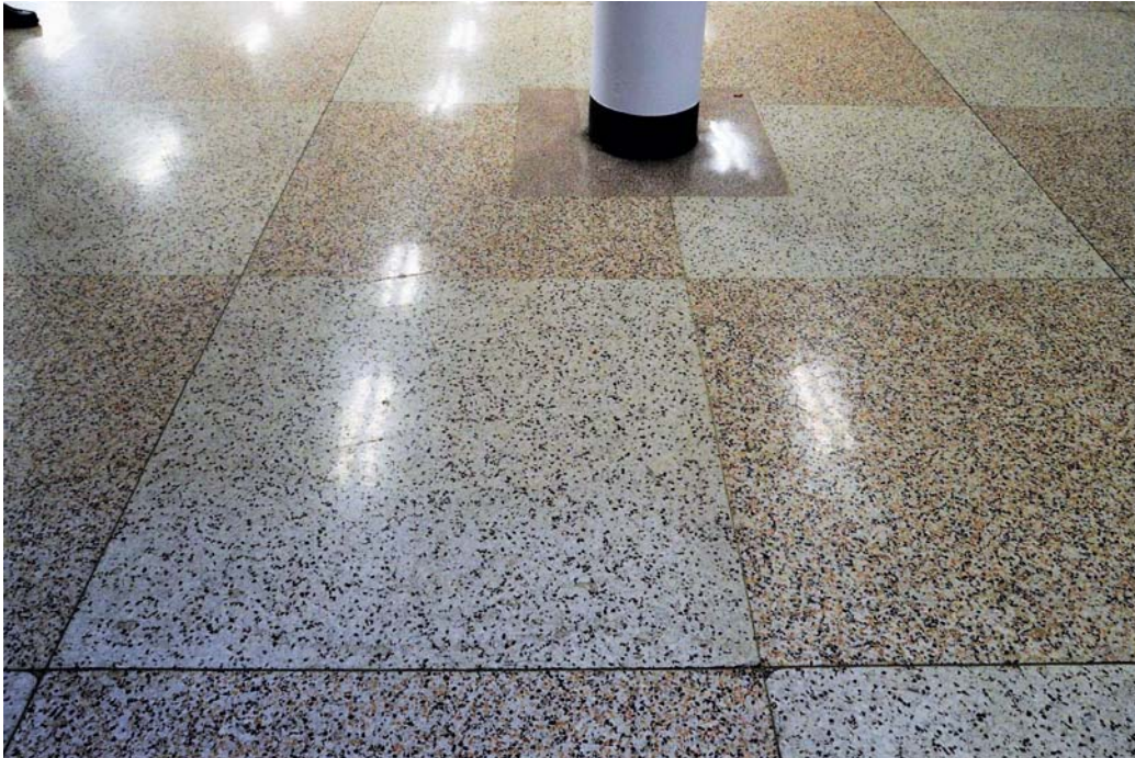
Fig. 151 Detail of cafeteria's terrazzo floor laid in a checkerboard pattern
