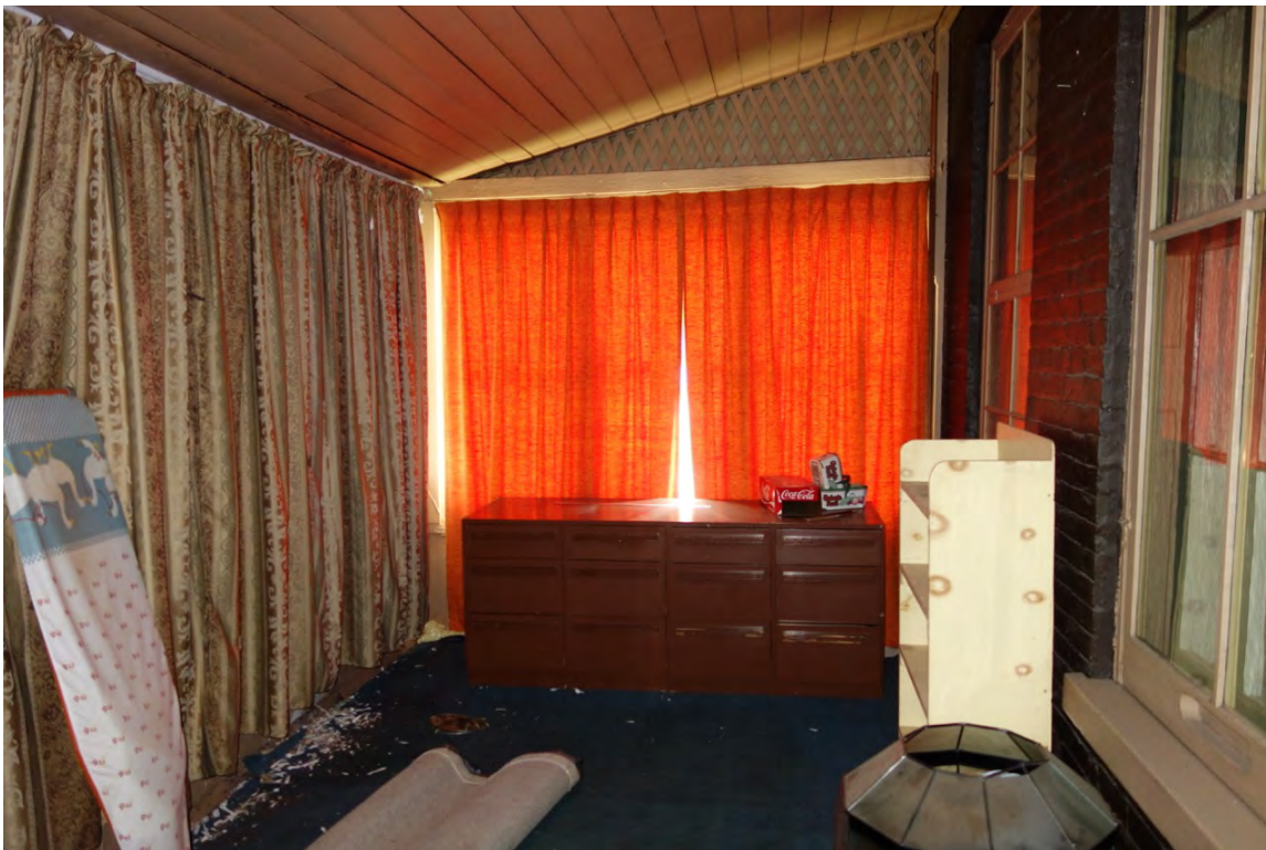
Porch – west end – tongue & groove wood ceiling
