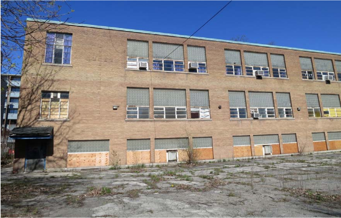
Fig. 63 Another view of the east elevation of 1951 wing
