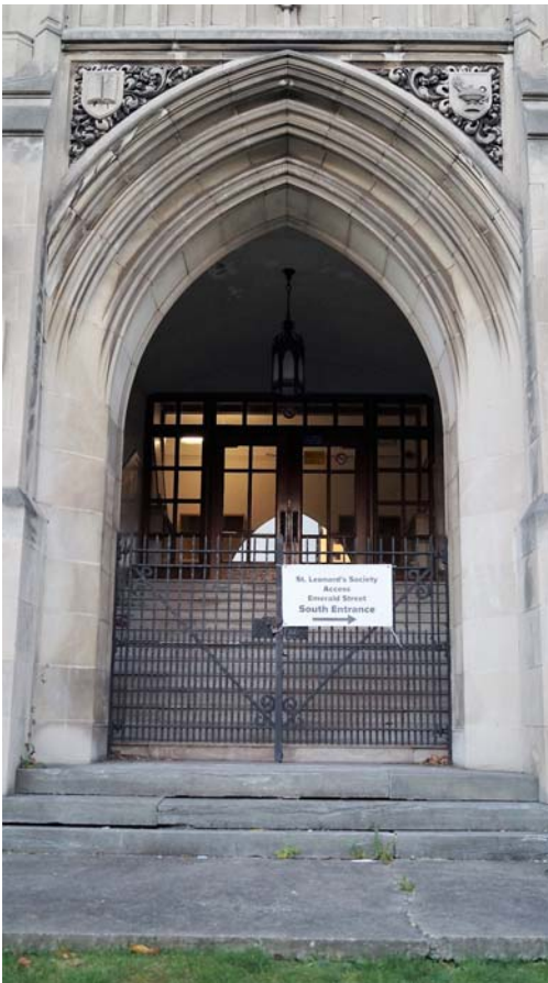
Fig. 29 Front entrance portal
