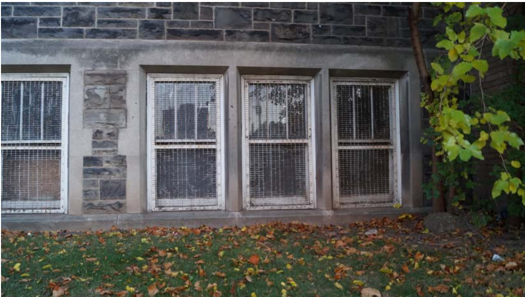
Fig. 68 Triple basement window in west facade
