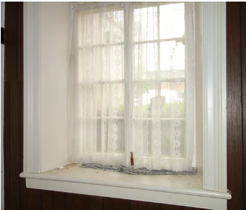
Bedroom 2 – wood casement window
