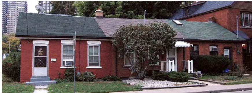
Typical one-storey row housing built in Corktown (mid-19 th century)
