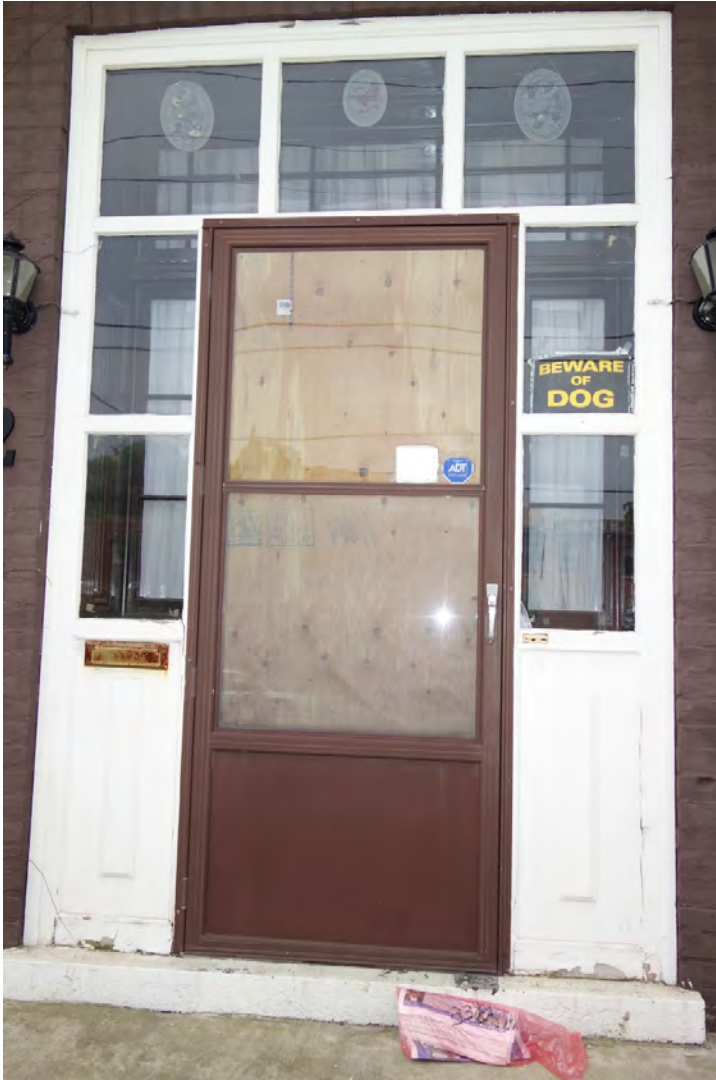
Front entrance with wood storm with modern metal door
