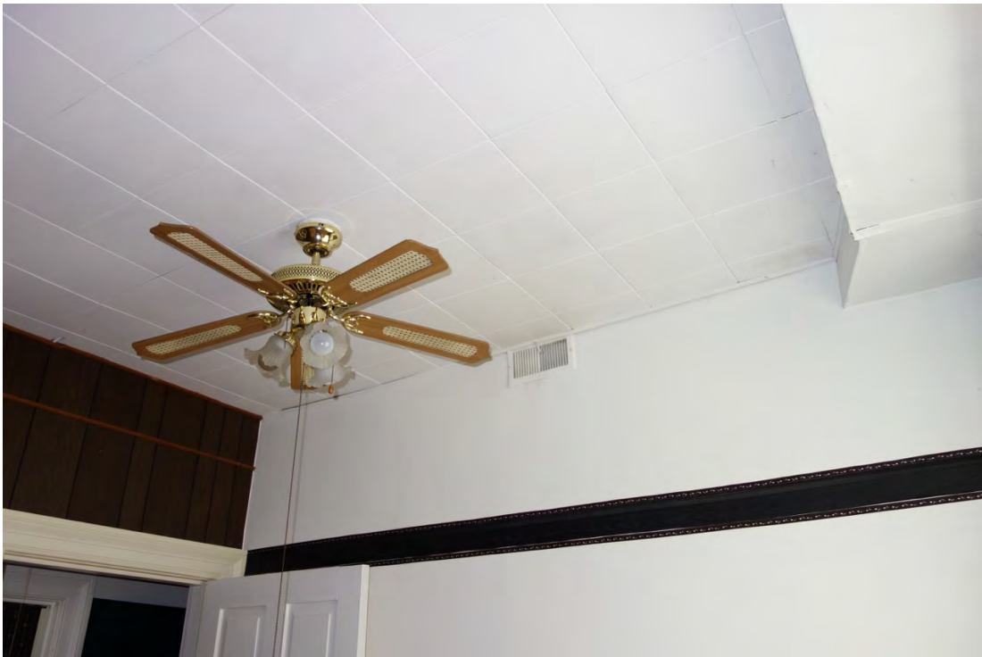
Bedroom 2 – modern ceiling tiles
