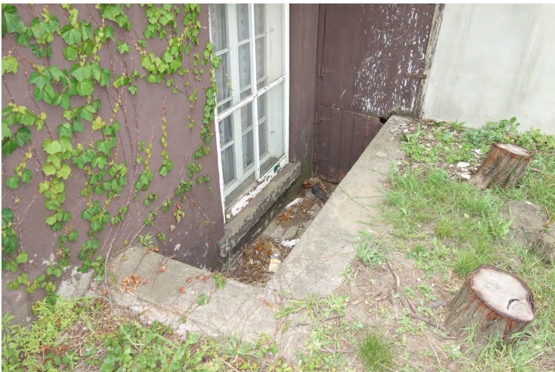
Modern concrete window well
