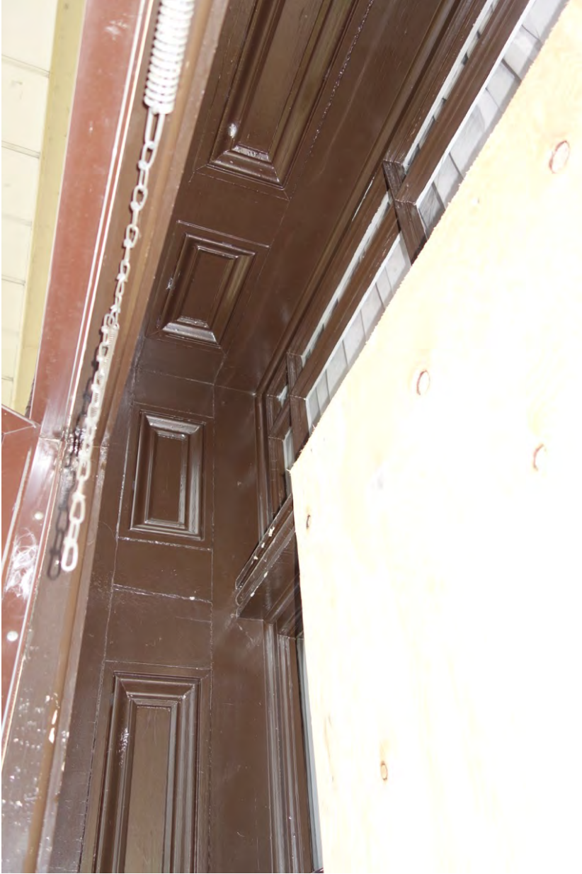
Front entrance wood paneling
