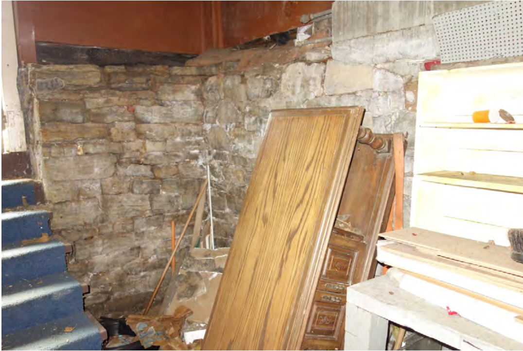
Exterior wall of porch - rubble stone
