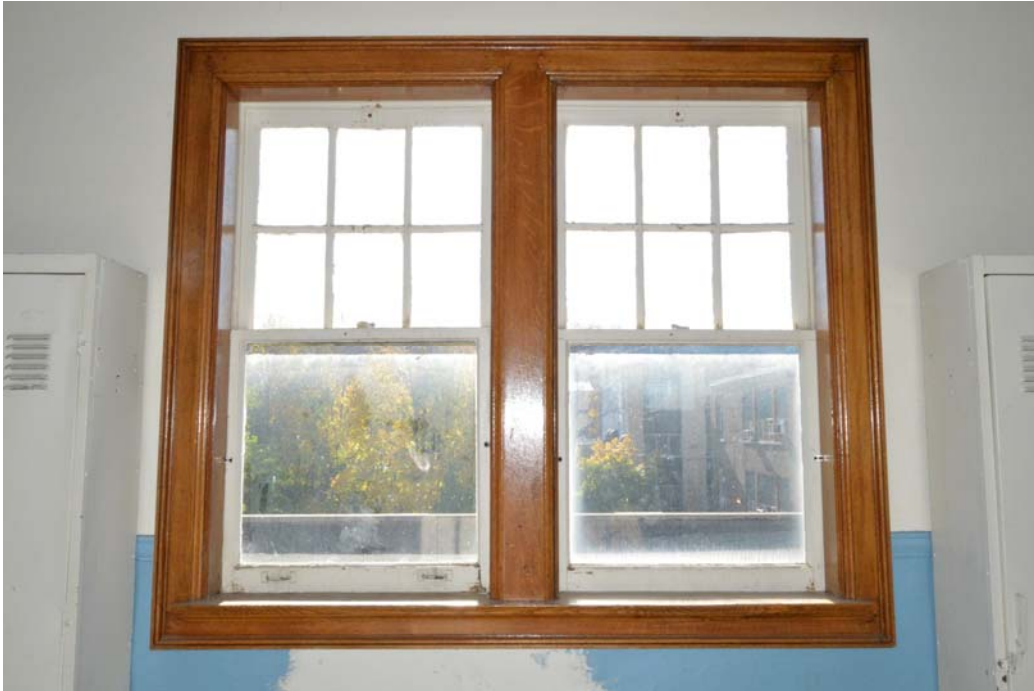
Fig. 97 South-facing window pair on upper-floor corridor
