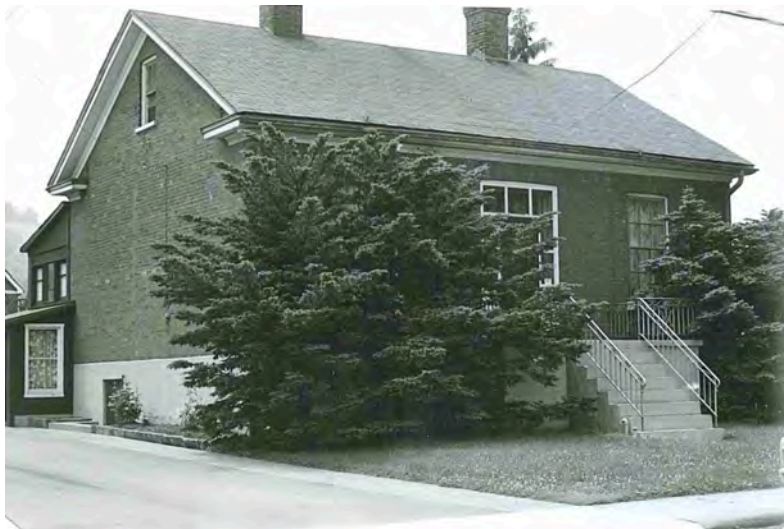
1973 photo showing two brick chimneys that have since been removed.
