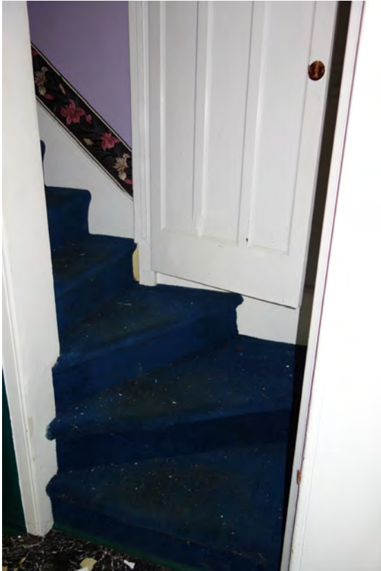
Kitchen – stairs to main floor
