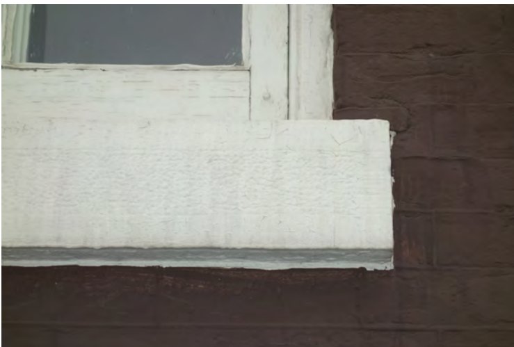
Dressed stone window sill on main elevation
