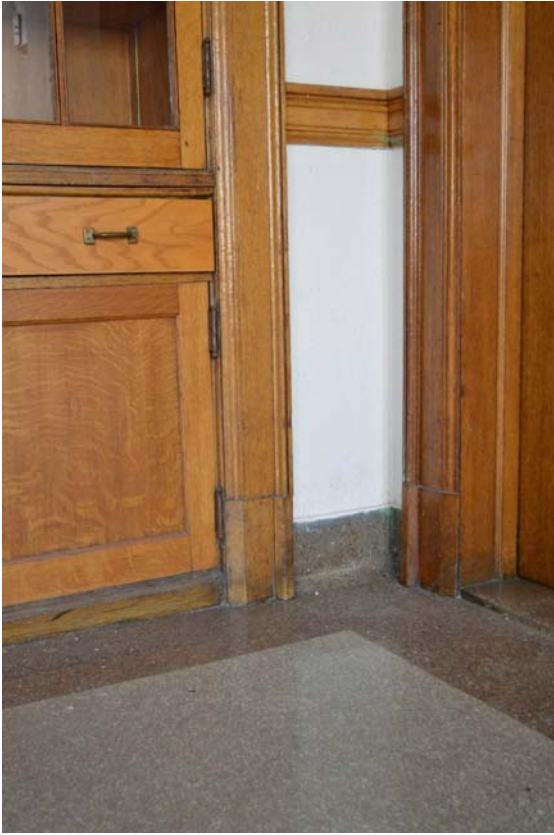
Fig. 103 Room 26 detail of grey terrazzo floor, brownish terrazzo border and baseboard, built-in oak cabinet, oak chair rail and oak door casing
