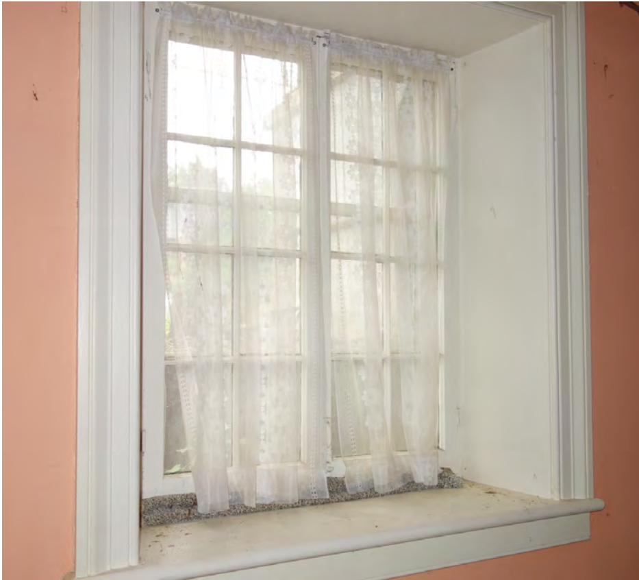
Bedroom 1 – wood casement window
