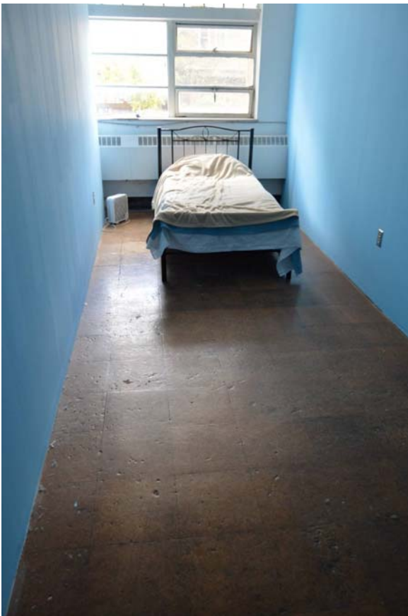
Fig. 142 Sample room on ground floor. Note cork floor from 1951 construction.
