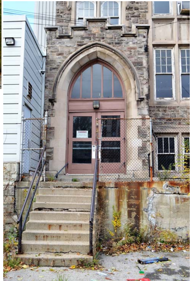
Fig. 54 East entrance vestibule
