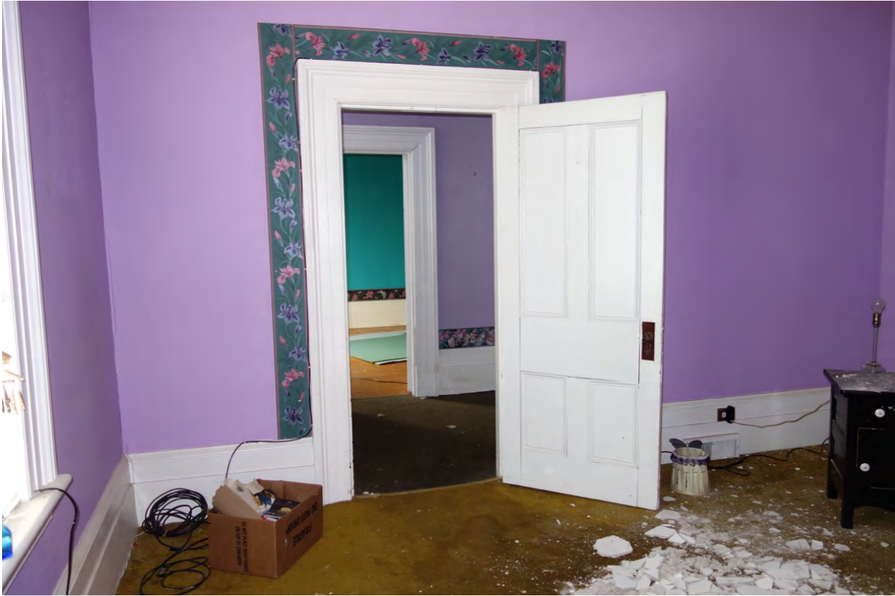
West parlour – door to hallway
