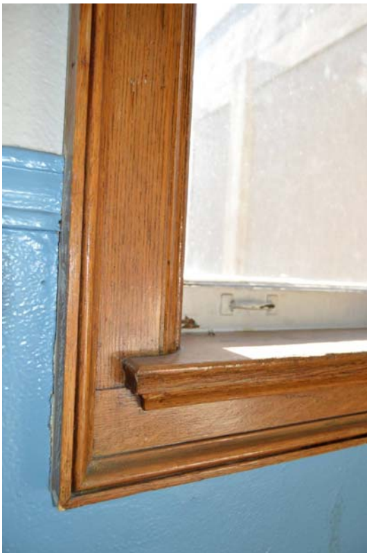
Fig. 98 Detail of oak surrounds for south-facing window pair
