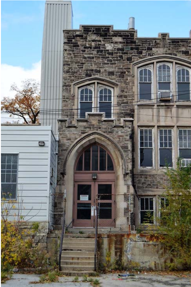
Fig. 53 East entrance bay
