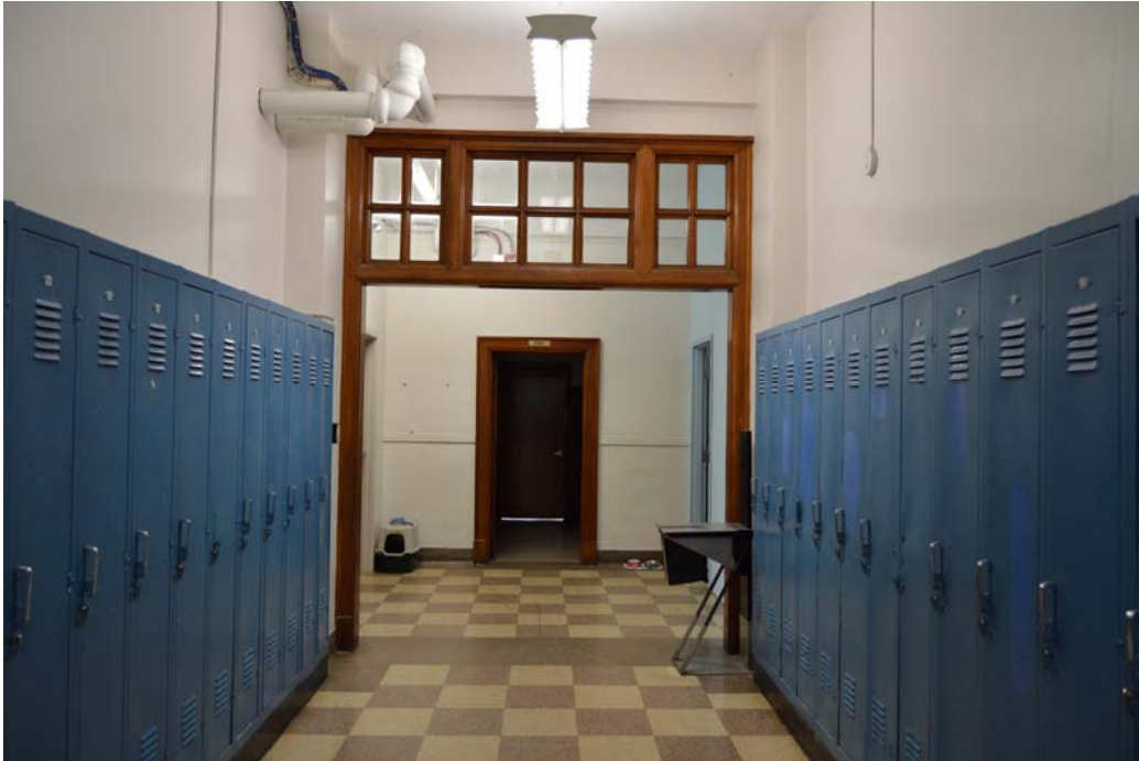
Fig. 80 Transom light over north-south corridor opening
