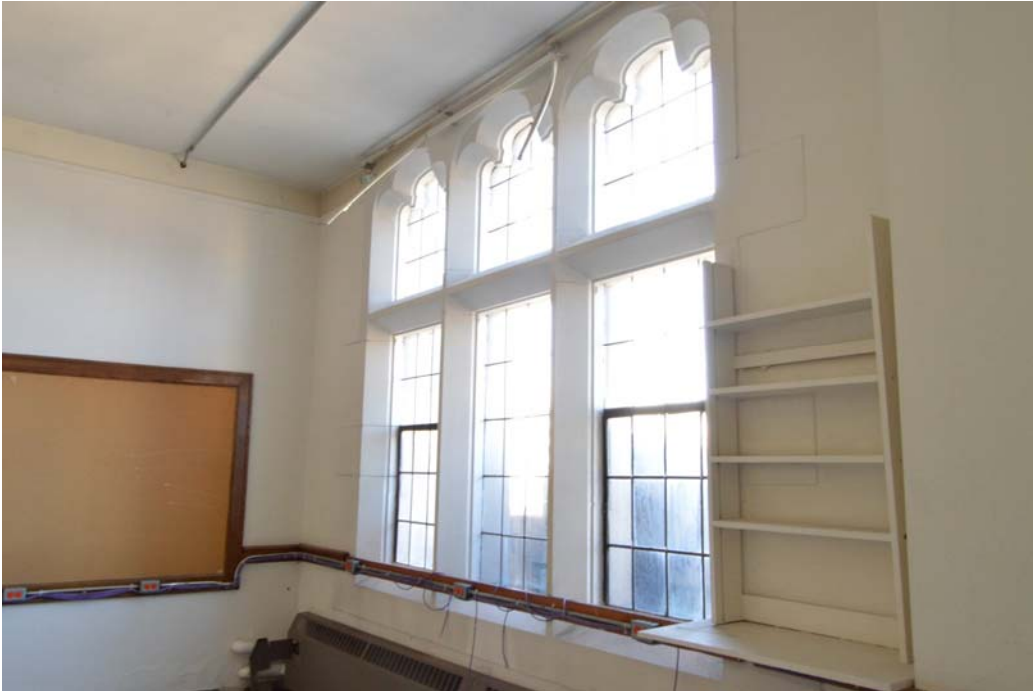
Fig. 111 Room 28 tripartite window in front facade entrance bay
