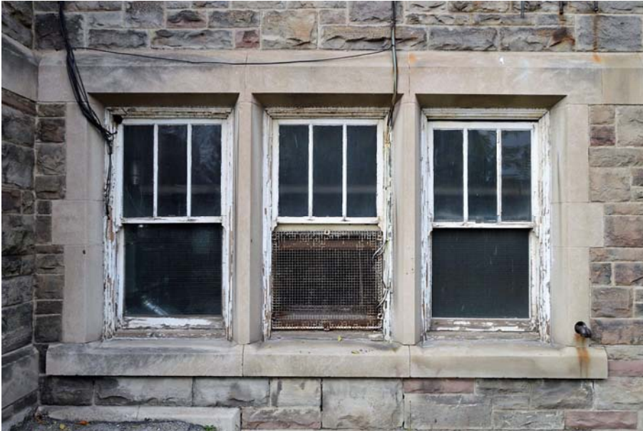
Fig. 57 Triple basement window in east facade
