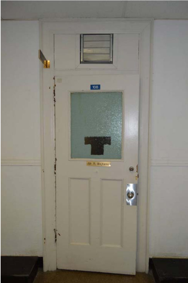
Fig. 119 Room 108 corridor door in basement
