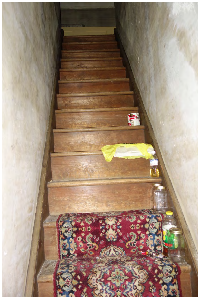
Enclosed stairs to the attic
