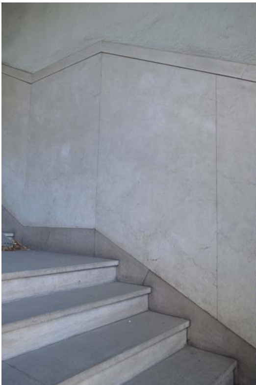
Fig. 36 Detail of marble staircase and wainscoting (dado)
