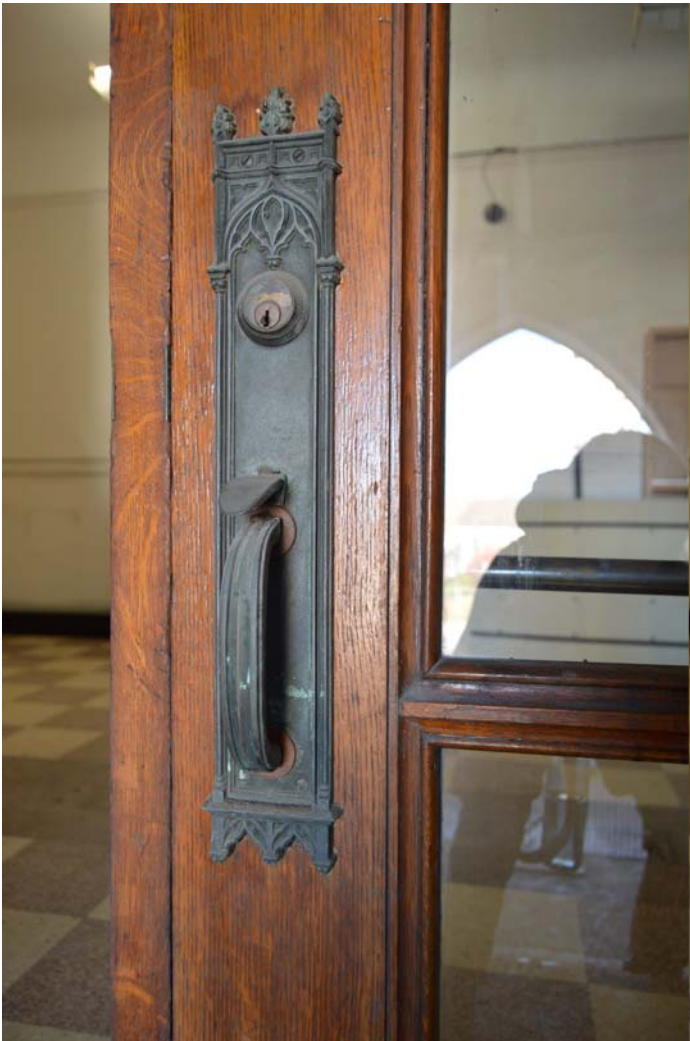
Fig. 39 Cast-iron door handle and escutcheon on stained oak and glazed doorway into vestibule. Note pointed arch in the design of the escutcheon.
