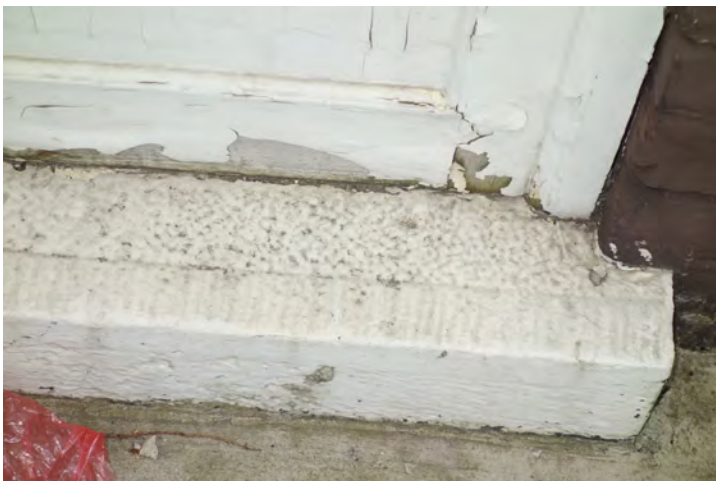
Dressed stone door sill at main entrance
