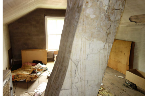
Attic room (freestanding chimney flue)
