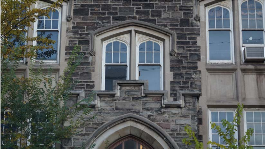
Fig. 67 Pair of windows in west entrance bay
