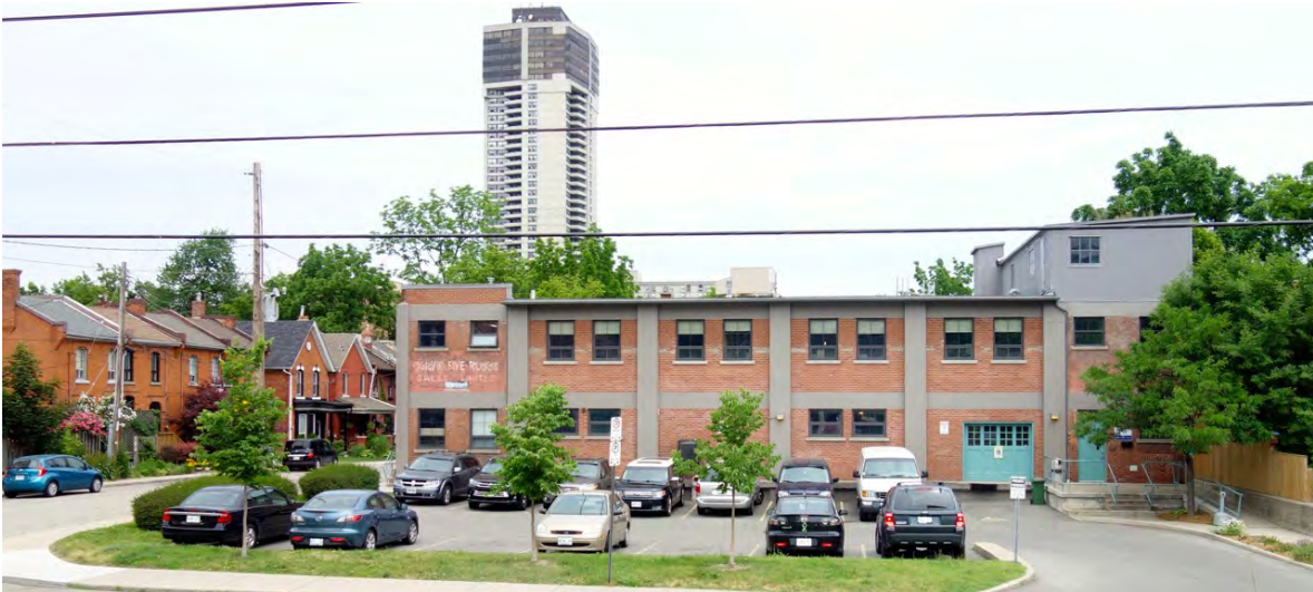
North side of Augusta Street – view from the subject property of the intact 19 th century streetscape on west side of Baillie Street (left) and the former Five Roses flour mill directly opposite
