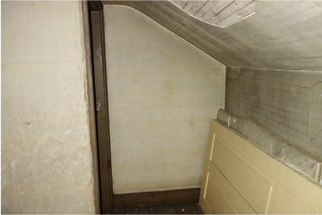
Attic hallway – west end
