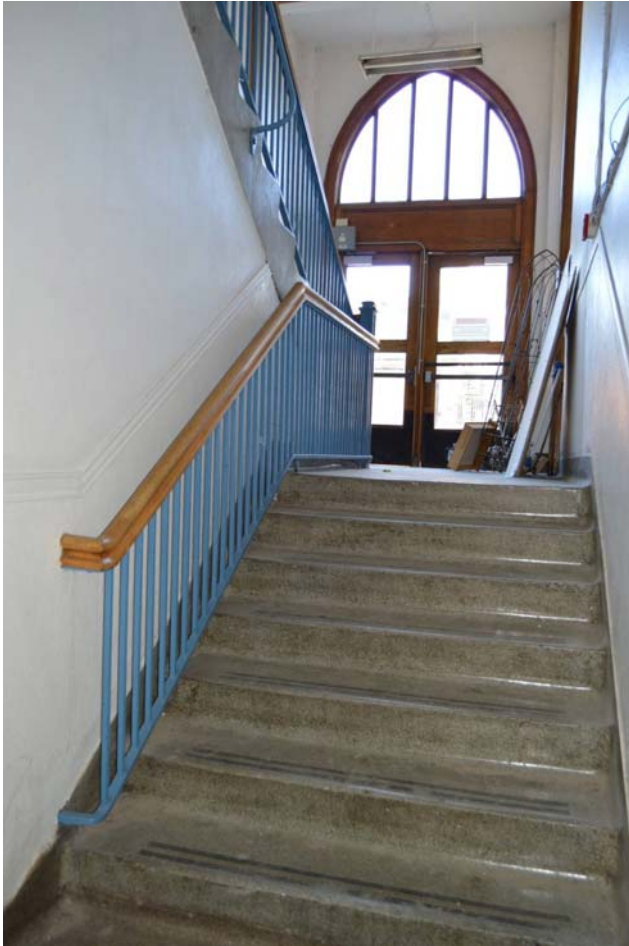
Fig. 129 Basement stairs, looking up to east vestibule entrance
