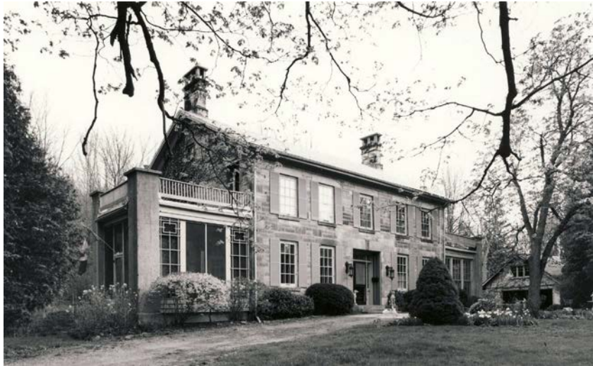
Figure 5: Front facade showing eastern addition (Flamborough Archives, 2002)
