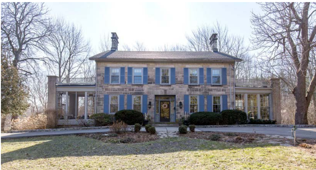
Figure 1: Front Facade of 6 Websters Falls Rd (Woolcott Realty, 2018)
