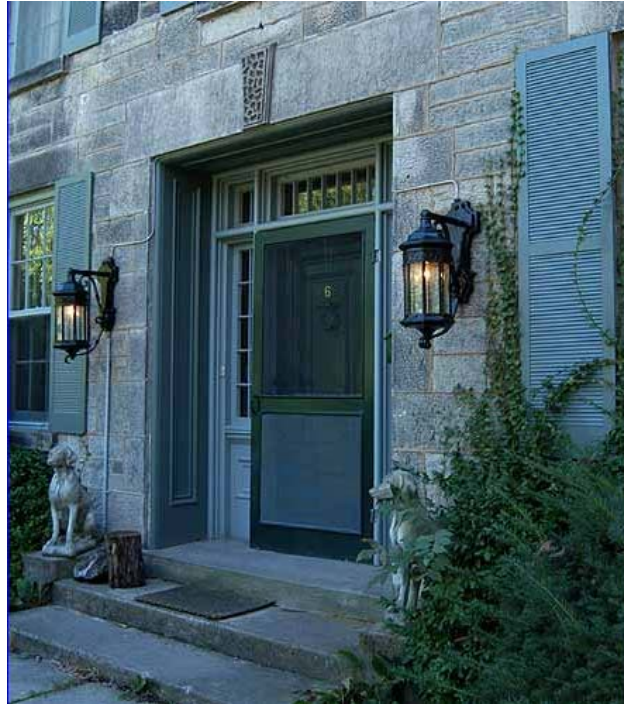
Figure 4: Front entrance to dwelling, showing transom, sidelights, lintel and quoins (Shannon Kyle, Ontario Architecture)
