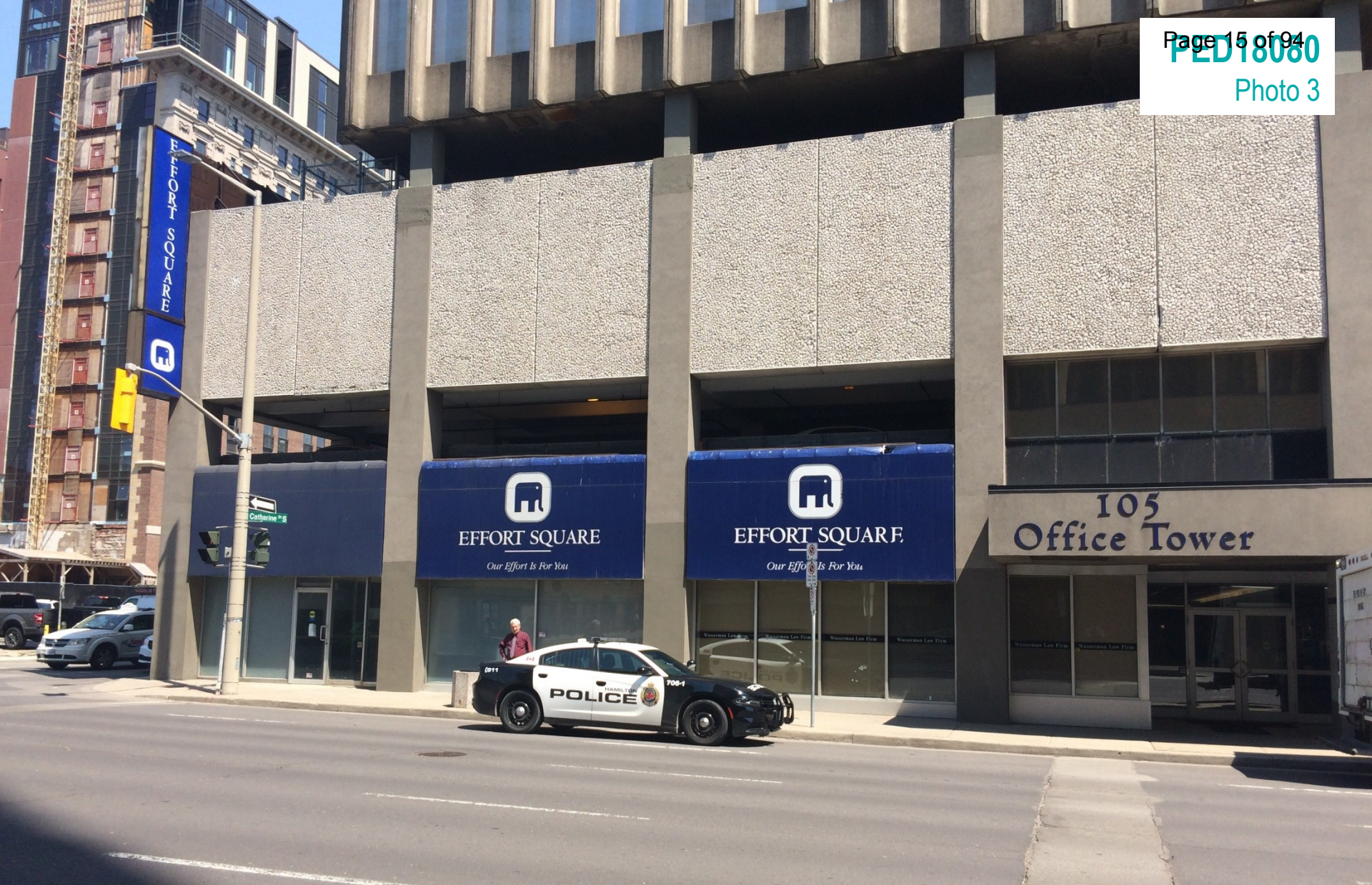
Existing building on the Subject Property as seen from Main Street East looking north
