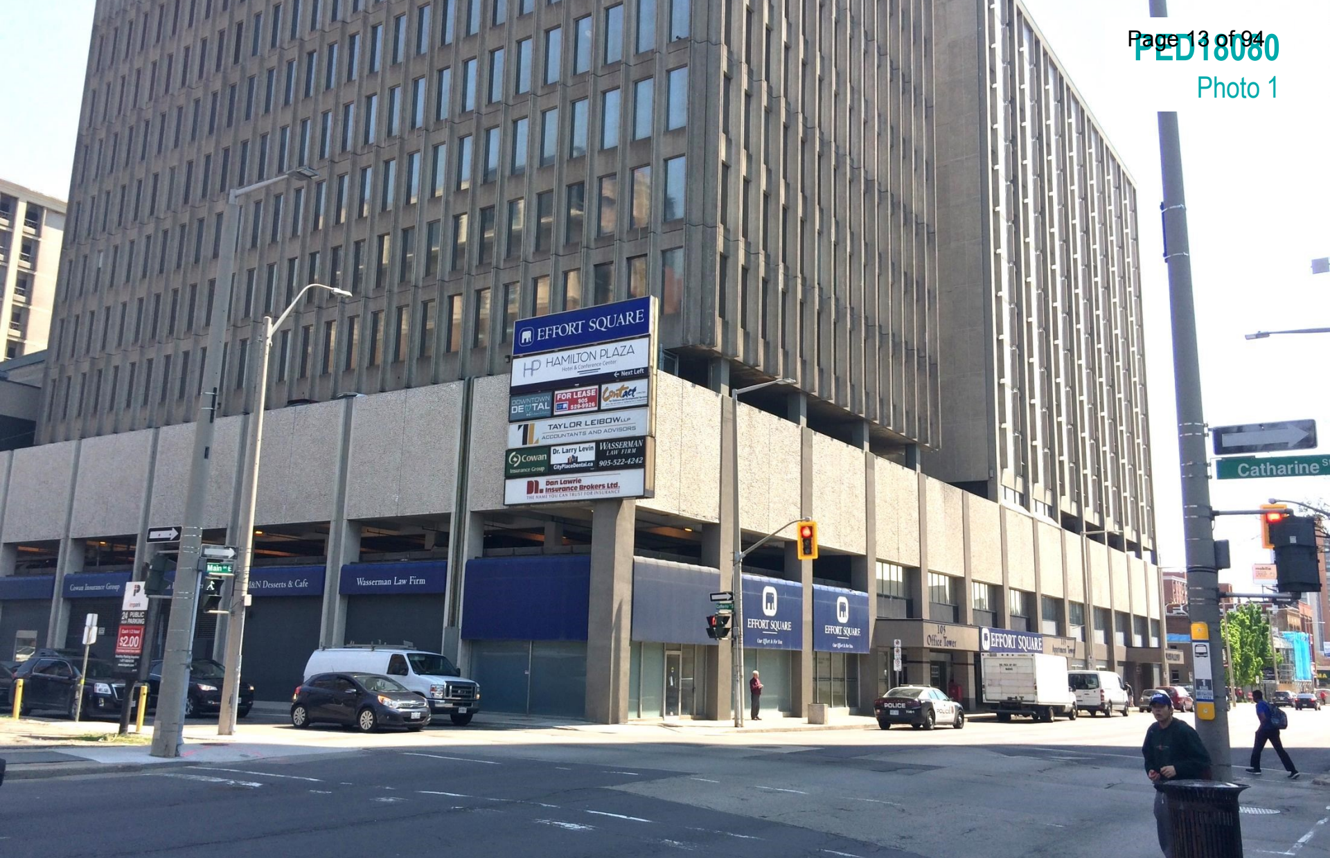
Existing building on the Subject Property as seen from Main Street East looking north east
