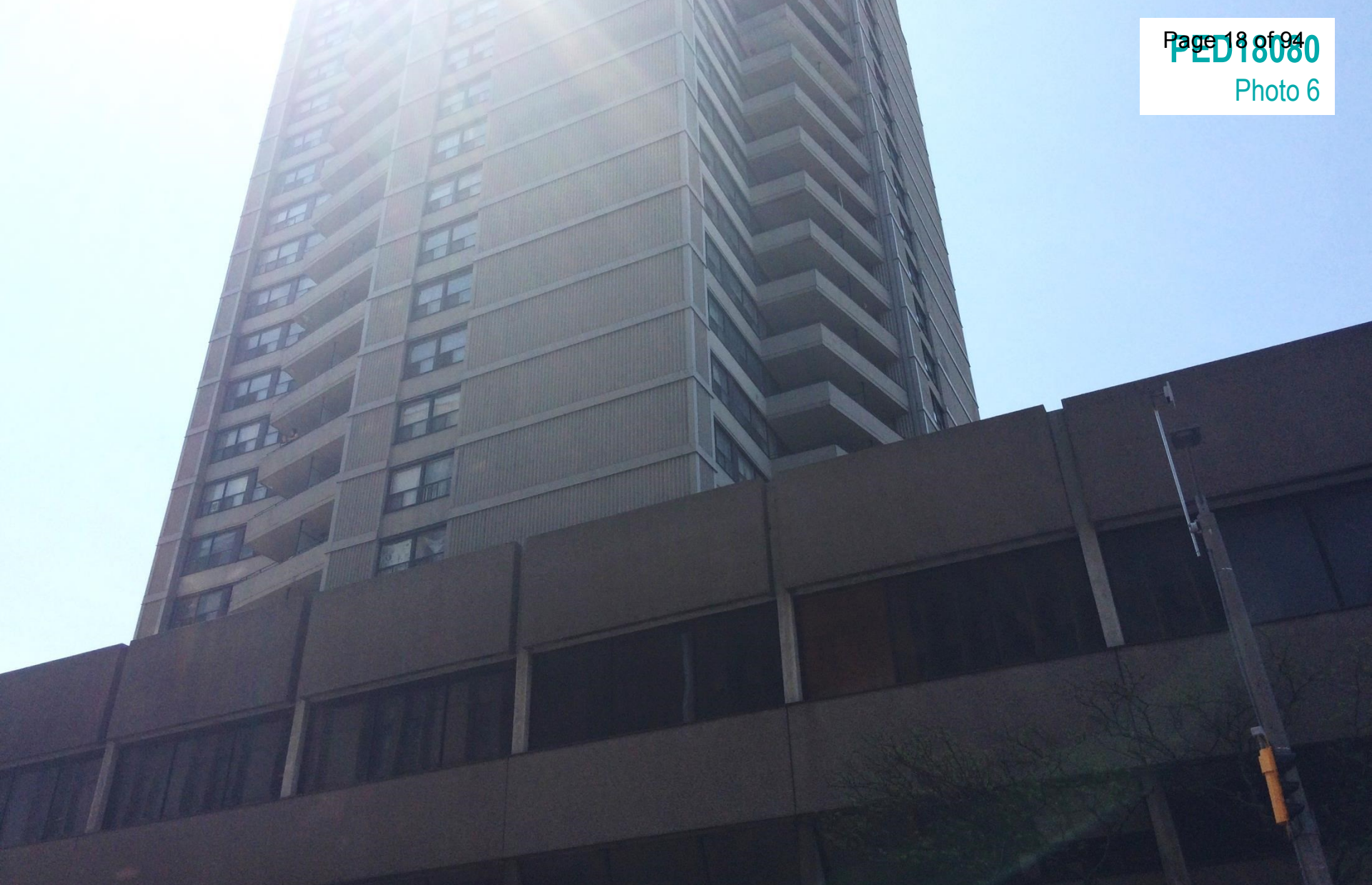
Existing tower of Landmark Place located to the south of the Subject Property, as seen from Main Street East looking south
