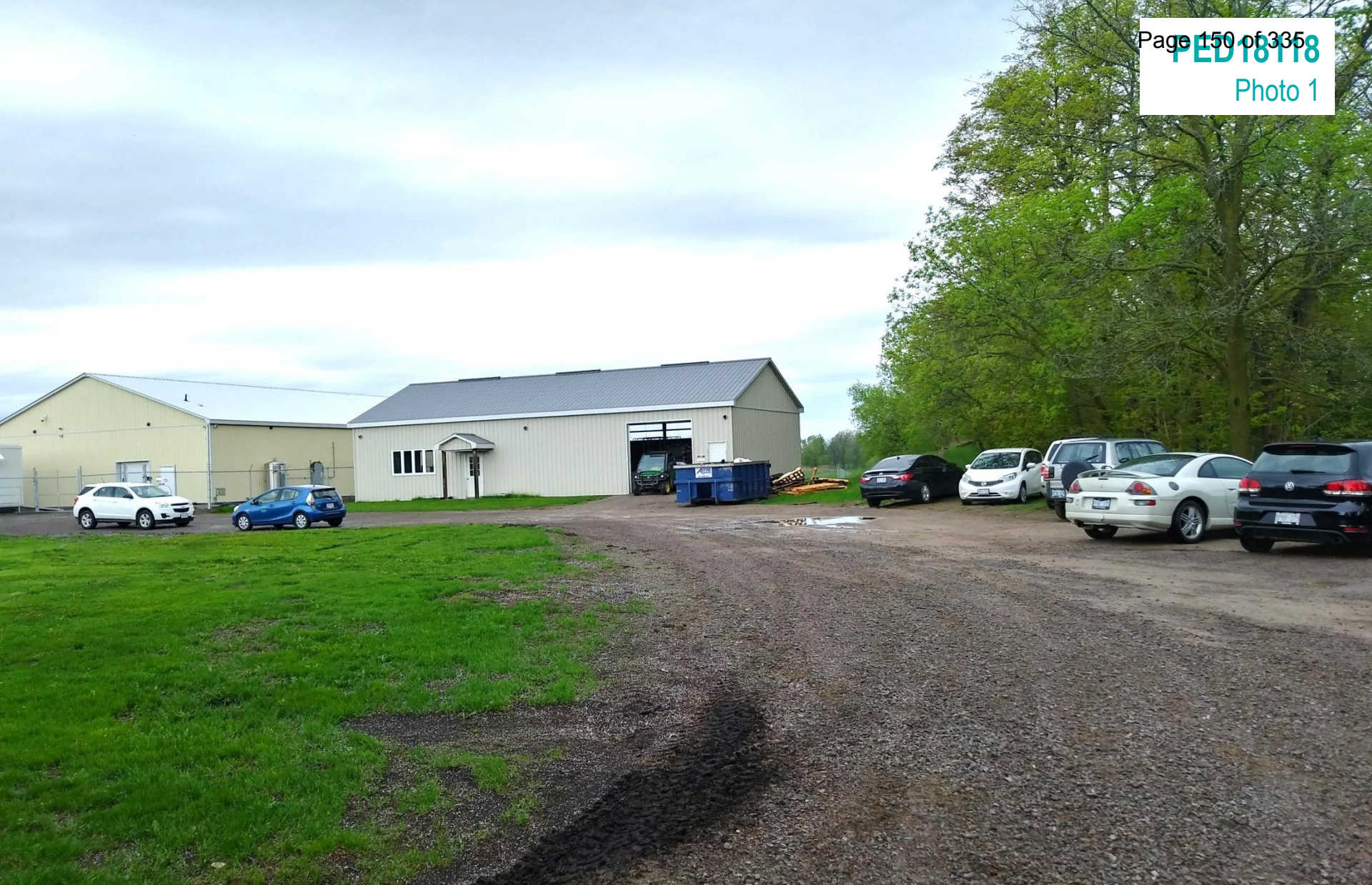
Existing medical marihuana facility, as seen from private road access
