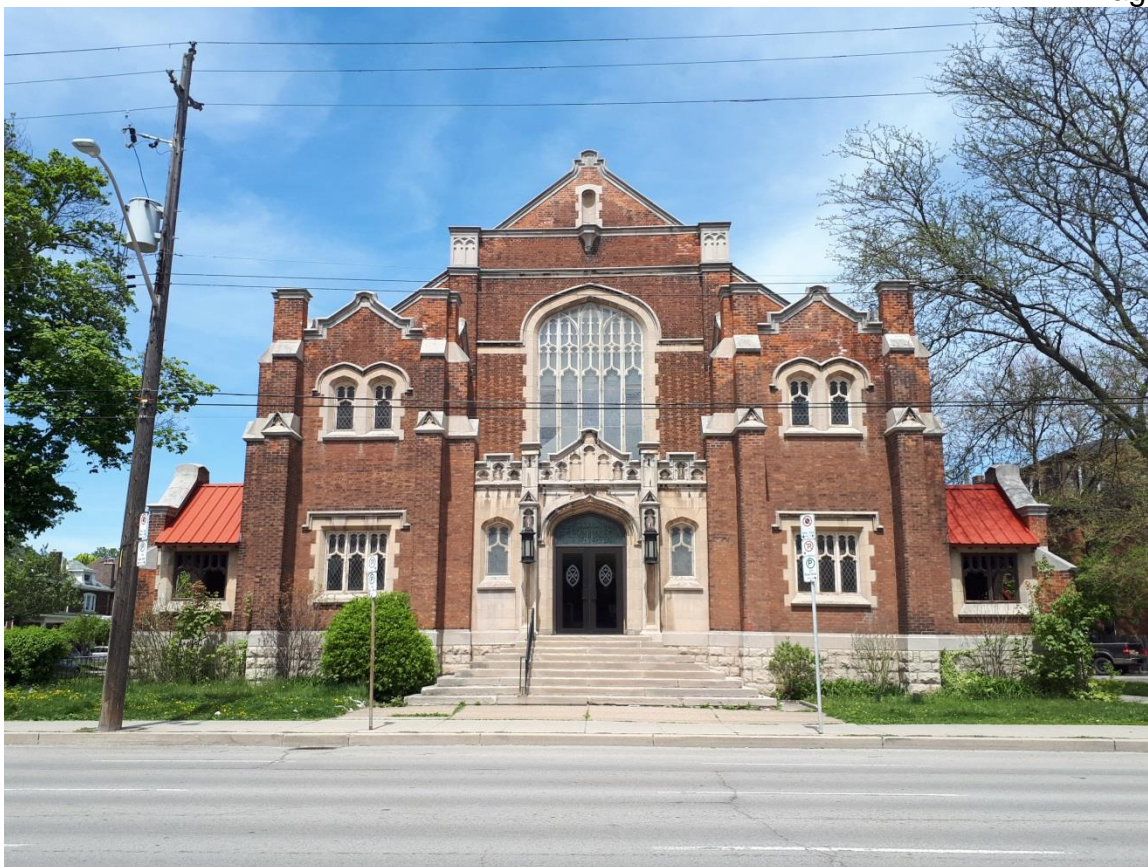
Front Façade, May 18, 2018
