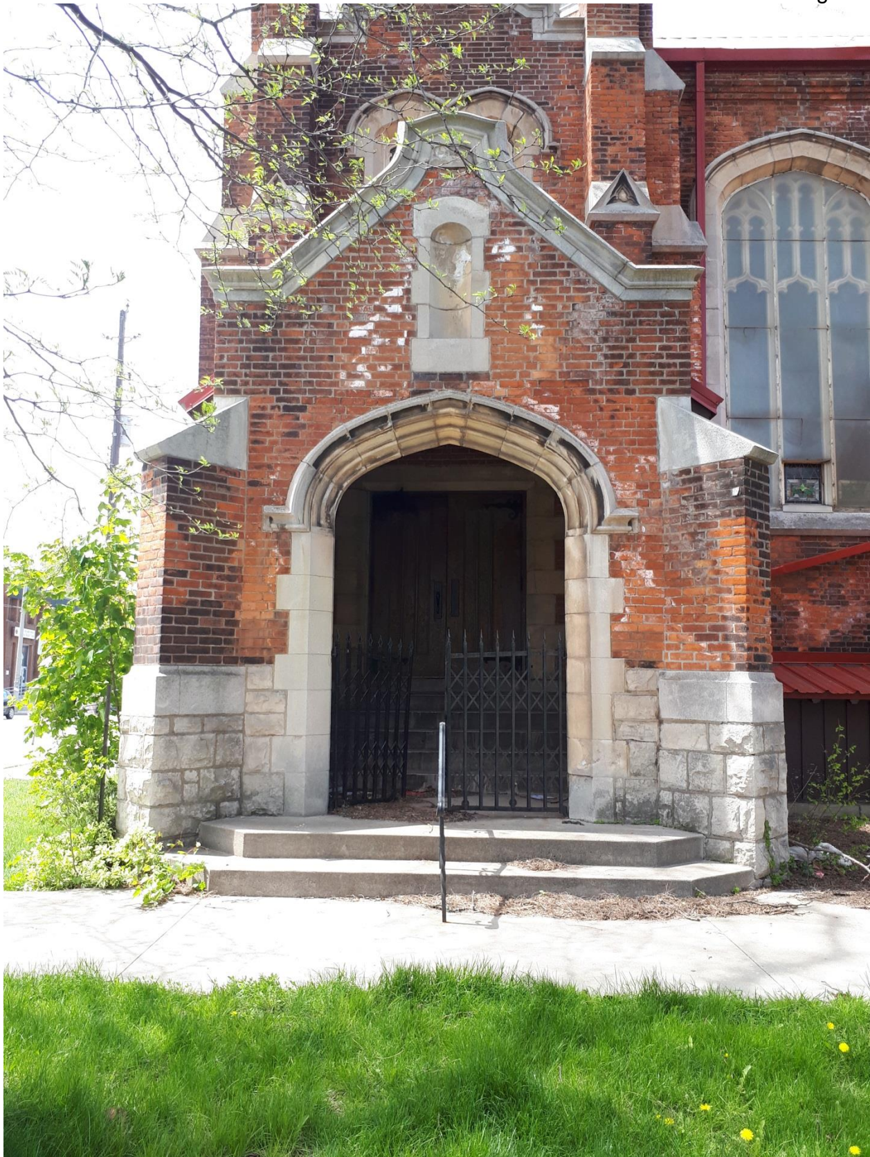
Close up of East Elevation Side Entrance, May 18, 2018
