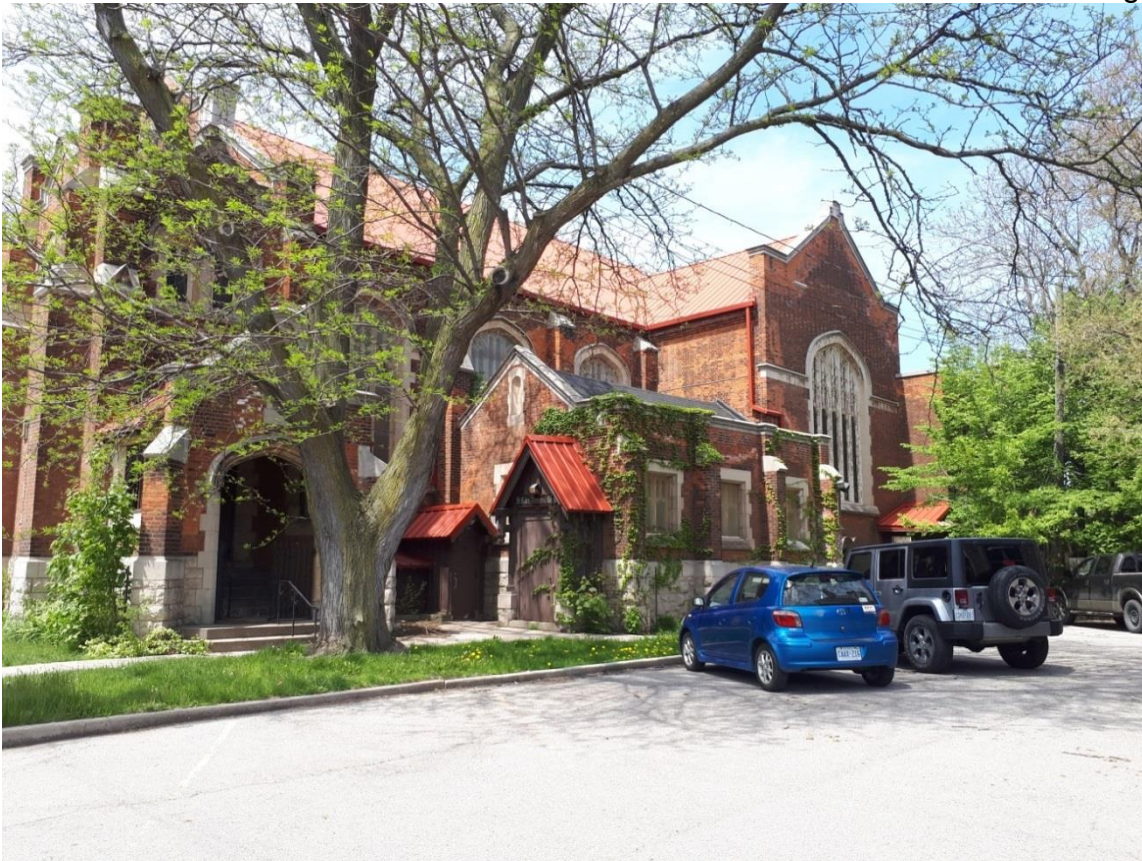
East Elevation, May 18, 2018
