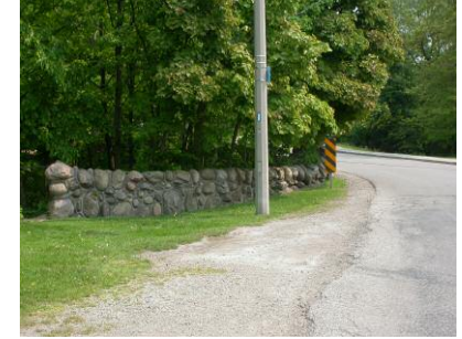
▲ Stone wall and pillar at vehicular bridge
