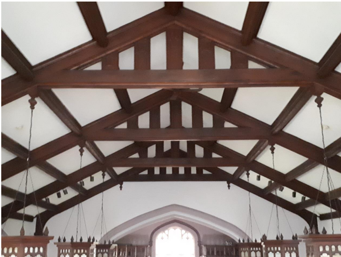
Wooden trusses, May 31, 2018
