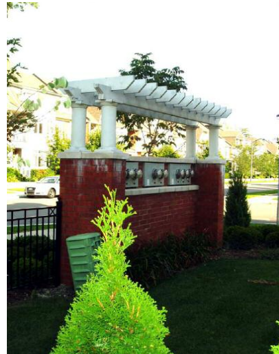
▲ Screen utilities that are at street level with architectural walls and/or landscaping
