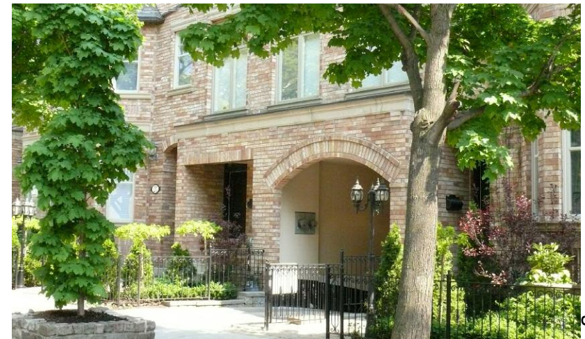
▲ Underground parking ramp is incorporated into the building design of this low-rise condominium.
