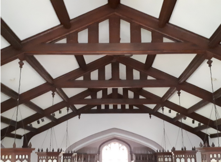
Wooden trusses, May 31, 2018
