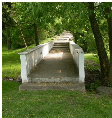
▲ Existing pedestrian bridge crosses Chedoke Creek Stream Corridor.
