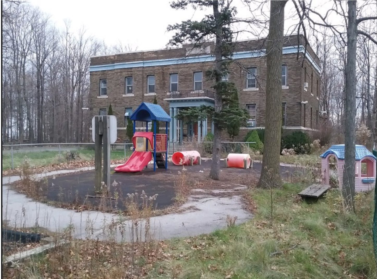
View of the building from the northeast. The children's play equipment is a reminder of its recent use as a daycare (Dan Collins, 2015).
