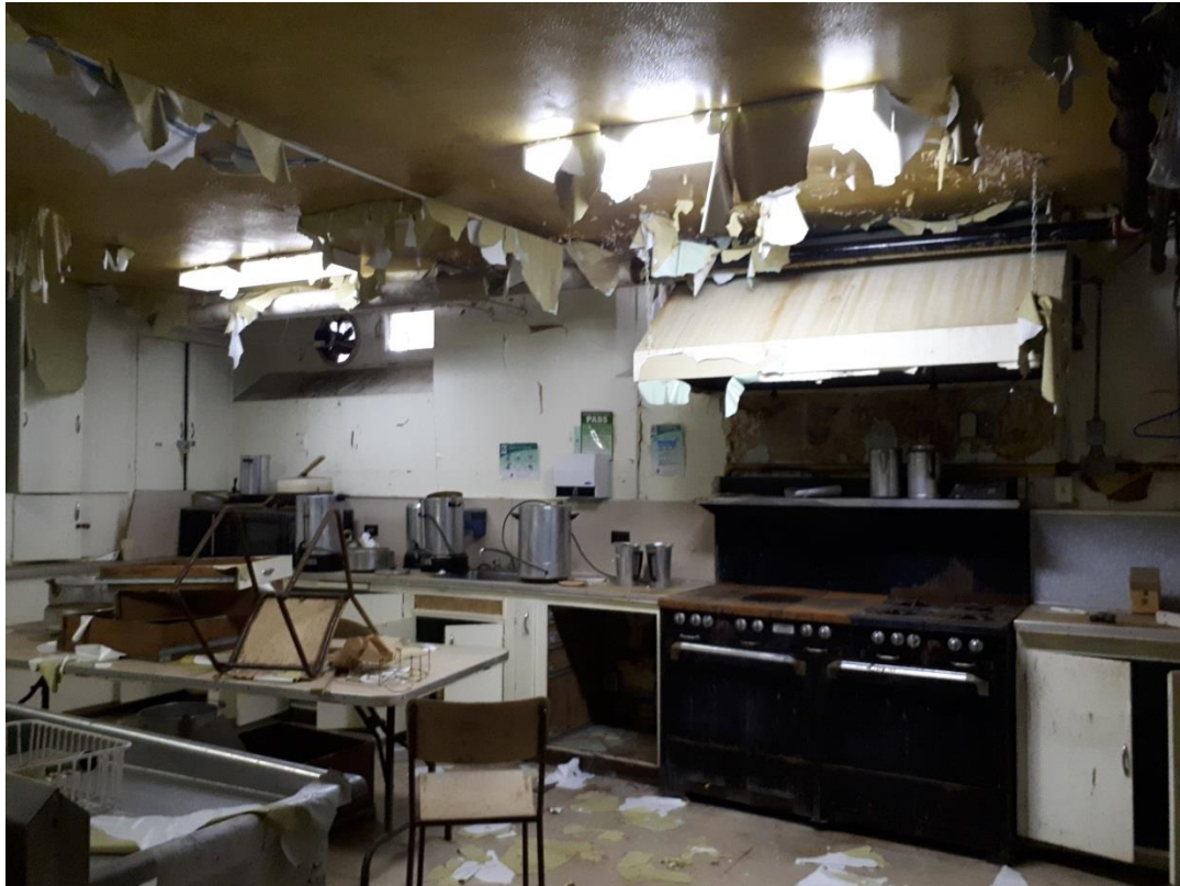
Basement kitchen, May 31, 2018
