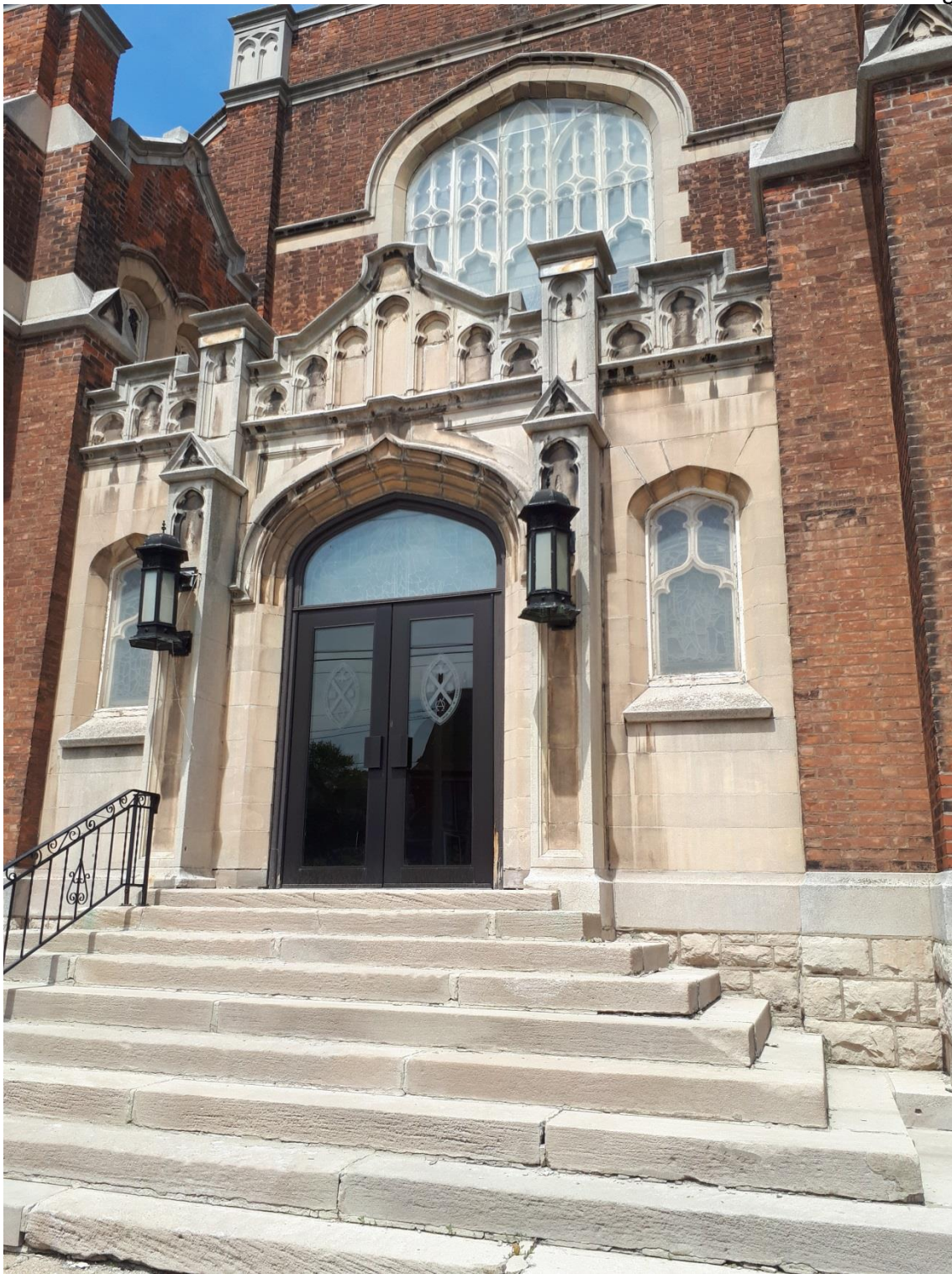
Front Entrance Close-up, May 18, 2018
