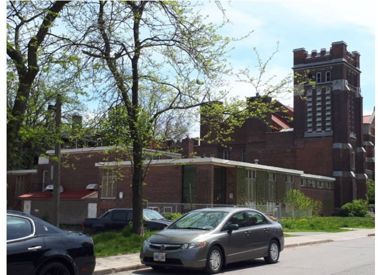
North Elevation, May 18, 2018
