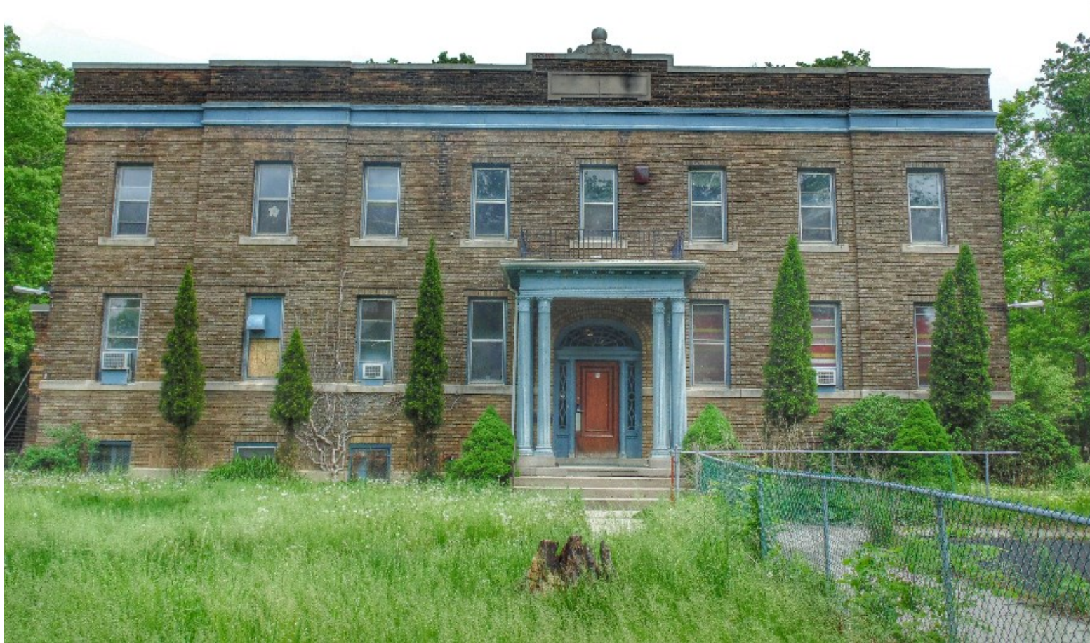
The façade of the Long & Bisby Building (Courtesy Goran Vla, 2016)
