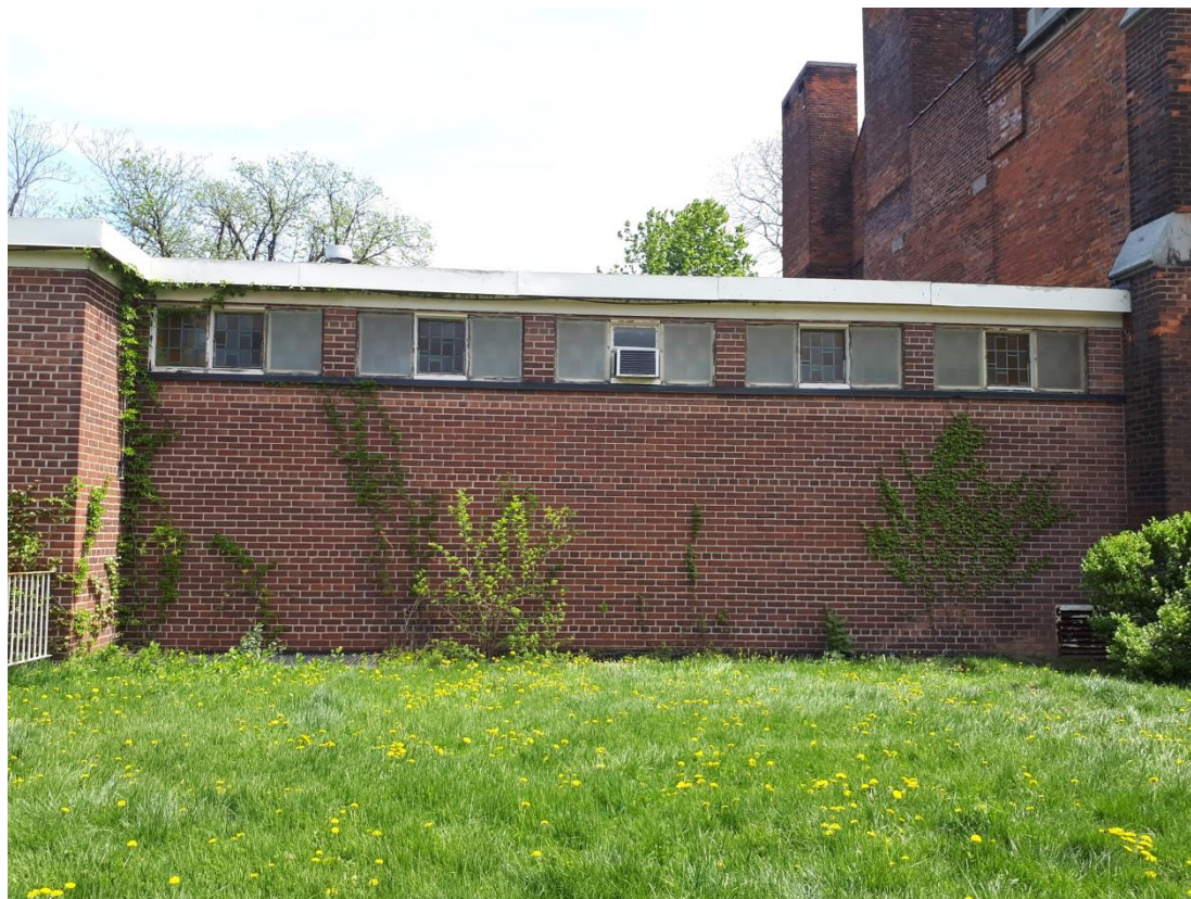
Close up of 1958 addition, May 18, 2018
