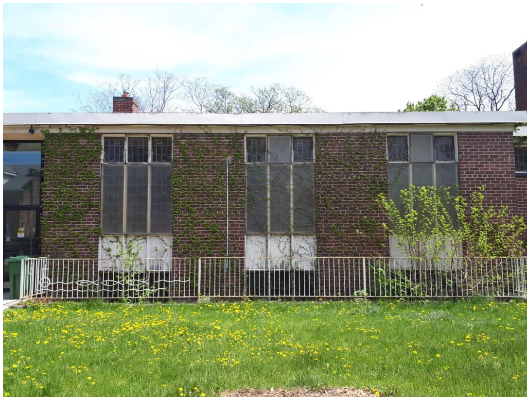
Close up of 1958 addition, May 18, 2018
