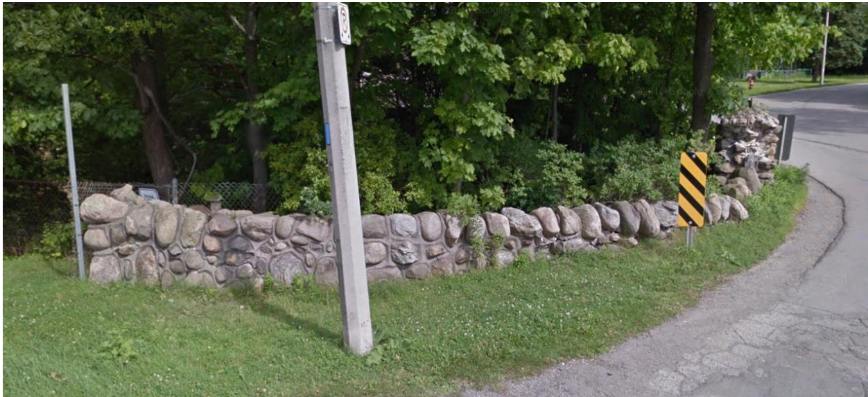
Figure 15: An image of the stone wall and pillars located between Sanatorium Road and the brow's edge (Google Street View, 2015).
