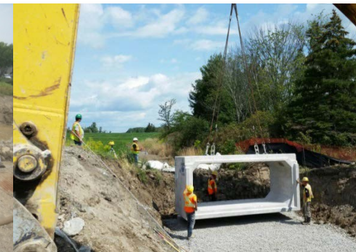
Bell Road Culvert Replacement
