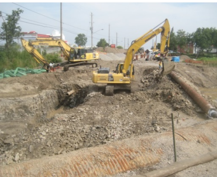
Dartnall Road Culvert
