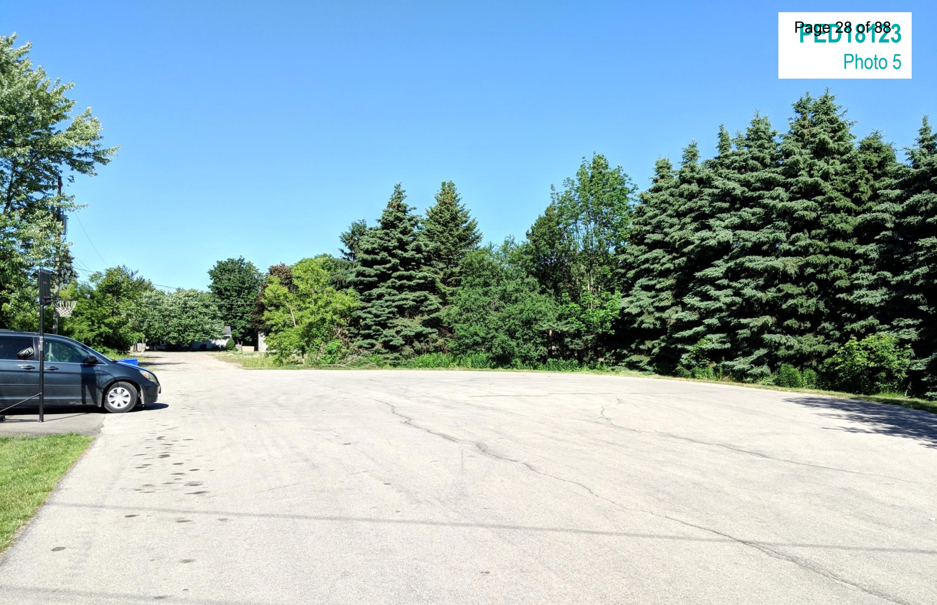
End of paved portion of Roselawn Avenue
