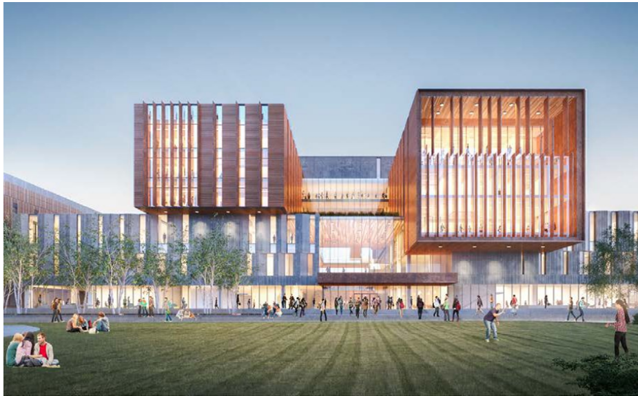
Mississauga Campus North Building, University of Toronto Perkins+Will
