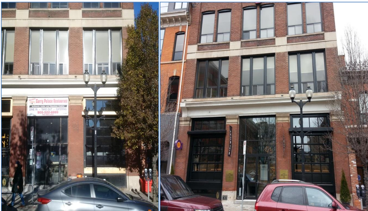
43 King William Street, Hamilton (before and after)
