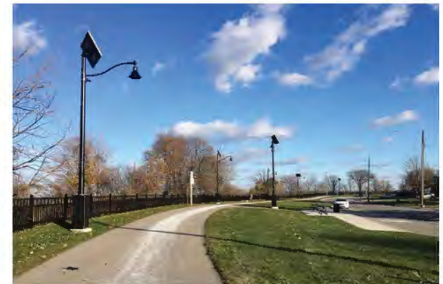
Exhibit 1 - Existing Mountain Brow Trail
