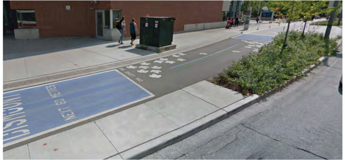
Exhibit 38- City of Toronto Waterfront Trail incorporating blue and green centreline, pavement marking decorations and blue and white stop bars (Source: Google Maps)
