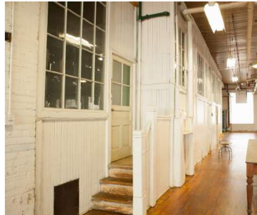
Figure 4.19 - Level 3: An interior wall that seems to be characteristic of an exterior envelope. It has similar character defining windows to those of the exterior and shows a progression of construction.
