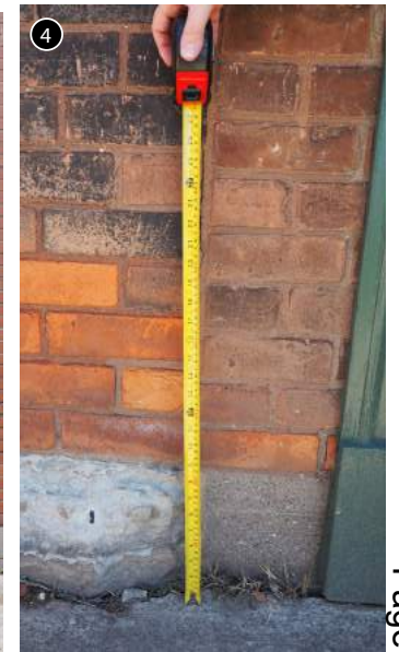
Figure 4.11 Connection between original Mill building office and addition
