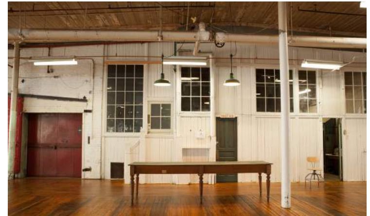
Figure 4.19 - Level 3: An interior wall that seems to be characteristic of an exterior envelope. It has similar character defining windows to those of the exterior and shows a progression of construction.
