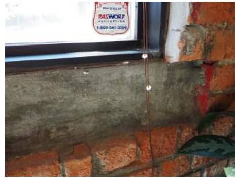
Stone lintel visible from interior window ledge
