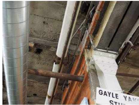
Condition where building 1948 addition required reinforcing steel post.
