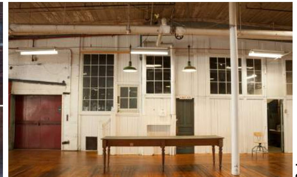
Figure 6.4- Mill Interiors: Original post and beam construction, wood floors and ceilings, original metal doors.
