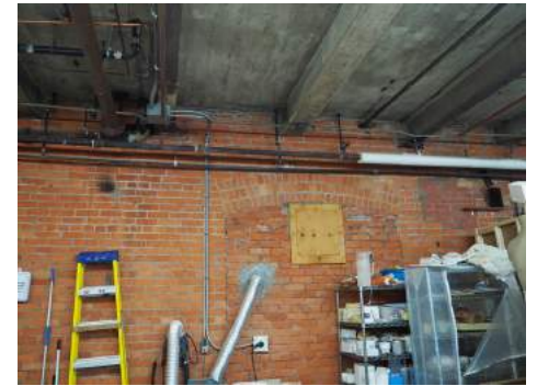
1948 addition wall, filled in window with brick
