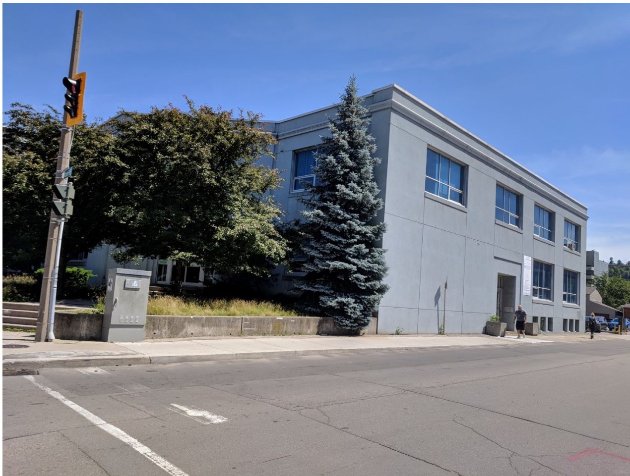
Image 4: View of the northwest façade of the Mainway Building (2018)
