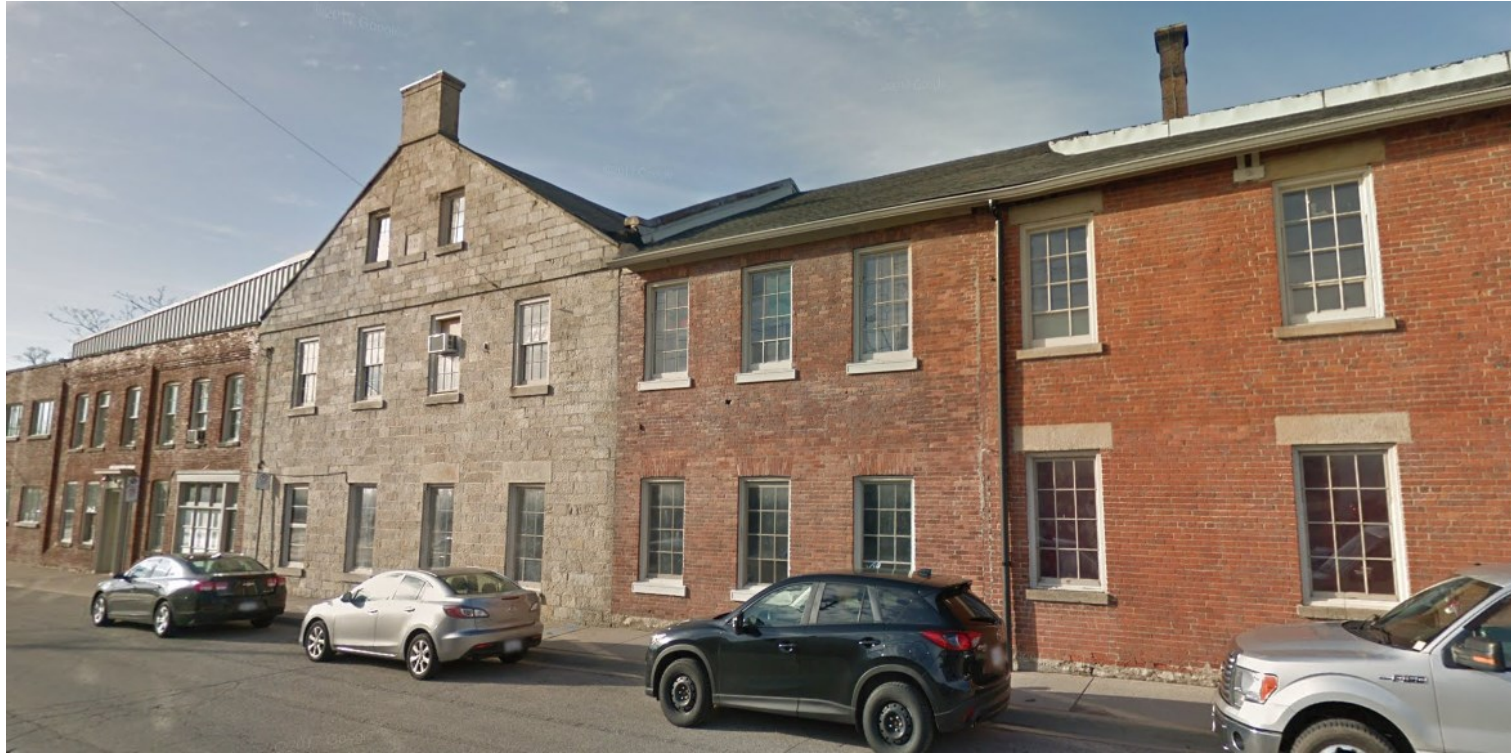
Image 3: View of the front façade of the historic Gartshore building at 64 Hatt Street in Dundas (Google Streetview, 2017).
