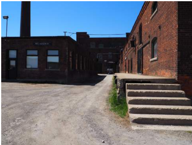
Figure 5.7 - (source: mcCallumSather) The TH&B Railway came directly into the site. The high platform indicated that the Storage Warehouse operated directly adjacent to the rail.
