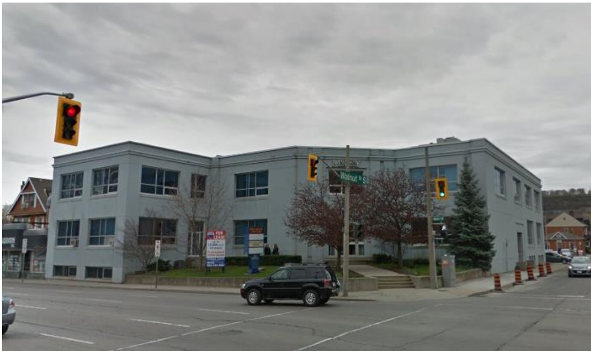
Image 2: View of the northeast façade of the Mainway Building (Google Streetview, 2017).
