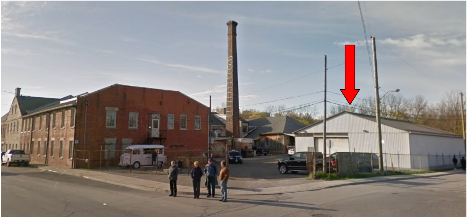
Image 2: View of the metal accessory building in relation to the Gartshore building at 64 Hatt Street in Dundas (Google Streetview, 2017).
