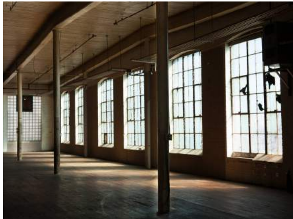
Figure 4.18 - Level 3: Large windows with 6 over 6 window panels, others with glass block infills
