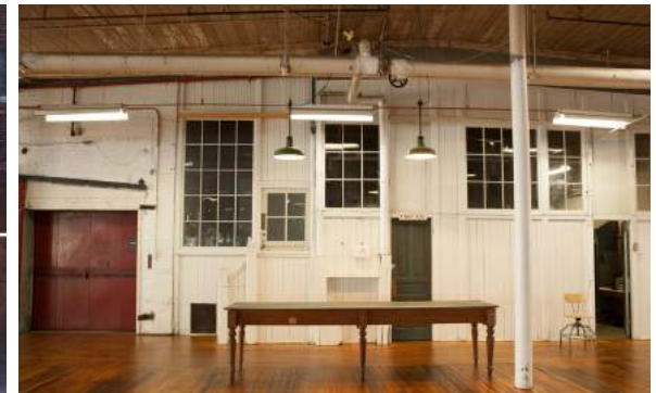
Figure 6.4- Mill Interiors: Original post and beam construction, wood floors and ceilings, original metal doors.
