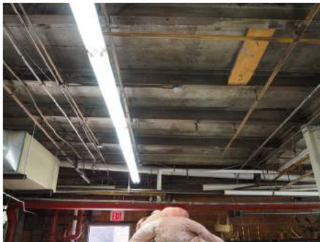
Exposed concrete ceiling (functioned as a 'wet floor' on Level 2) and steel beams.
