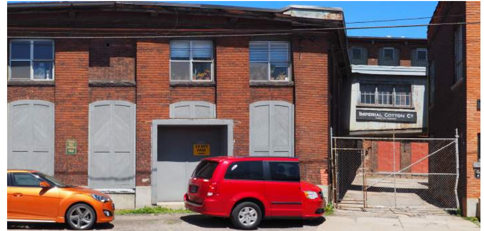
Figure 4.23 - South Elevation Detail
