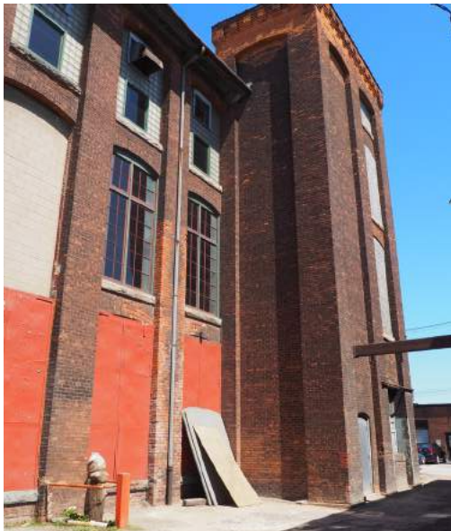
Figure 4.8 South East All original openings with ranging enclosure from plywood, glass block, and wood replacement windows.
