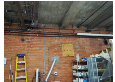
1948 addition wall, filled in window with brick
