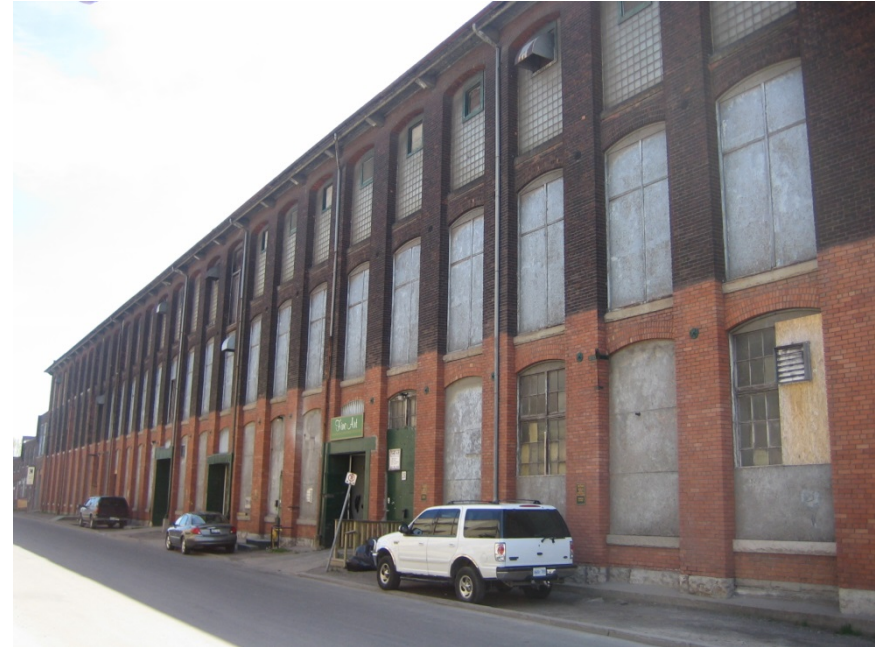
North elevation of Mill Building
