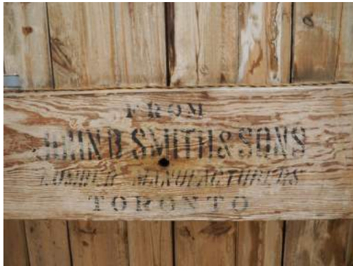
Figure 4.15 - Exposed timber beam and ceiling
