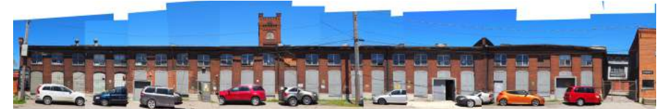
Figure 4.25 South Elevation Photo stitch
