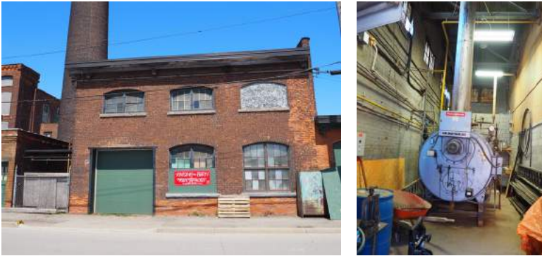
Figure 4.40 -This Utility Building housed the coal-boiler that operated the smoke stack.
