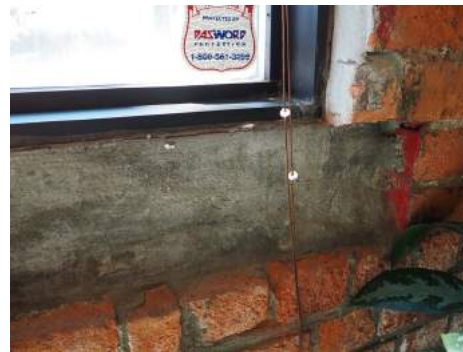
Stone lintel visible from interior window ledge
