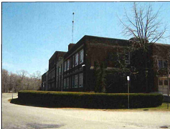
Oblique View to the Western End of the Brow Building from Sanatorium Road.
