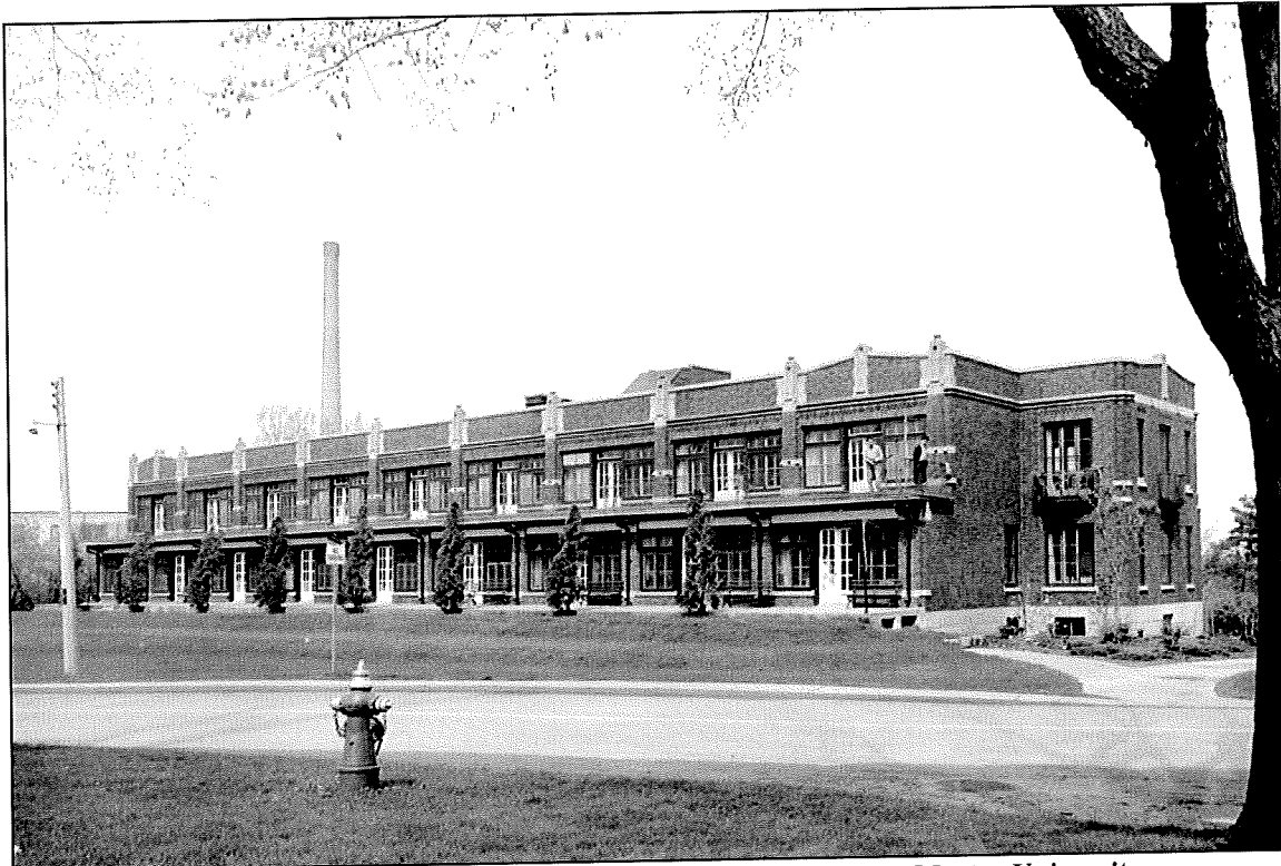
Southam Pavilion from Sanatorium Road [Health Sciences Library, McMaster University, Hamilton].
