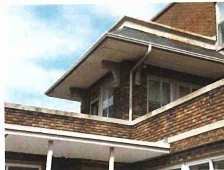
Sundeck (original brackets and roof flashings)
