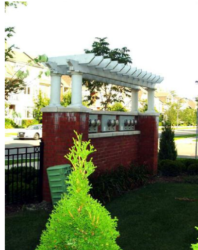
▲ Screen utilities that are at street level with architectural walls and/or landscaping
