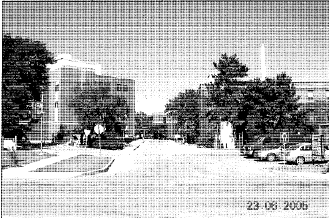
View west to Bruce Building with Wilcox Building (left) and Central Building (right).
