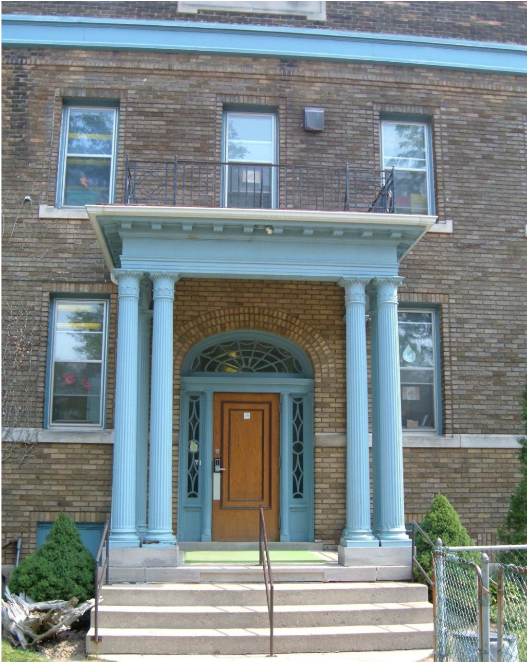
Figure 14: A closer view of the entrance portico, from 2007. The entrance features a decorative transom window, sidelights and brick voussoir. The portico includes detailed columns along with simple bracketing and cornice (City of Hamilton Archives).
