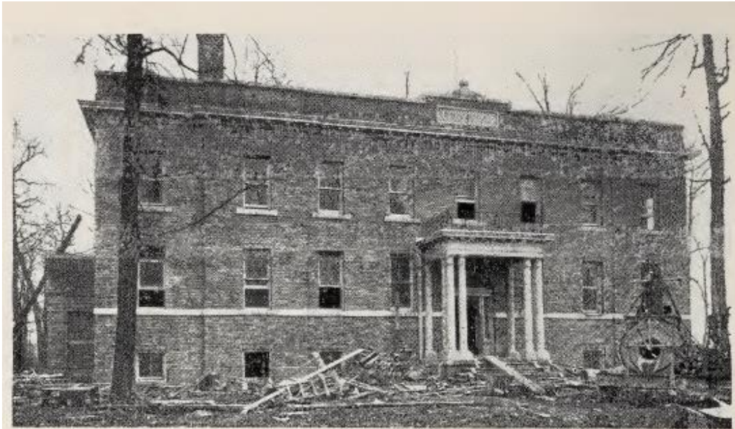
View of the New Nurses Home nearing completion, the gift of Mr W. D. Long and Mrs. George H. Bisby for which they contributed $75,000. This is a fine fire-proof structure and on account of the high cost of building Mrs. Bisby later contributed an additional $10,000.
