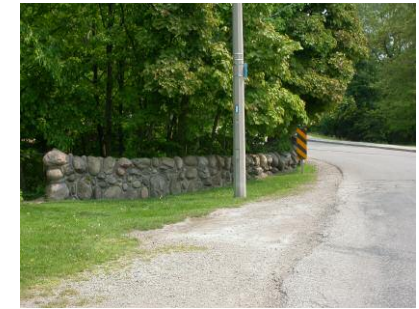
▲ Stone wall and pillar at vehicular bridge
