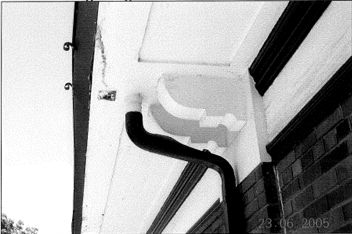
Paired wood brackets support the upper verandah.
