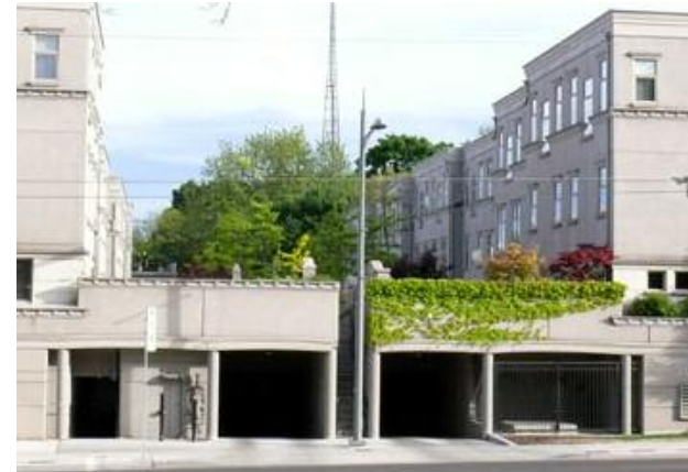
▲ Parking garages are concealed from view of the public street by a rooftop terrace in this townhouse development.
