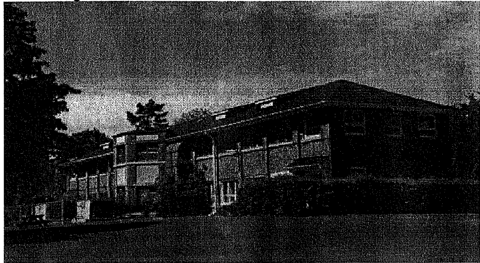
View of east (front) elevation of the East Pavilion.
