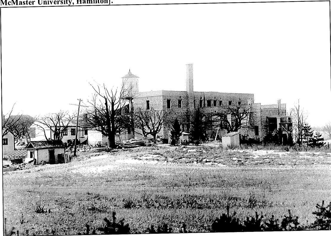
Bruce Building, northeast corner during construction. Circa 1920. [Health Sciences Library, McMaster University, Hamilton].
