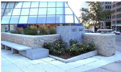
▲ This architectural planter wall creatively screens the building venting system from view.
