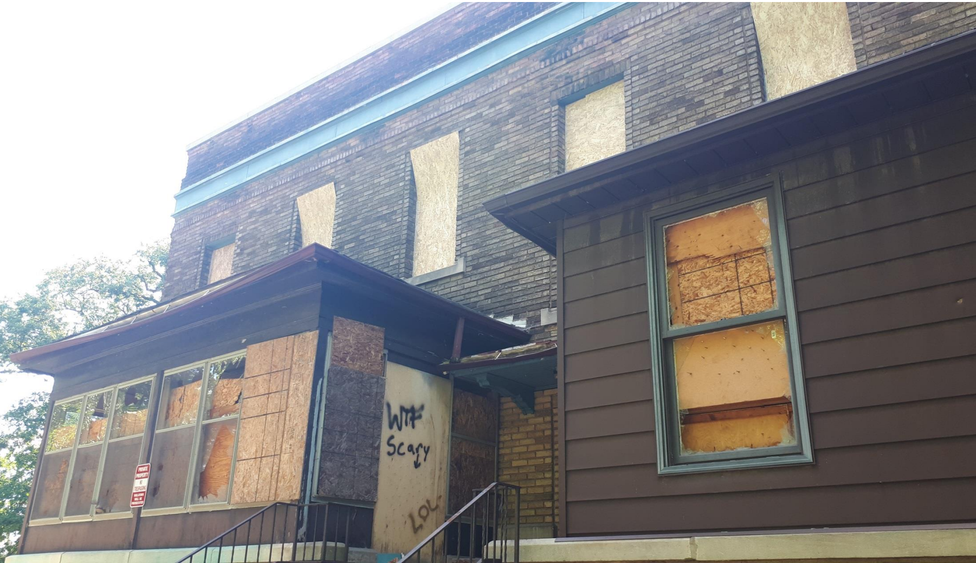
Photograph of rear elevation with small vestibule additions (Parsons, 2018).
