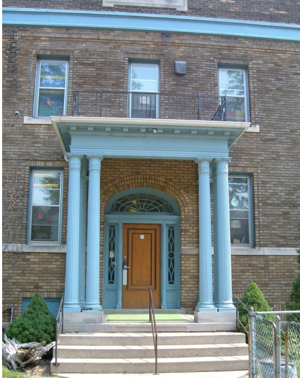
A closer view of the entrance with portico, decorative transom window, sidelights, and brick voussoir (City of Hamilton Archives, 2007).
