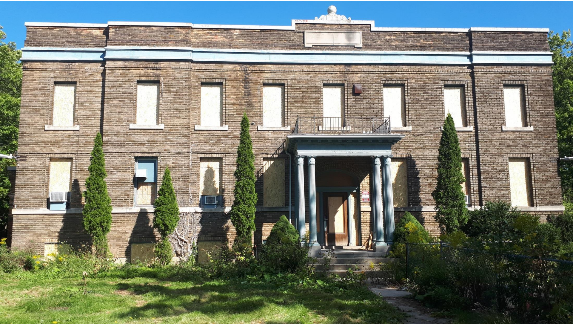
Front façade (Parsons, 2018)
