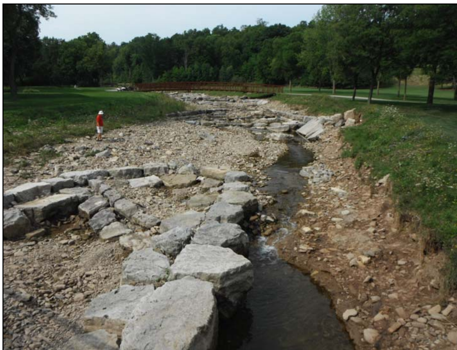
Figure 5. Red Hill Creek post-flood event on August 9 th , 2012 showing extensive scouring of the channel bank and loss of vegetation in King's Forest Golf Course.
