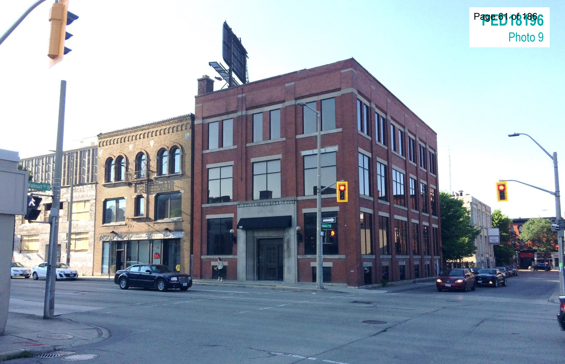
Existing development at 145 and 147 Main Street East located to the north west of the subject property, as seen from Main Street East looking north west
