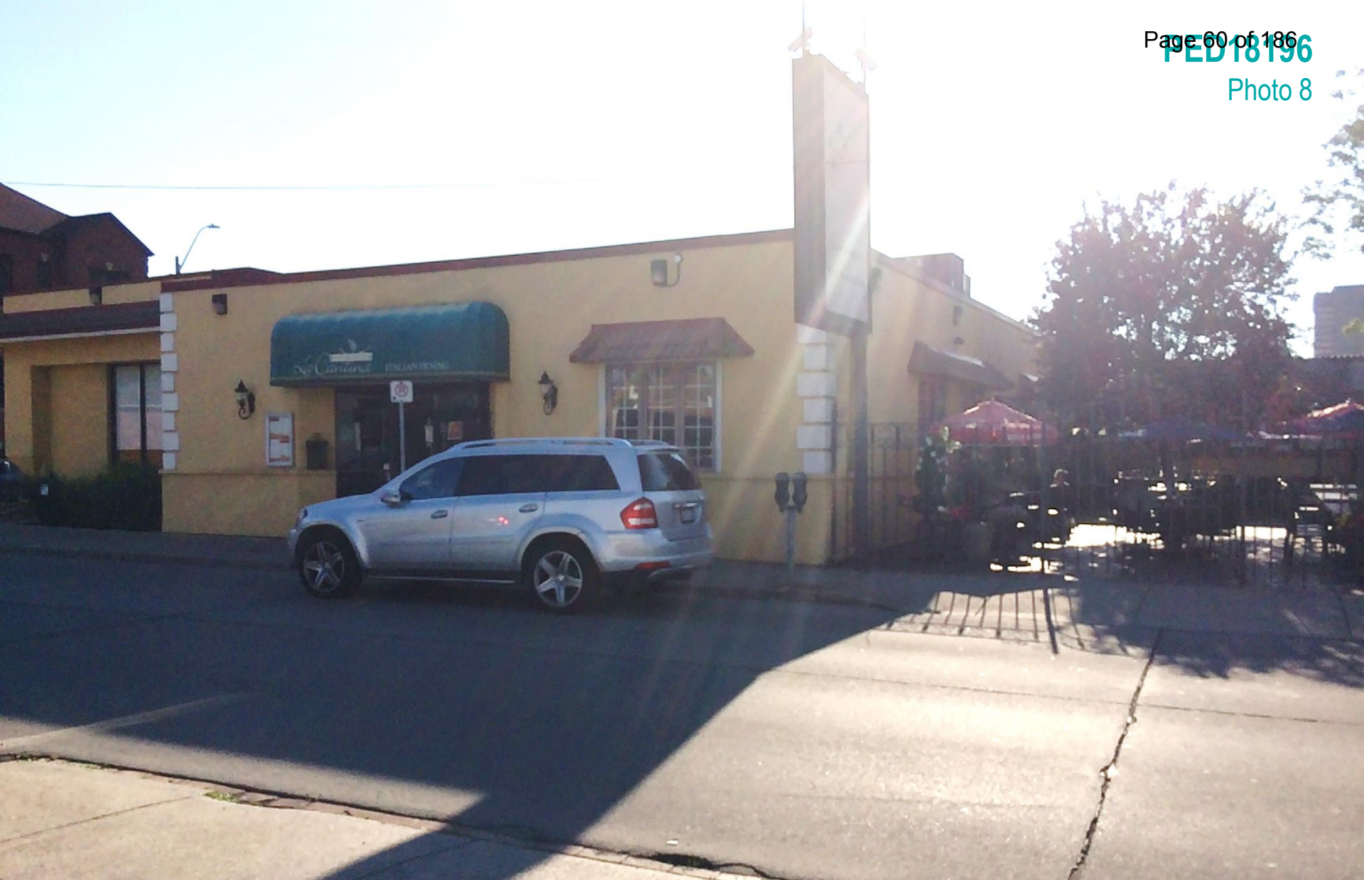
Existing development at 60 Walnut Street South, as seen from Walnut Street South looking west
