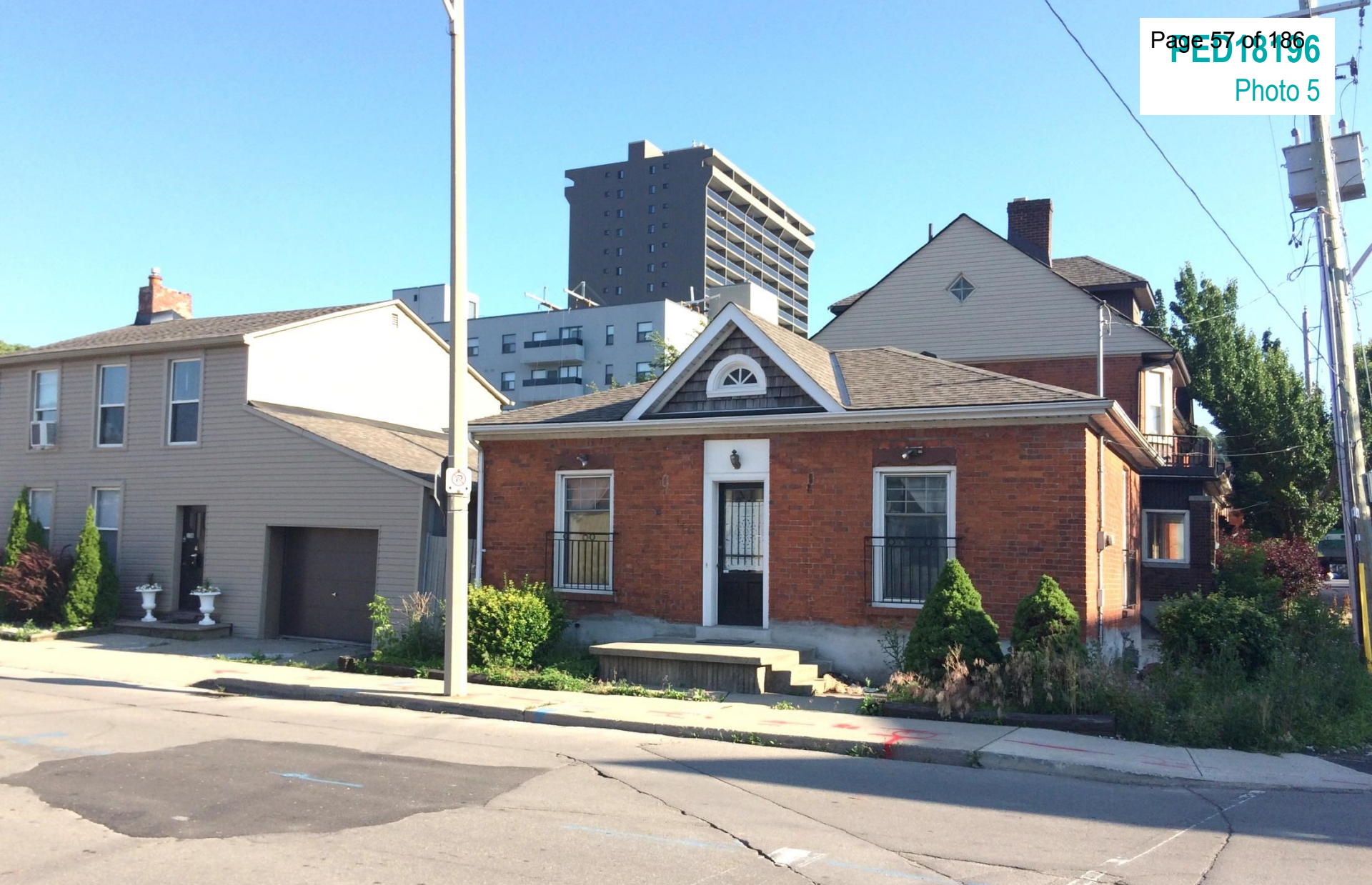
Existing development at 154 and 158 Jackson Street East located to the south of the Subject property, as seen from Jackson Street East looking south west
