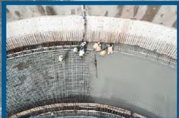
2092m 3 of concrete 1.3-1.4 metres thick
