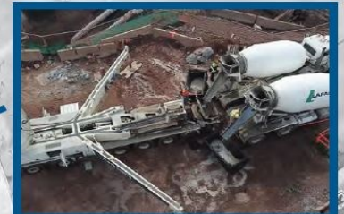
240 truckloads of concrete
