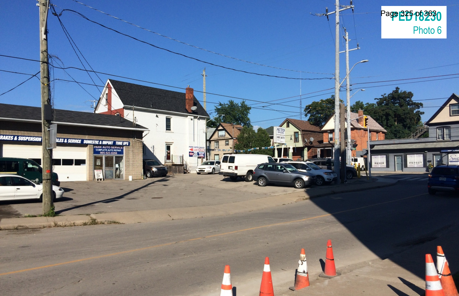
216 Dundurn Street South located to the north of the Subject Property, as seen from Chatham Street looking north east
