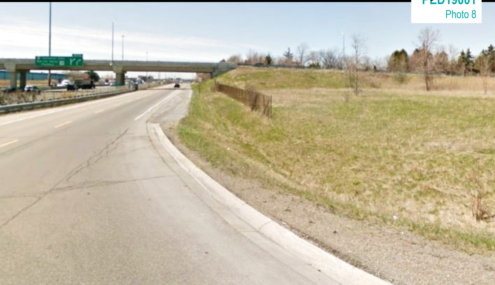
North Service Road looking west
