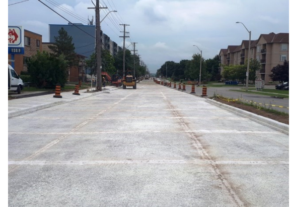
Mohawk Road Resurfacing
