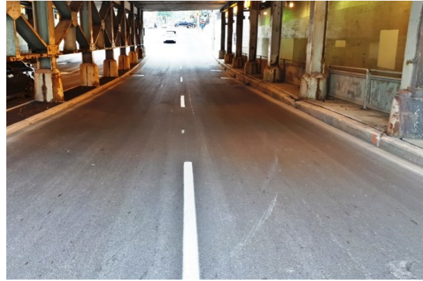
James St S Resurfacing
