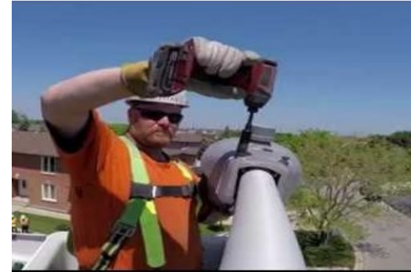
Street lighting upgrades
