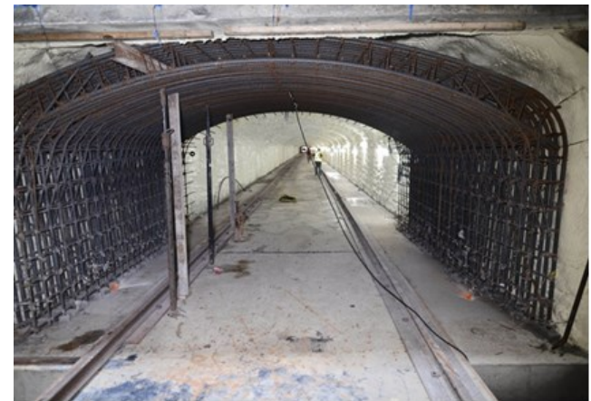
Mountain Trunk Storm Sewer Rehabilitation
