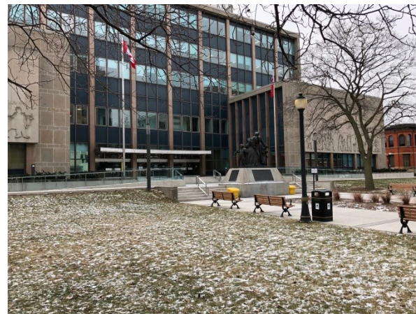
AFTER: POA Building
