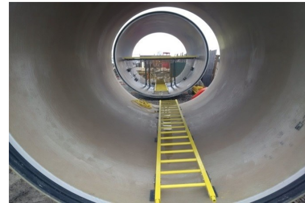
Centennial Sewer Trunk
