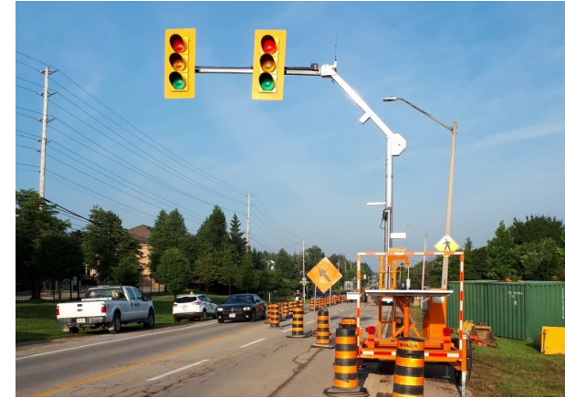
Governor's Road Reconstruction
