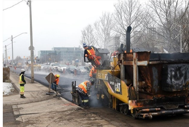
Main Street West Resurfacing
