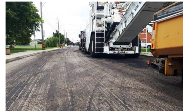
$12 million in road resurfacing “shave and paves”
