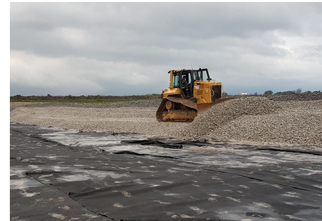
Glanbrook Landfill Stage 3
