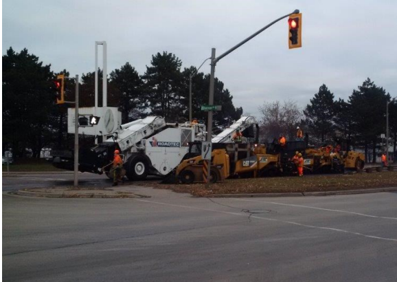
Burlington Street Resurfacing
