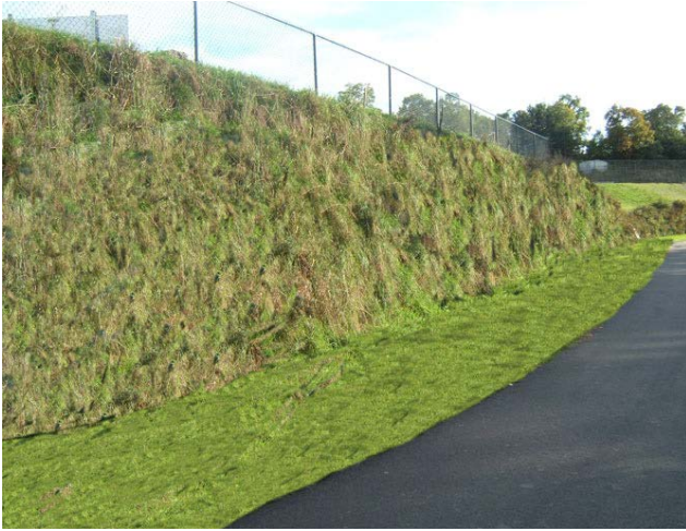
Figure 6.19 Mechanically Stabilized Earth Berm (Strata System)
