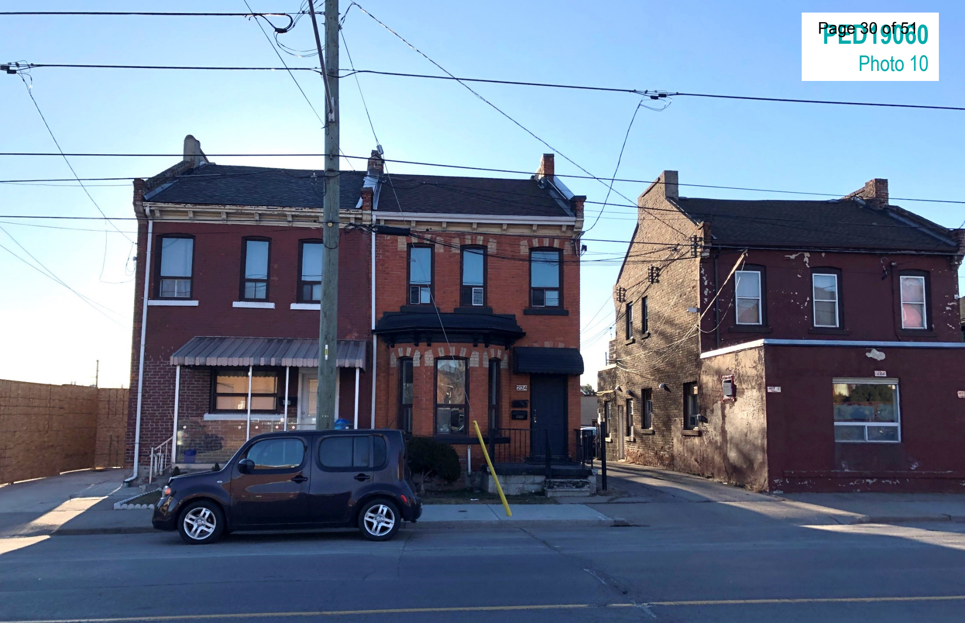
Lands abutting the John Street North frontage
