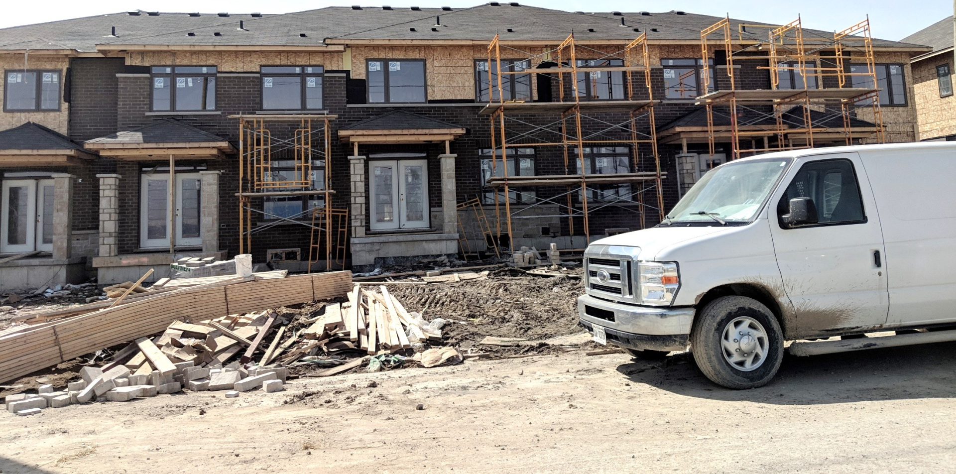
Greenwich Avenue dwellings under construction
