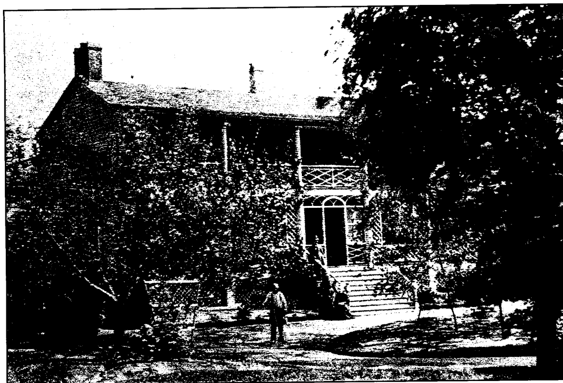
Crooks' house – demolished 1884
