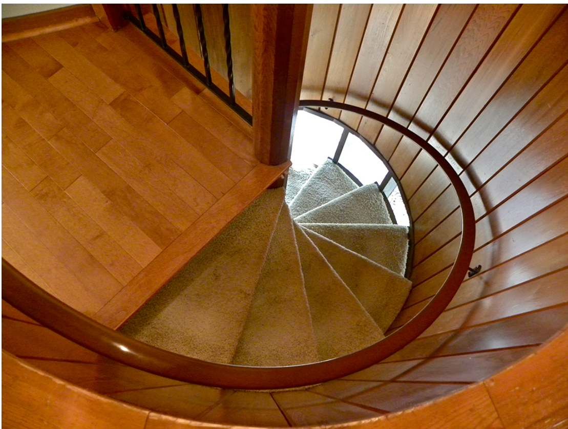
Photo 7: View looking down the spiral staircase to its glass enclosure on the lower level. Carpeting was likely a later addition to the metal stairs. (Graham Crawford, 2011)
