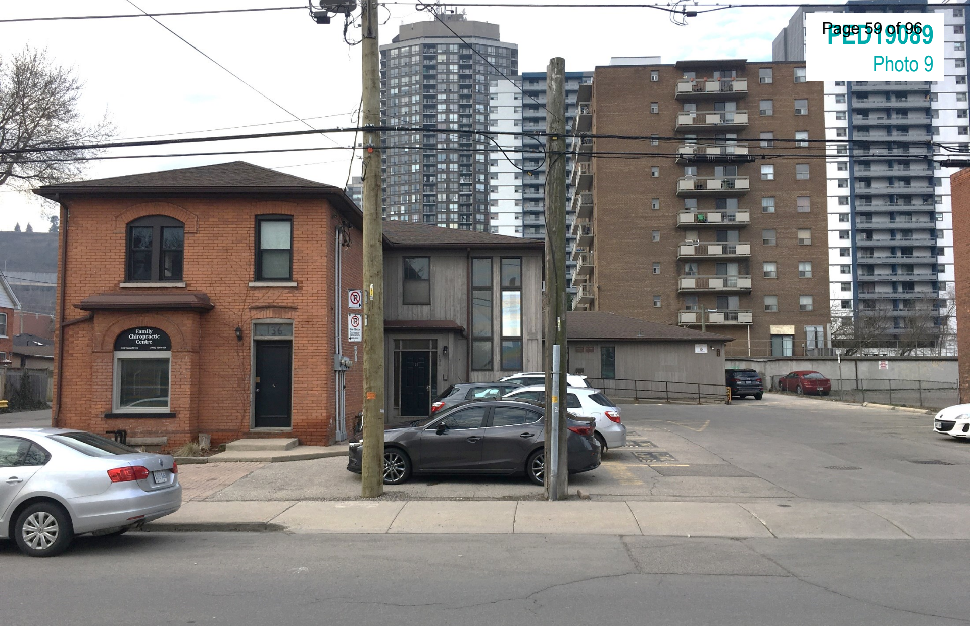
Existing development located to the south of the Subject Lands, as seen from Young Street looking south.
