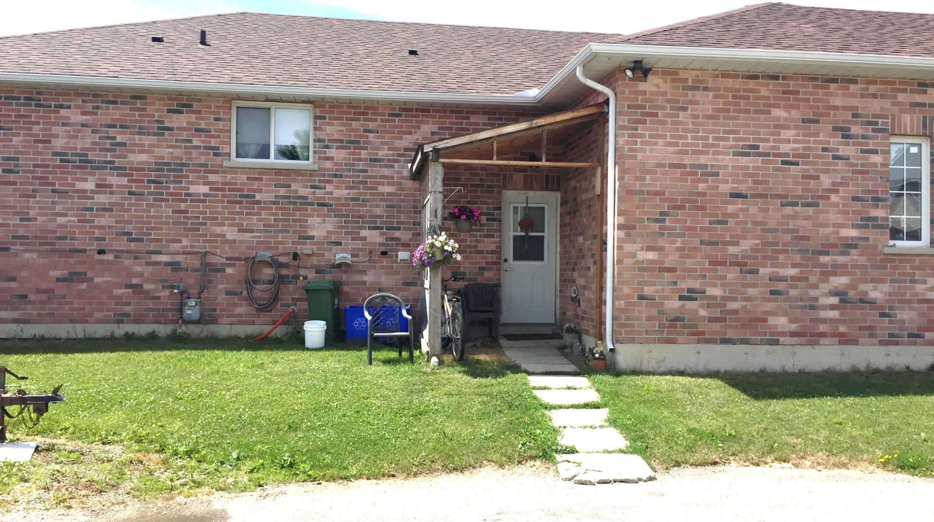
Single detached dwelling adjacent to Marion Street stub
