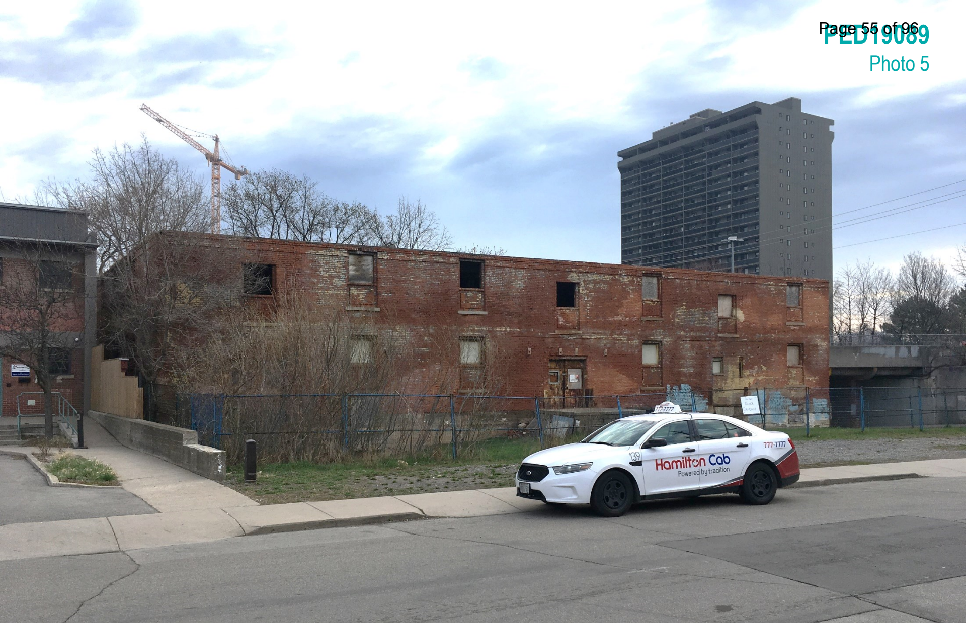
Existing development located to the northeast of the Subject Lands, as seen from Augusta Street looking northeast.
