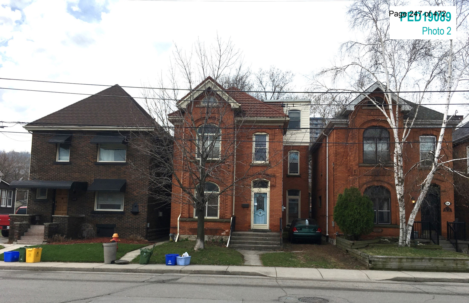
Existing development located to the west of the Subject Lands, as seen from Augusta Street looking south.
