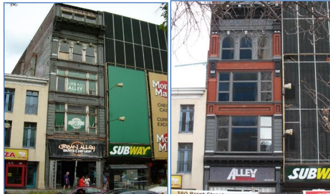
11 King Street East, Hamilton (before and after)
