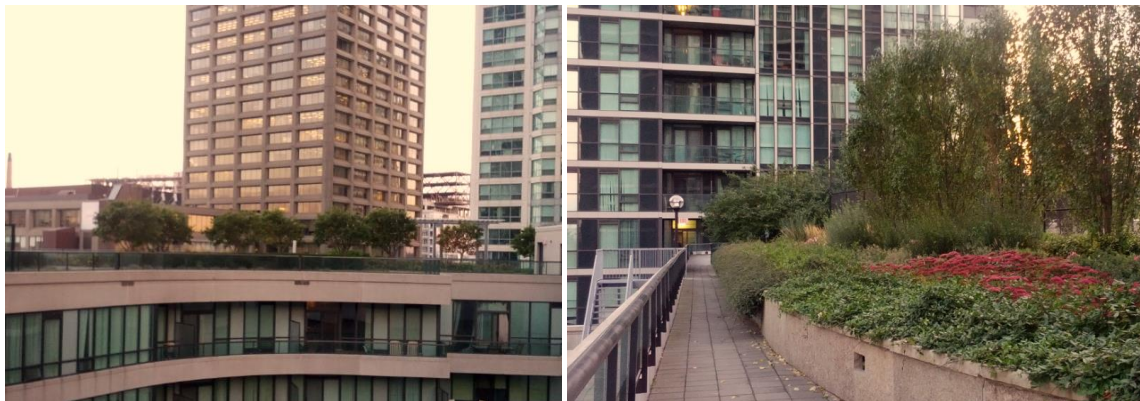
b) Dense Landscaping Canopies – The strong winds expected to accelerate around the tower corners could be dispersed by wraparound overhead canopies.
