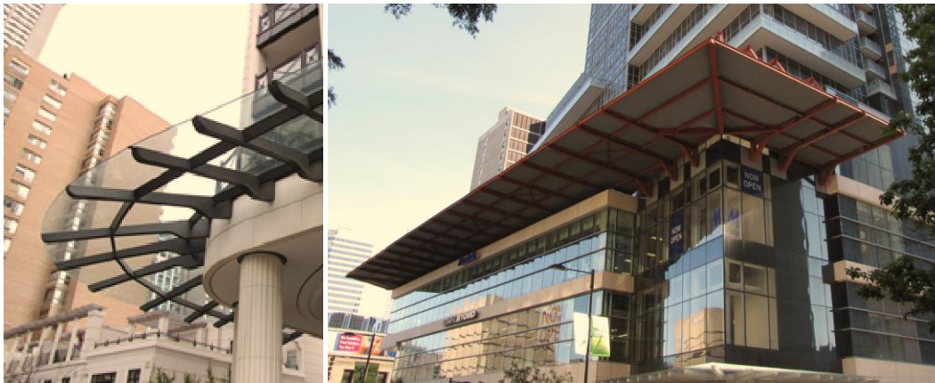
a) Wraparound Overhead Canopies – The strong winds expected to accelerate around the tower corners could be dispersed by wraparound overhead canopies.
