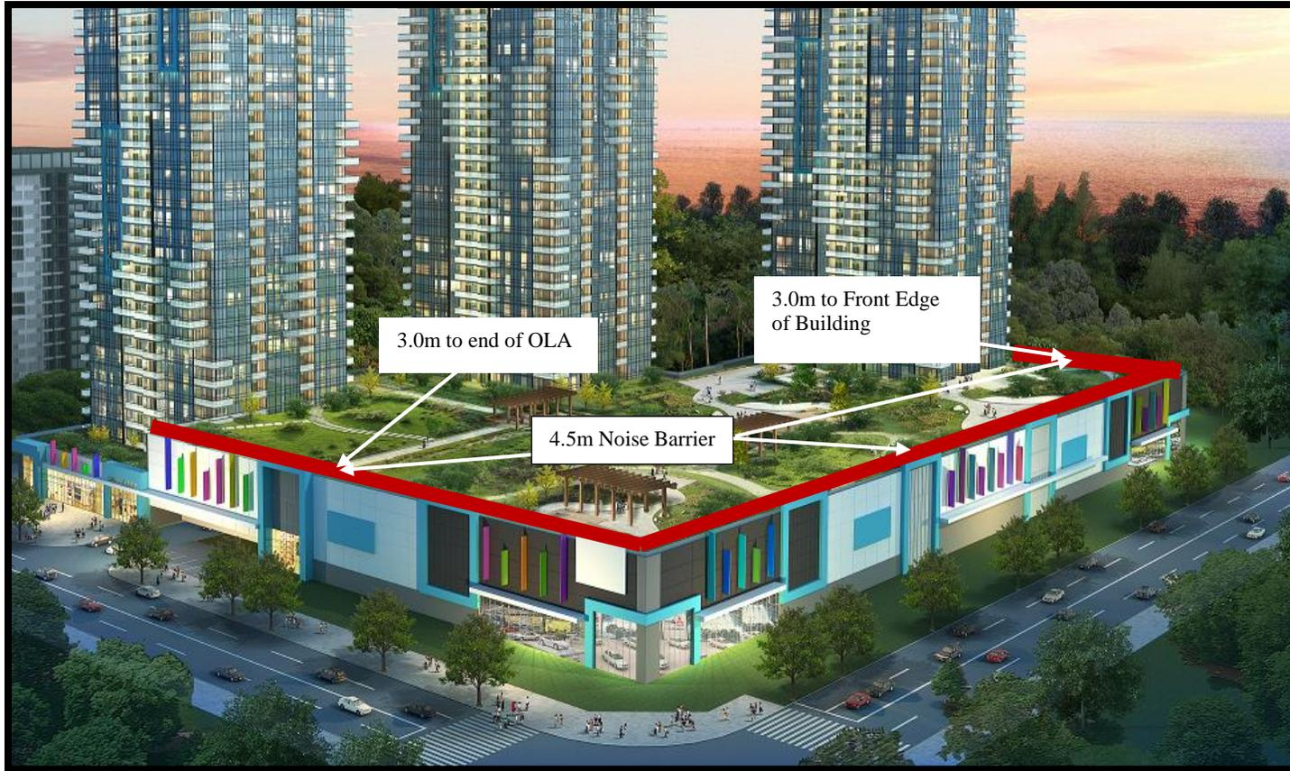
Note: Red line represents the 4.5m height noise barrier that will be constructed of concrete extending from the parapet walls to the south, east, and west. The east and west wing walls will be staged to a minimum 3.0m height wall and confirmed length once final designs are completed.
