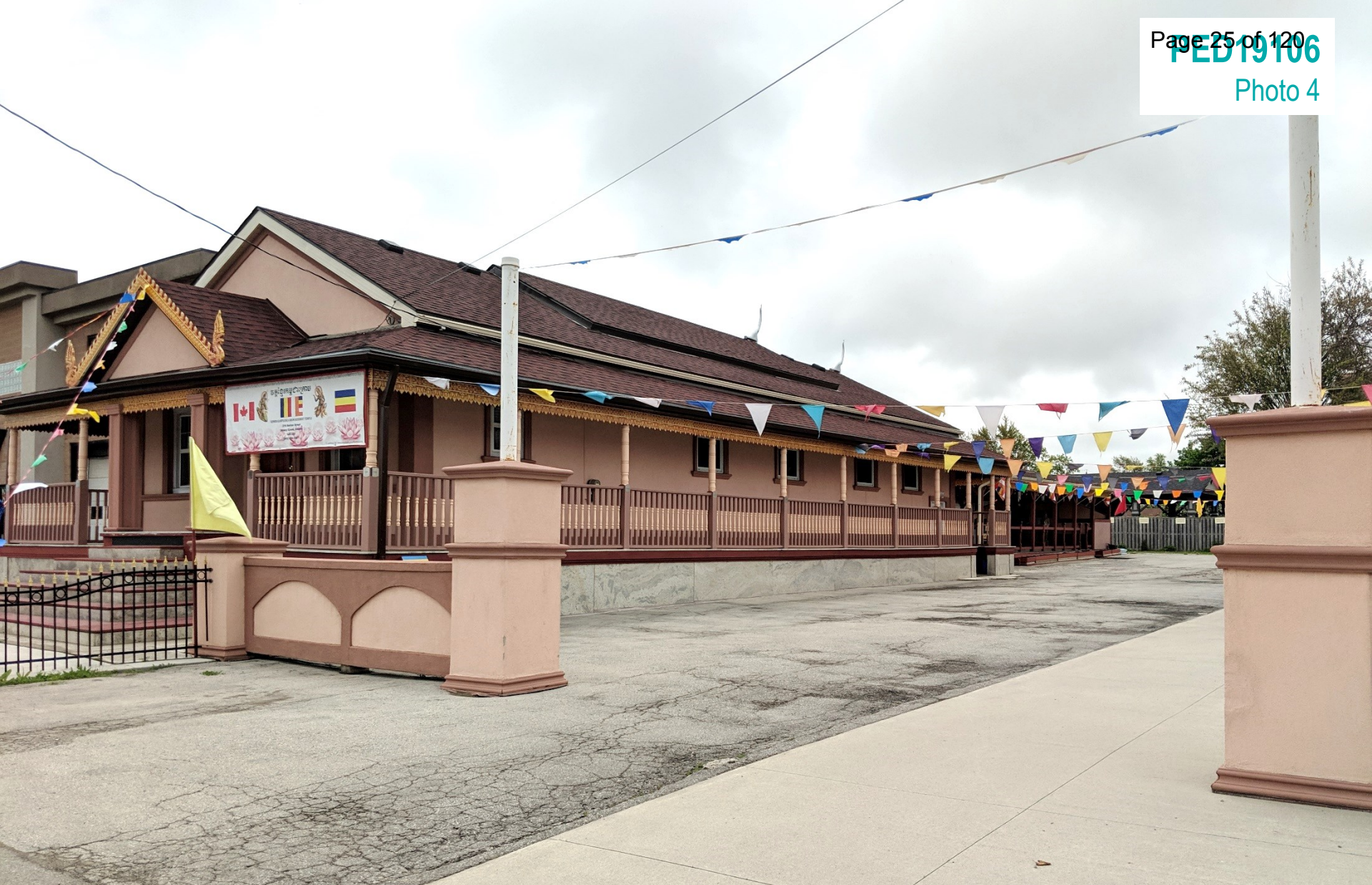
Parking area within Subject Lands.
