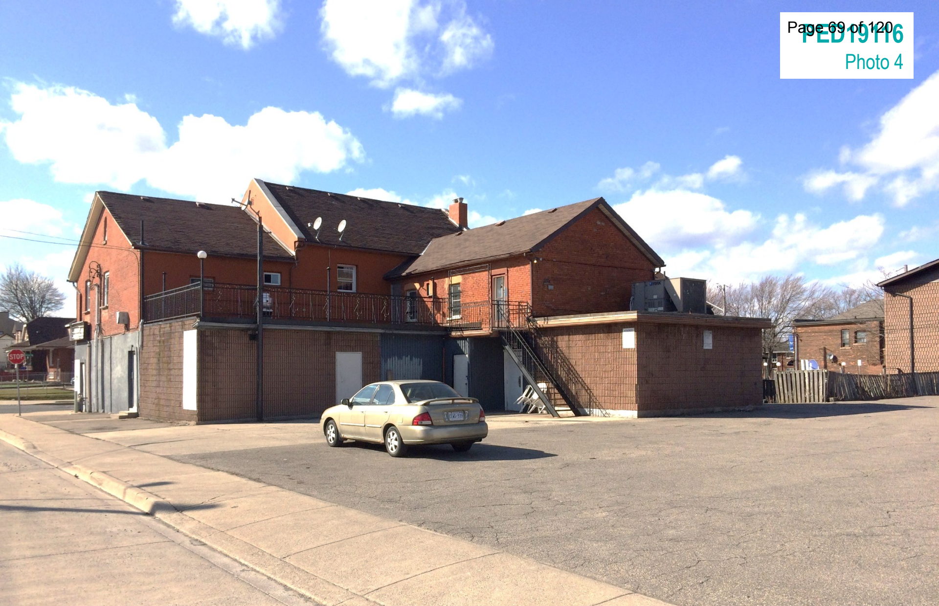
Photo of the rear of the existing buildings on the Subject Lands, as seen from Ferrie Street East looking north west.
