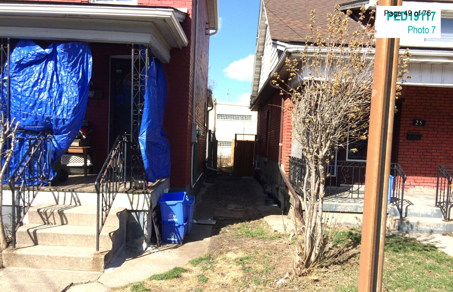
Edward Street frontage of the subject property, located between the properties at 23 and 25 Edward Street, as seen from Edward Street looking north
