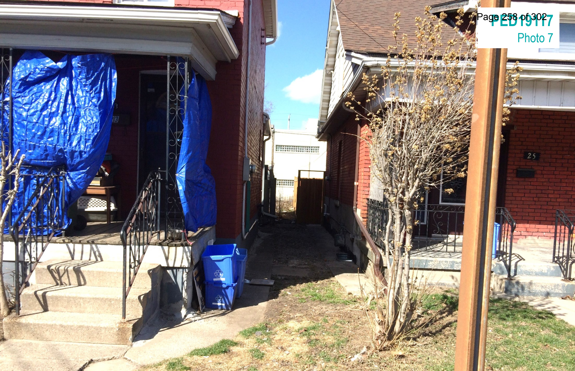
Edward Street frontage of the subject property, located between the properties at 23 and 25 Edward Street, as seen from Edward Street looking north
