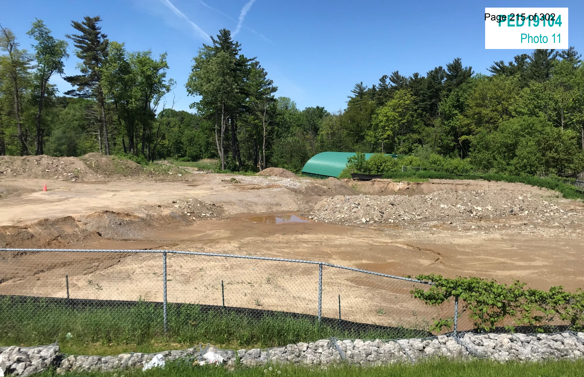
Looking over Vansickle Court at Subject Lands.
