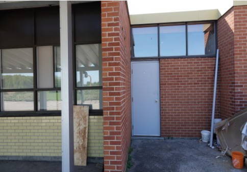
Ladies Wash room access from outside
