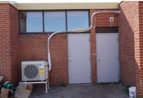
Gents Washroom access from outside
