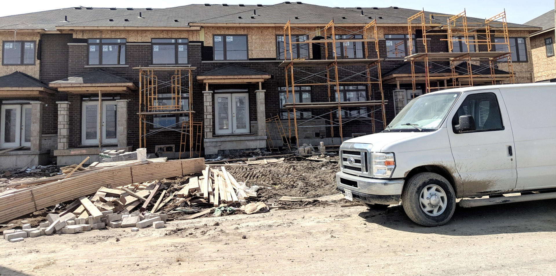
Greenwich Avenue dwellings under construction
