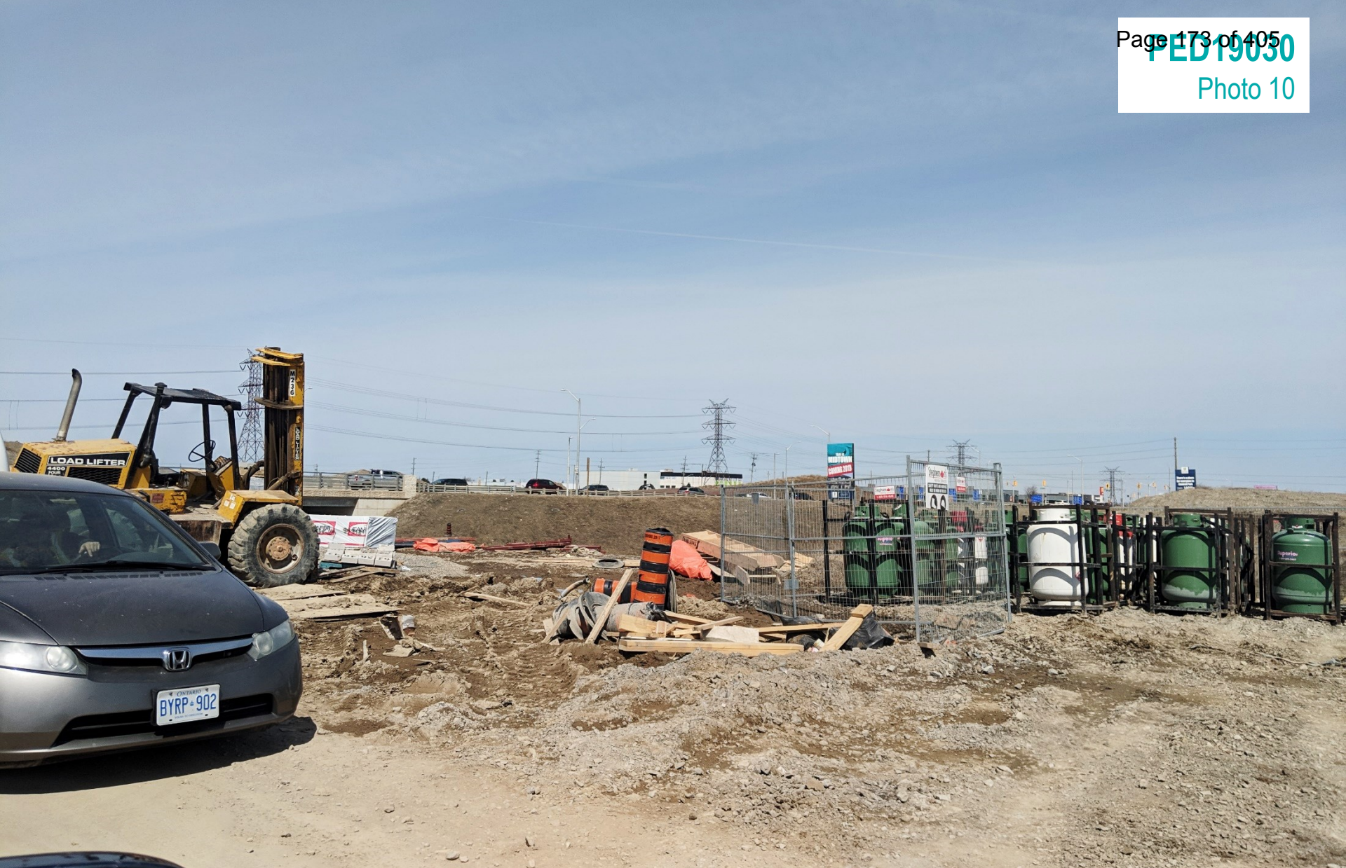
Phase 1 lands with open space block, looking west
