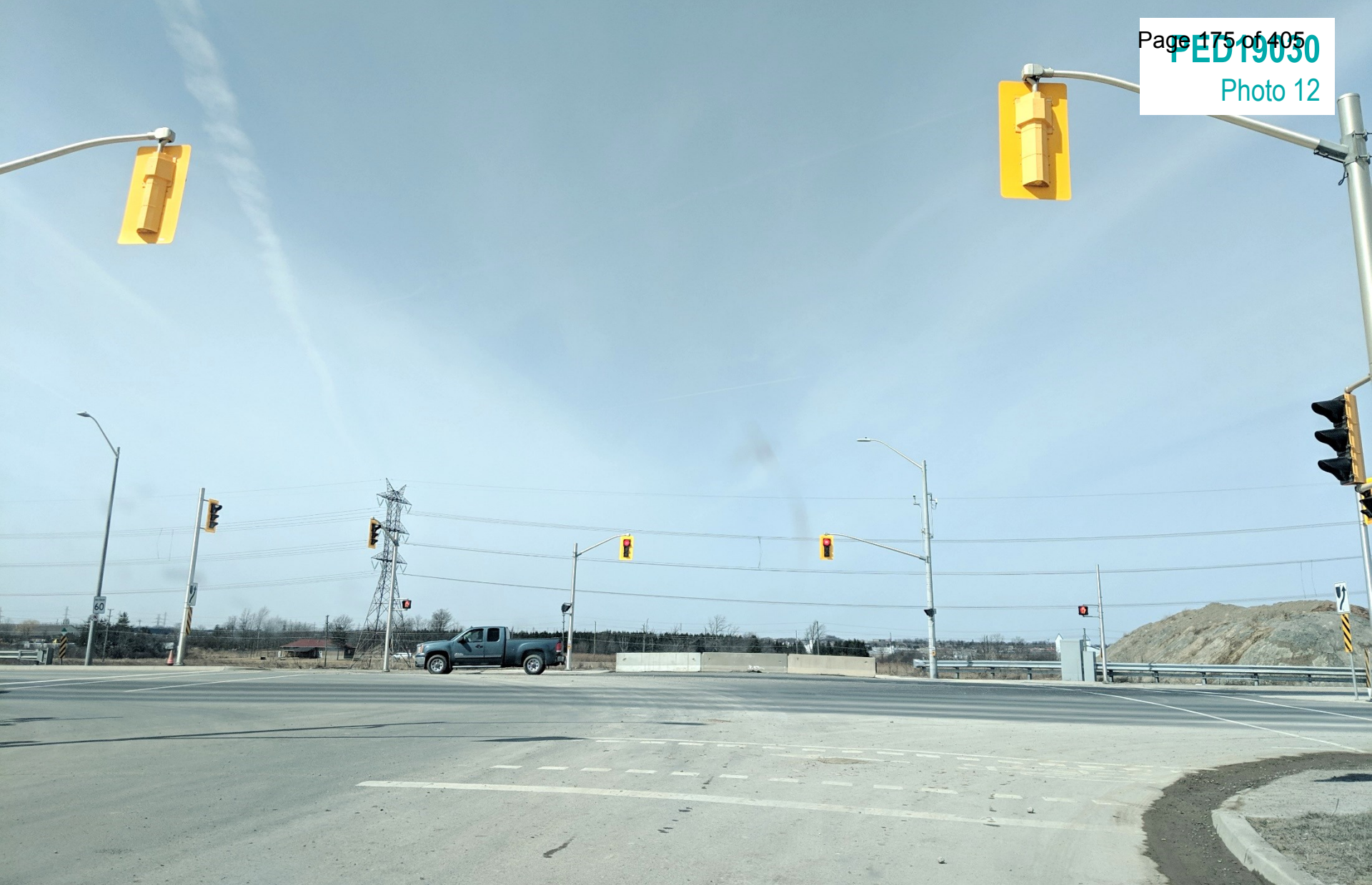
Upper Red Hill Parkway from Times Square (South of Block 97 of Subject lands)
