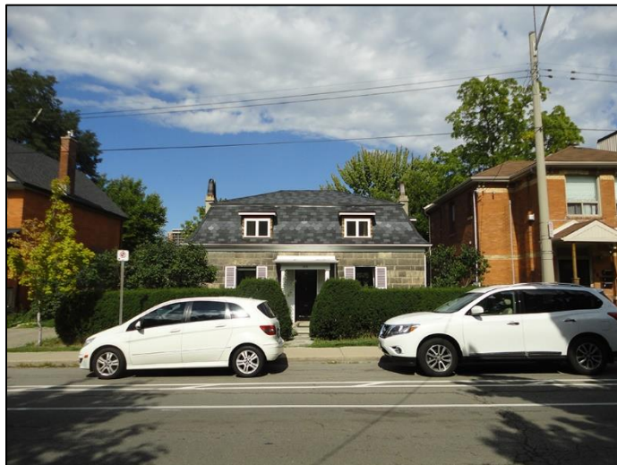
An example of a stone façade with brick on either side.
