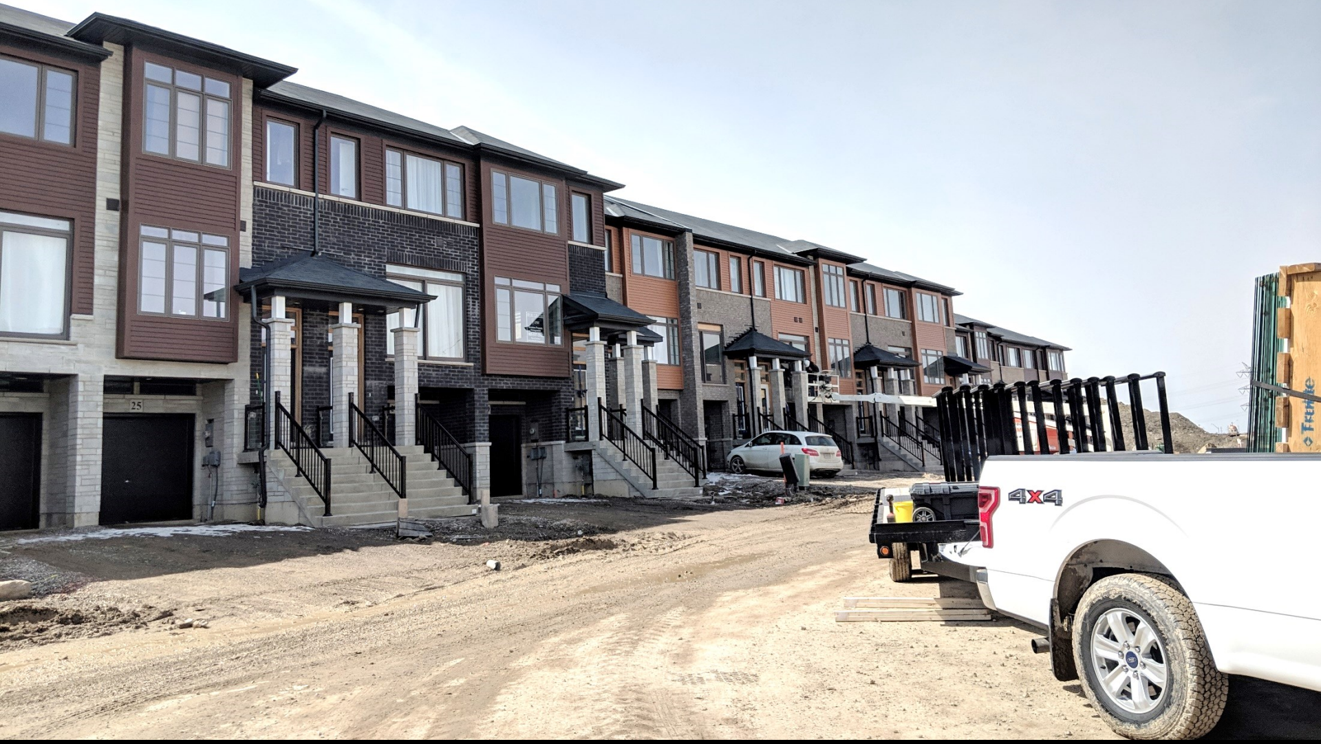
Residential uses under construction in Phase 2
