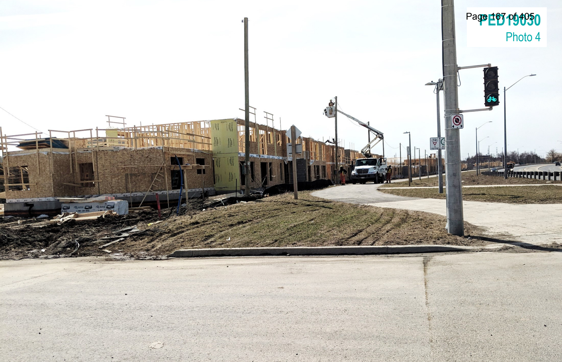
Phase 3 of Subject Lands, showing dwelling units under construction
