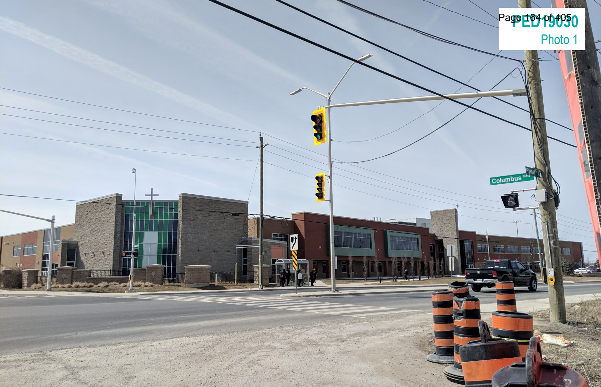
Existing secondary school south of Phase 3, Bishop Ryan Catholic Secondary School
