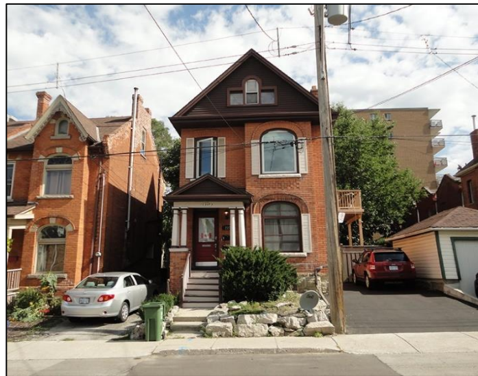
An example of a 2.5 storey house in Durand.
