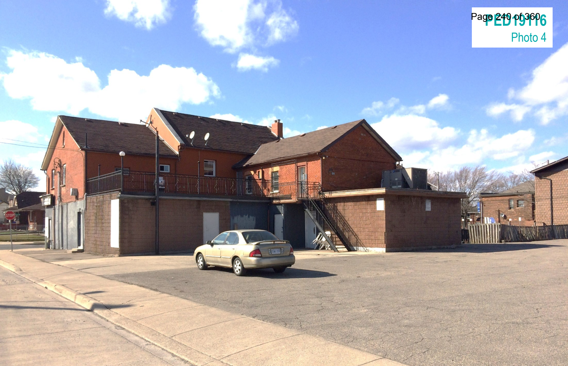
Photo of the rear of the existing buildings on the Subject Lands, as seen from Ferrie Street East looking north west.
