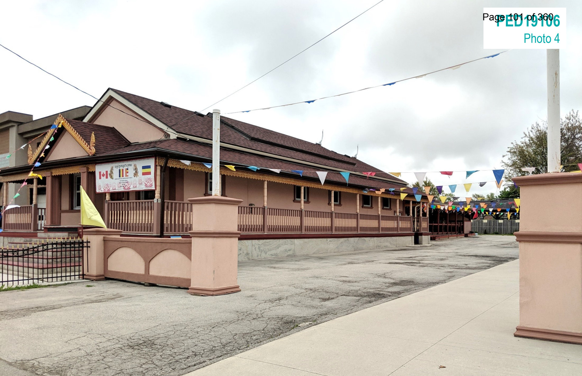
Parking area within Subject Lands.
