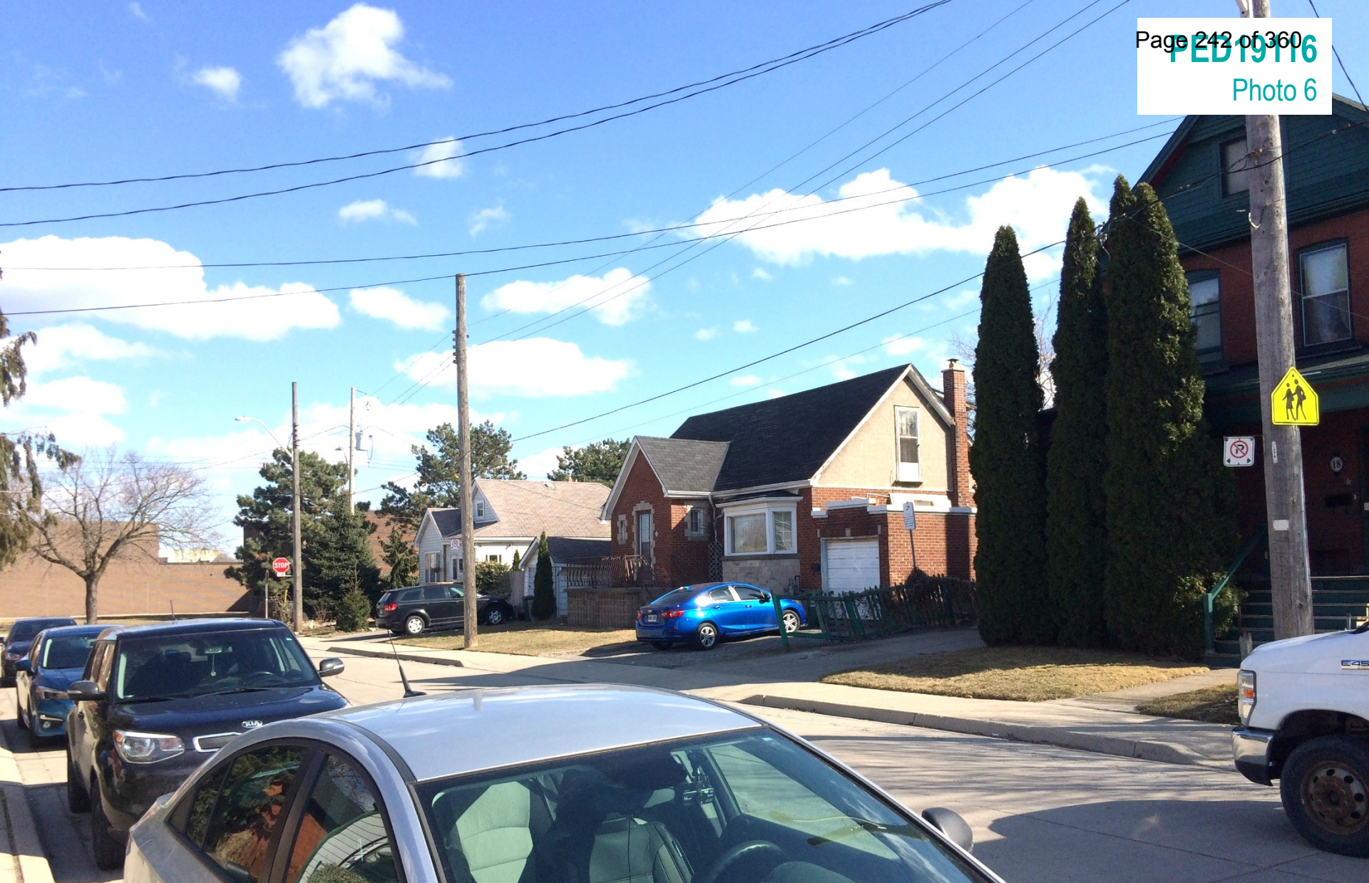
Photo of 18, 24, and 28 Ferrie Street East located to the south east of the Subject Lands, as seen from Ferrie Street East looking south east.
