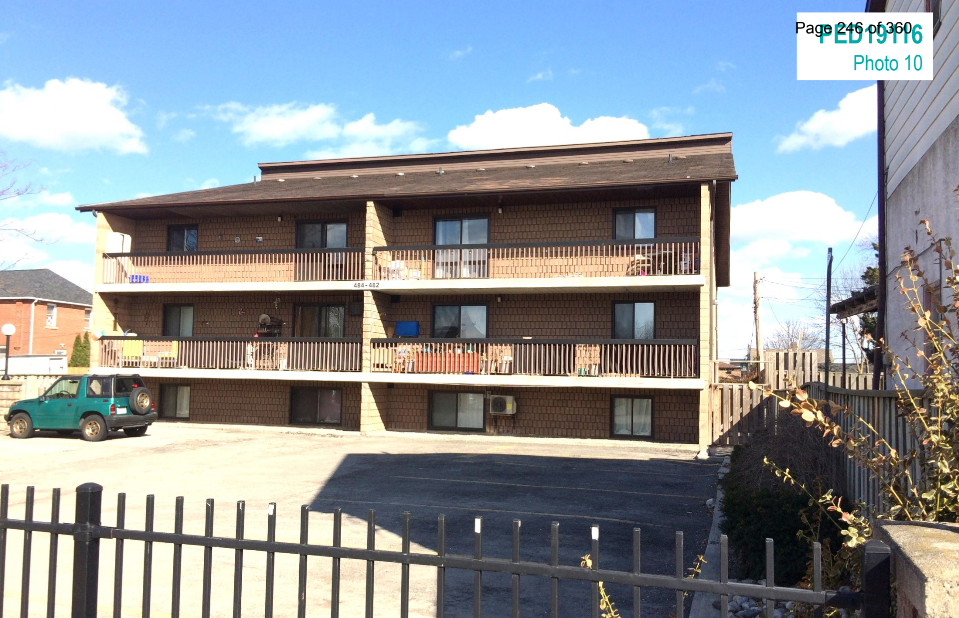
Photo of 482 James Street North located to the north of the Subject Lands, as seen from James Street North looking east.
