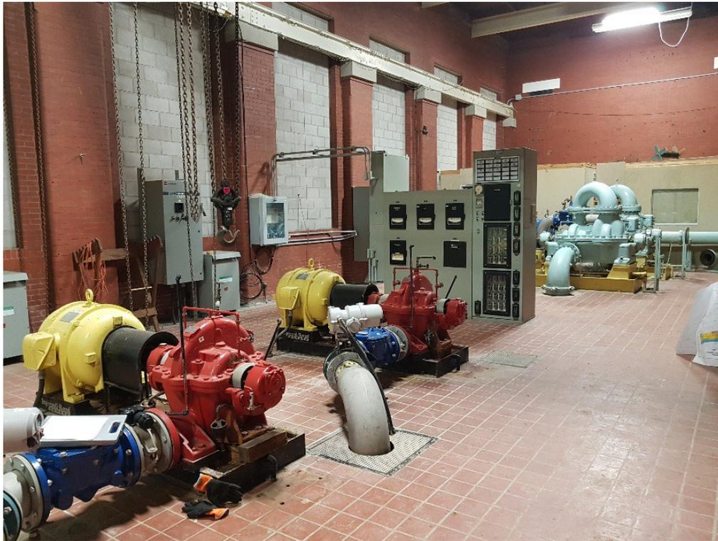
Figure 52: Mountain Level Pump Trains, High Lift Pump Trains, and Control Panel on the north portion of the floor.
