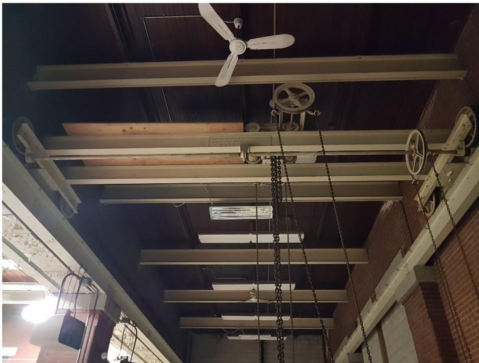
Figure 65: Chain pulley hoists suspended from lateral I-beams with Herbert Morris Chain and Hoist Company Ltd plaque.
