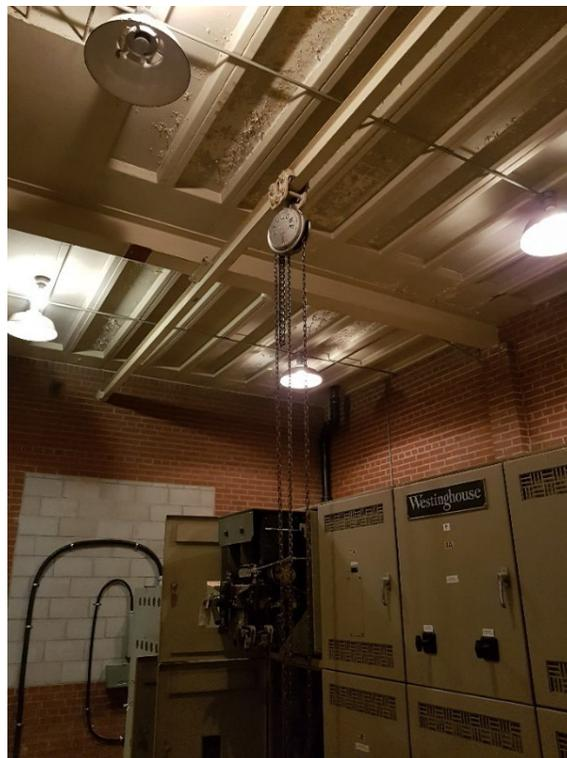
Figure 71: Fire proof ceiling with elliptical lights, and Columbus McKinnon Cyclone 1/2-ton beam trolley with hanging chain hoist.
