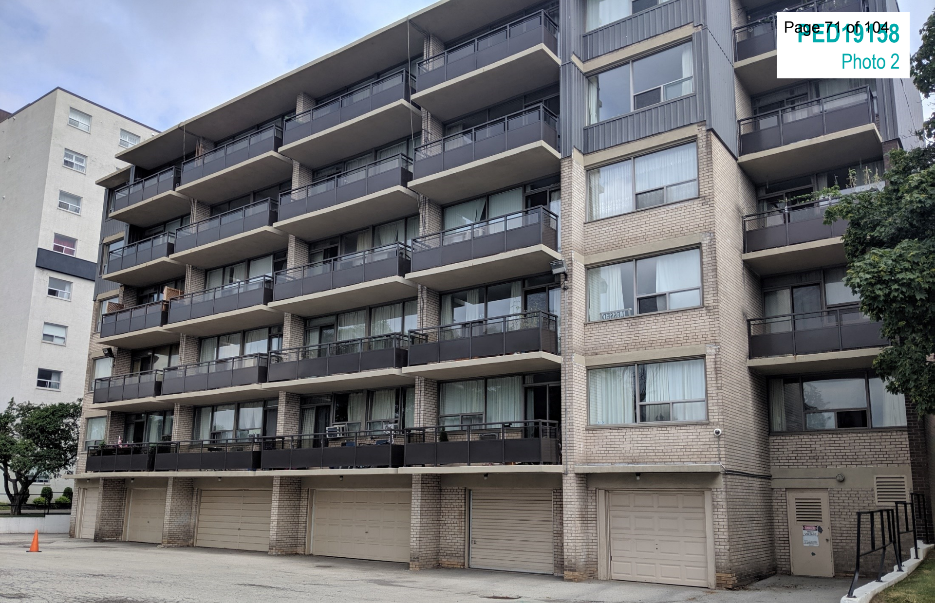
Existing multiple dwelling from the rear
