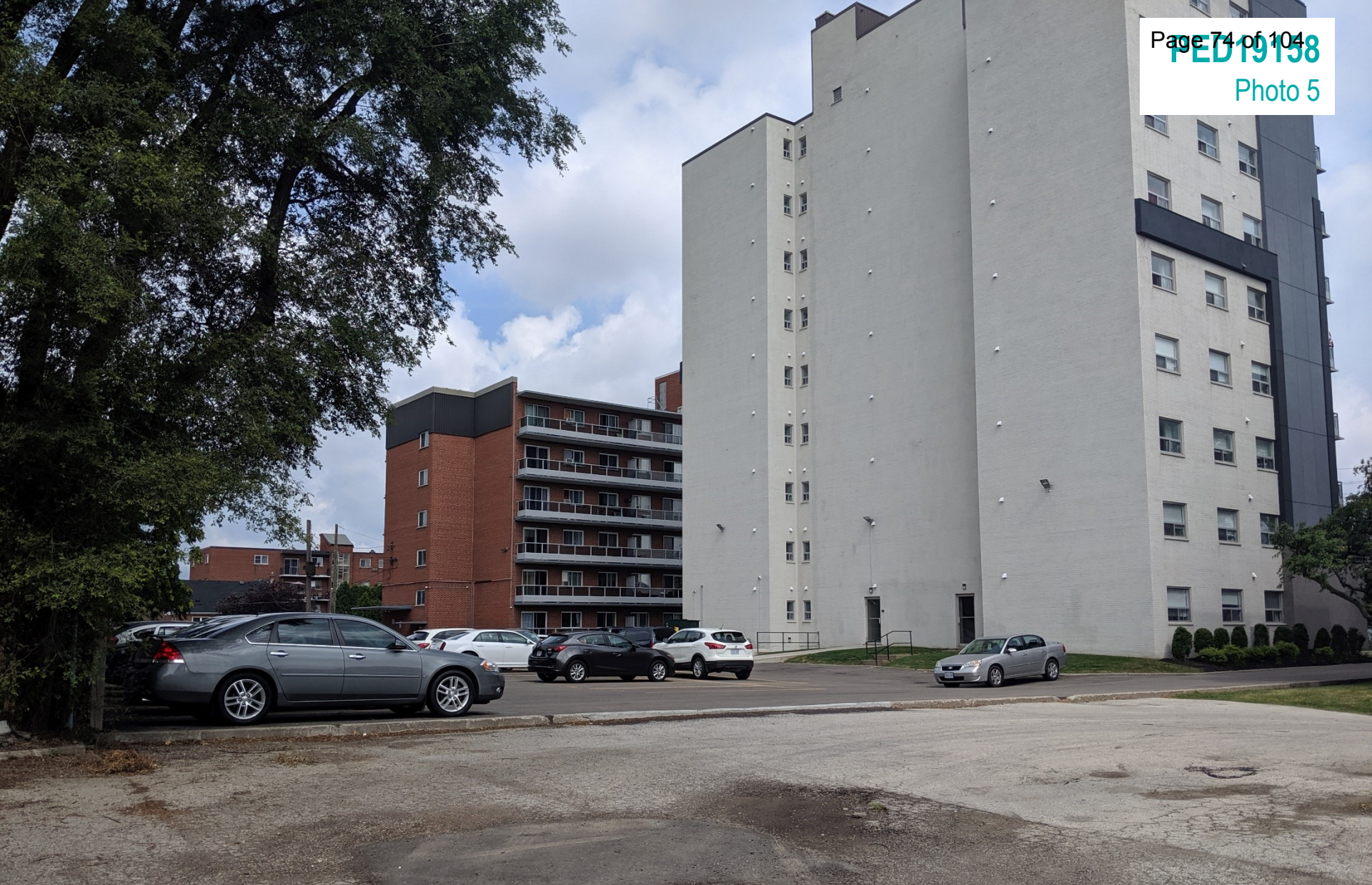
Existing rear parking lot and lands to the west
