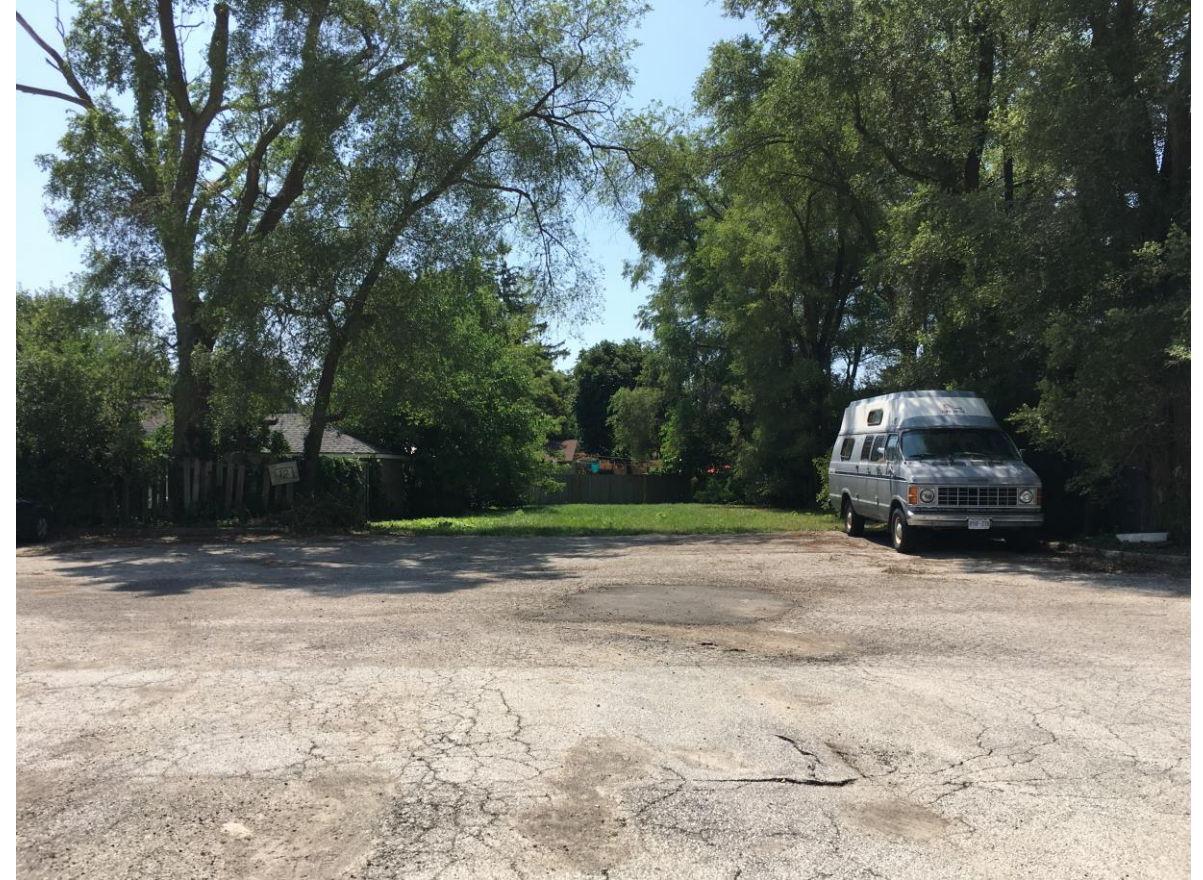
Image 3 - View of the proposed parking expansion area.
