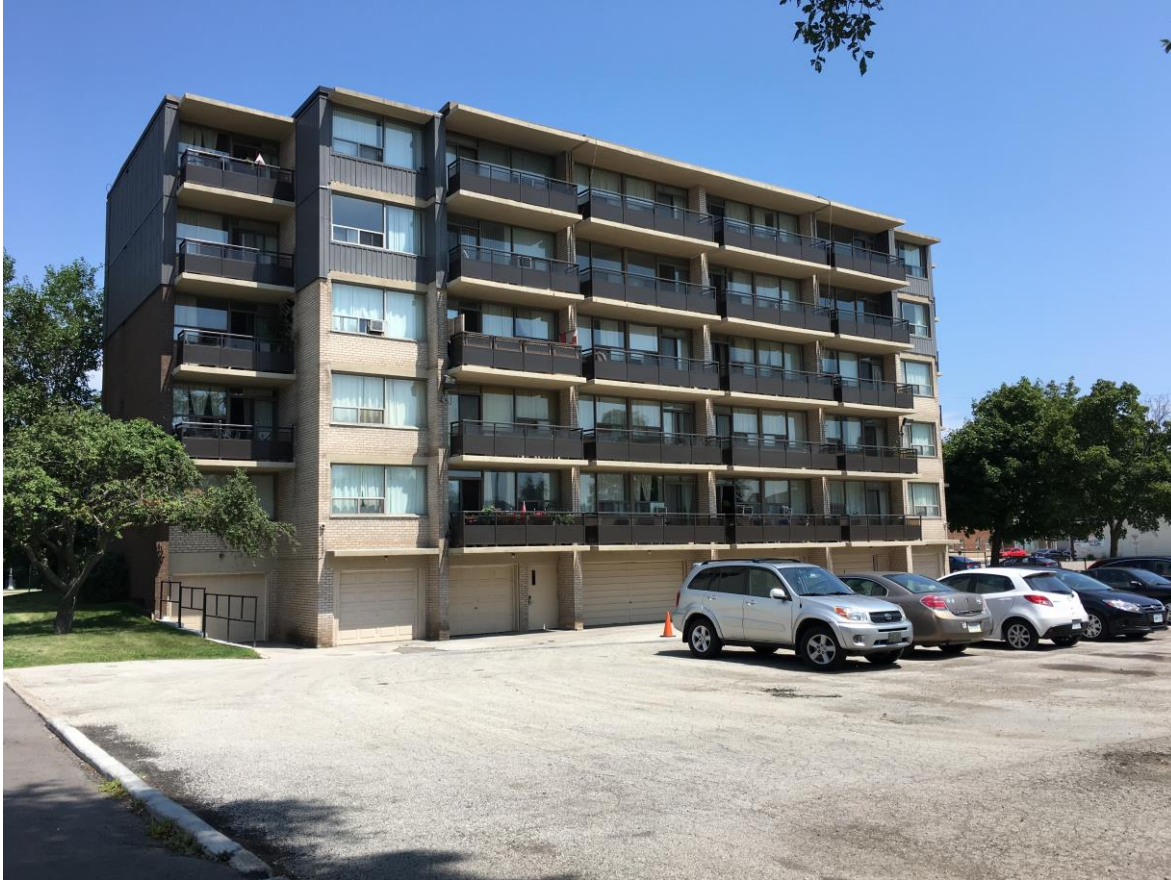
Image 2 - View of the existing apartment building from rear.
