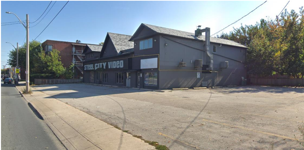
Existing Conditions – 1160 Main Street East, Hamilton
