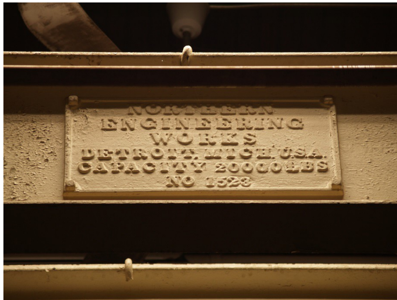
Figure 57: Northern Engineering Works plaque on a lateral I-beam.
