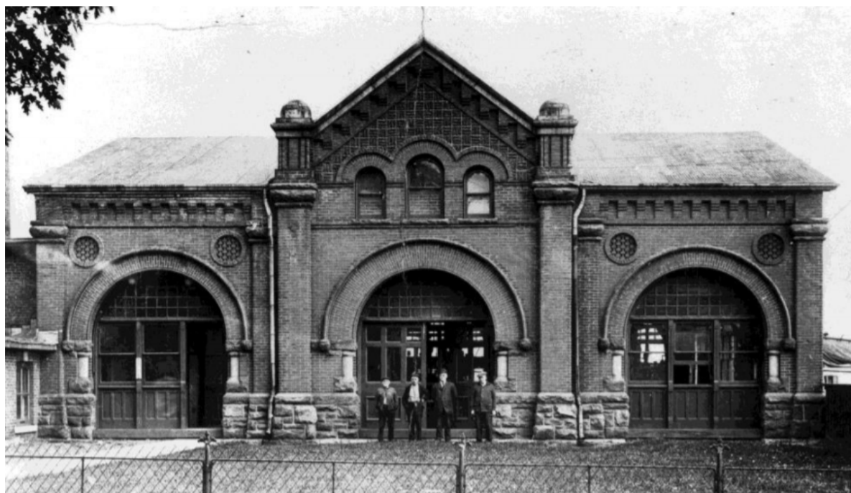
Figure 75: The 1889 Kingston Pumping Station, photographed in 1901 (Wevers 2013:2).
