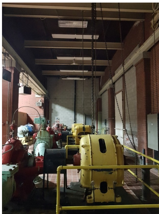
Figure 62: Interior of the 1929-30 Extension, facing east.
