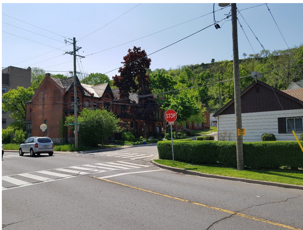
Figure 31: View facing southeast from the intersection with Charlton Avenue East. The pumping station is just visible behind the trees at centre, and the designated heritage properties of 221-227 Ferguson Avenue South are at left.
