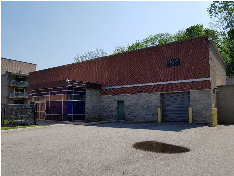
Figure 24: West facade of the 2012 New Ferguson Avenue Water Booster Pumping Station.
