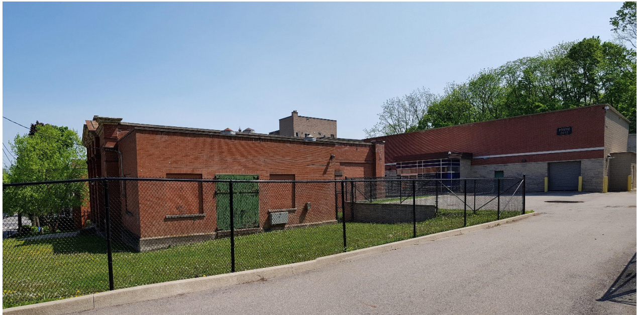
Figure 28: View facing northeast of the Ferguson Avenue Pumping Station (left) and new station (right) showing the irregular topography.
