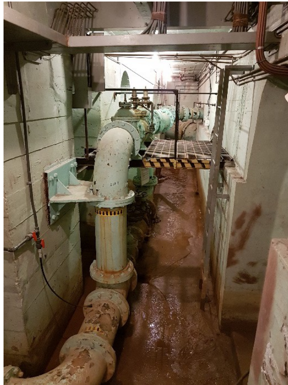
Figure 58: View facing east of the south basement passageway.
