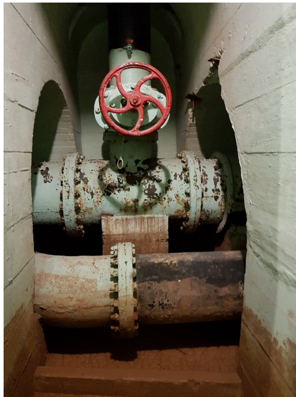
Figure 59: Arched cast-in-place concrete arches in the north portion of the basement.
