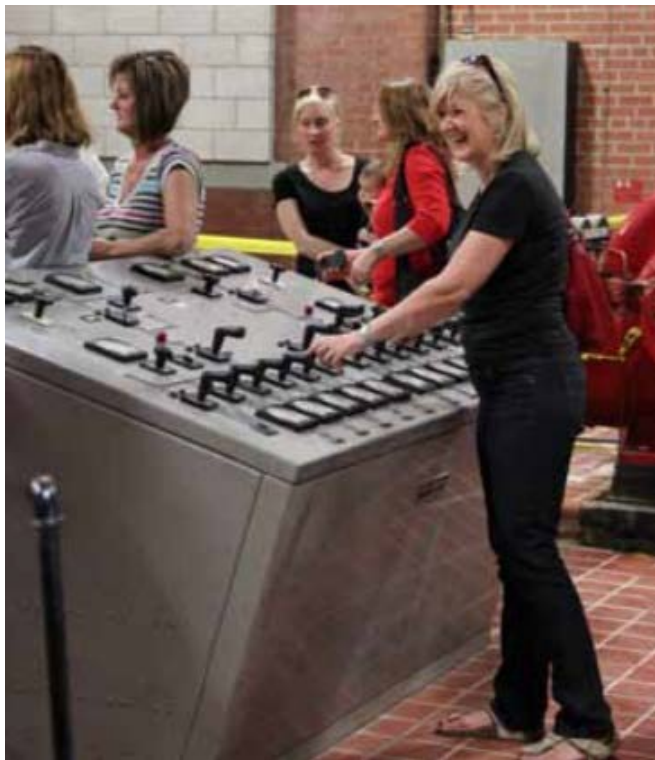
Figure 25: Visitors to the 2013 Doors Open at the Ferguson Avenue Pumping Station (City of Hamilton 2014:41).
