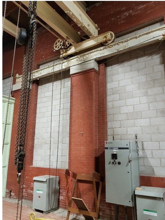
Figure 54: I-beams, engaged columns, and blind windows on the north wall interior.
