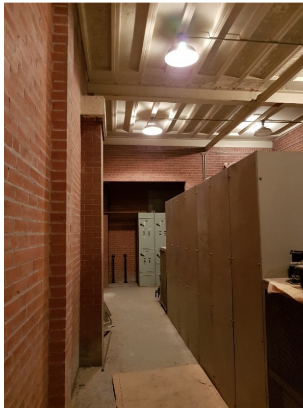
Figure 69: North interior portion of the 1955 Extension facing east.
