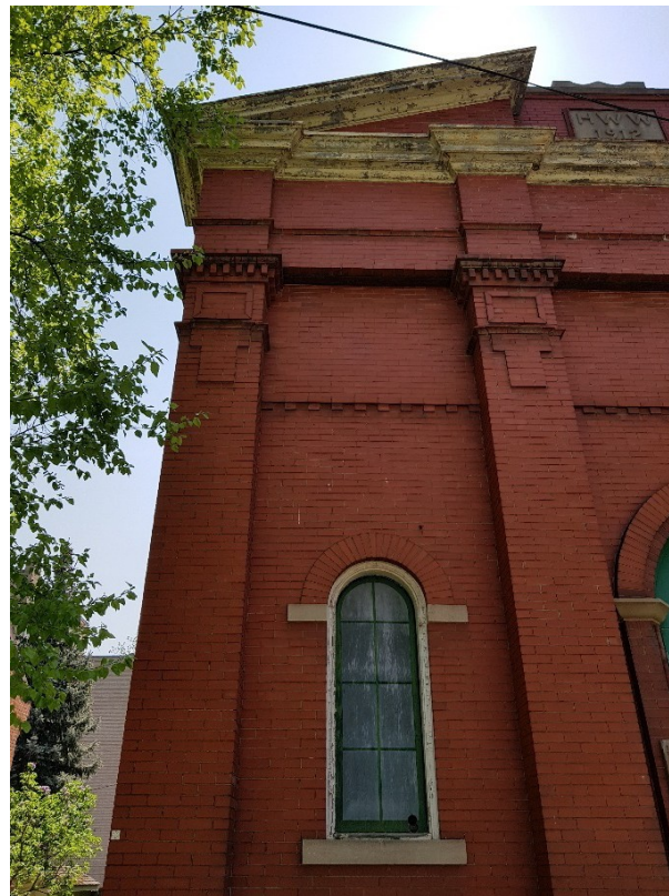
Figure 46: Denticulated string course, pilaster capitals, and entablature above the north bay of the west façade.
