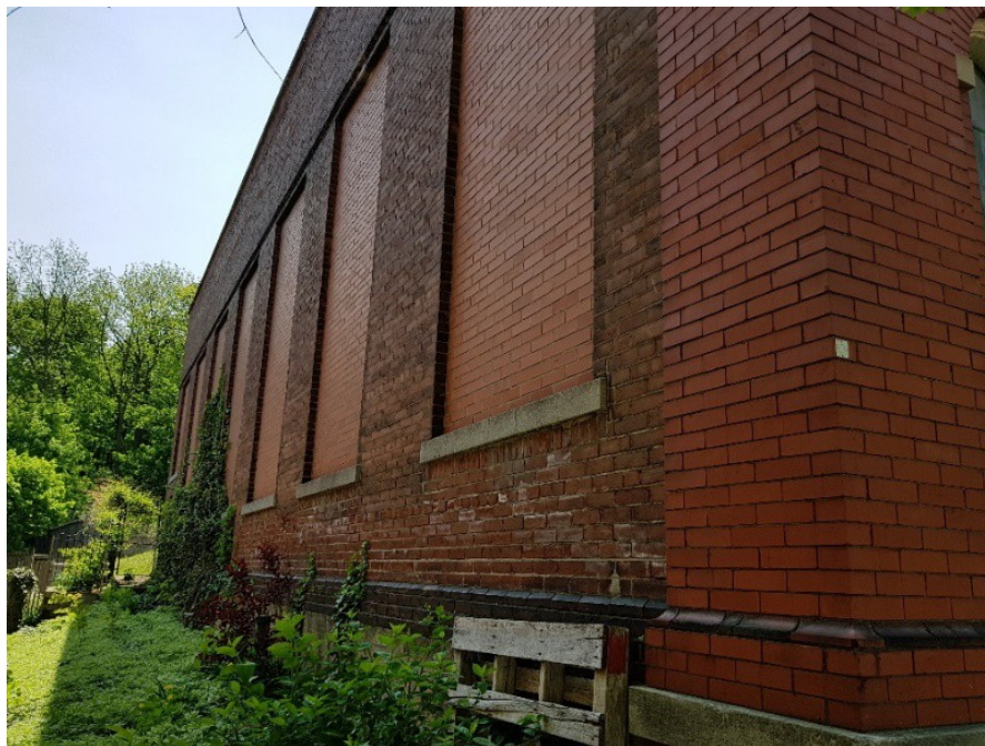
Figure 45: Blind windows and lower quality brick laid in common bond on the north façade. Note also the cogging course above the windows.
