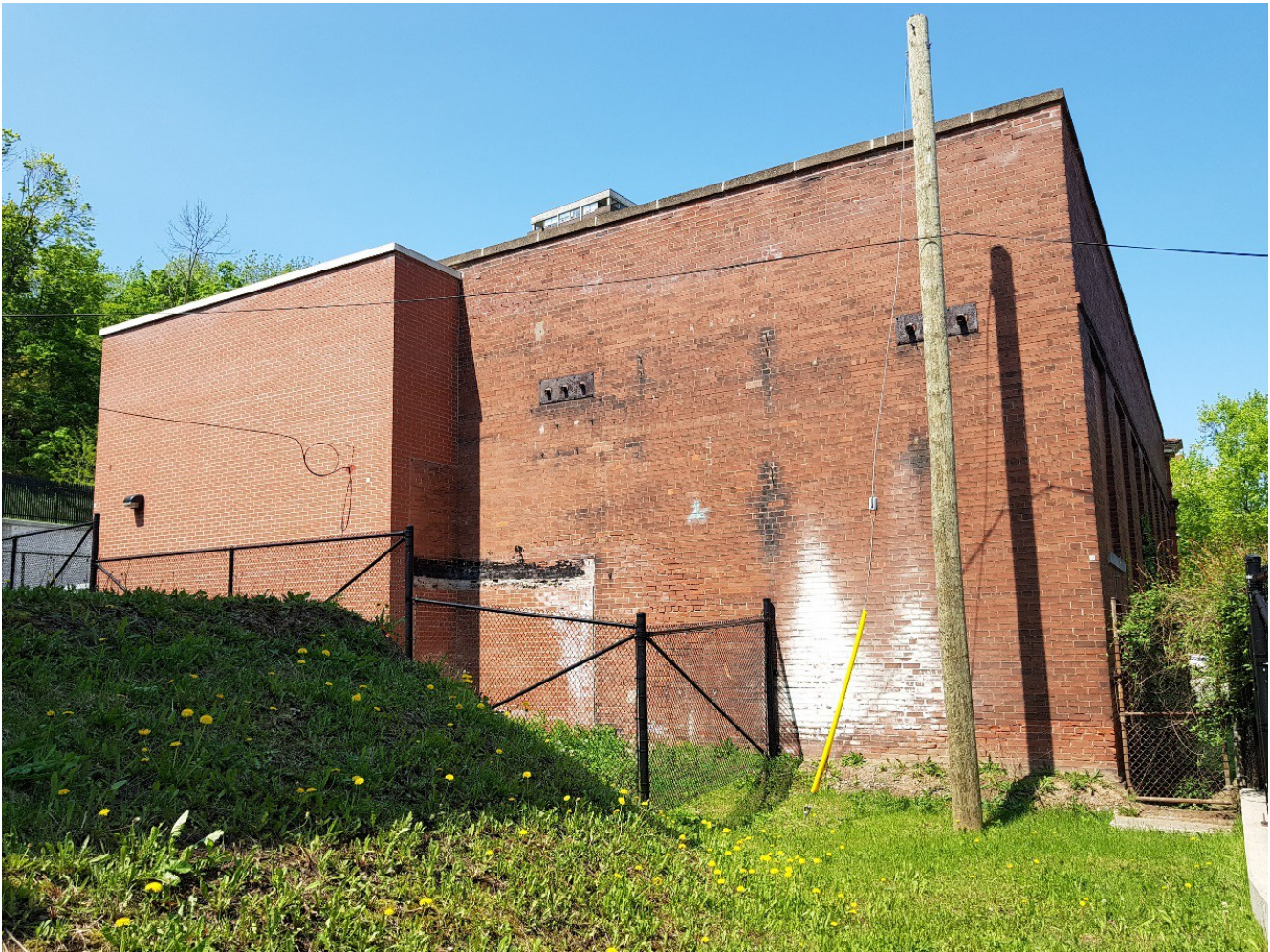
Figure 41: East and north façades (rectified to minimize distortion).
