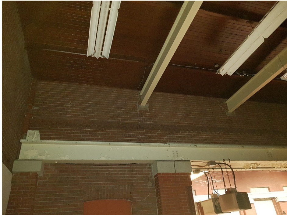
Figure 55: Exterior wall with coggling of the 1912-13 Block as seen from within the 1929-30 Extension.
