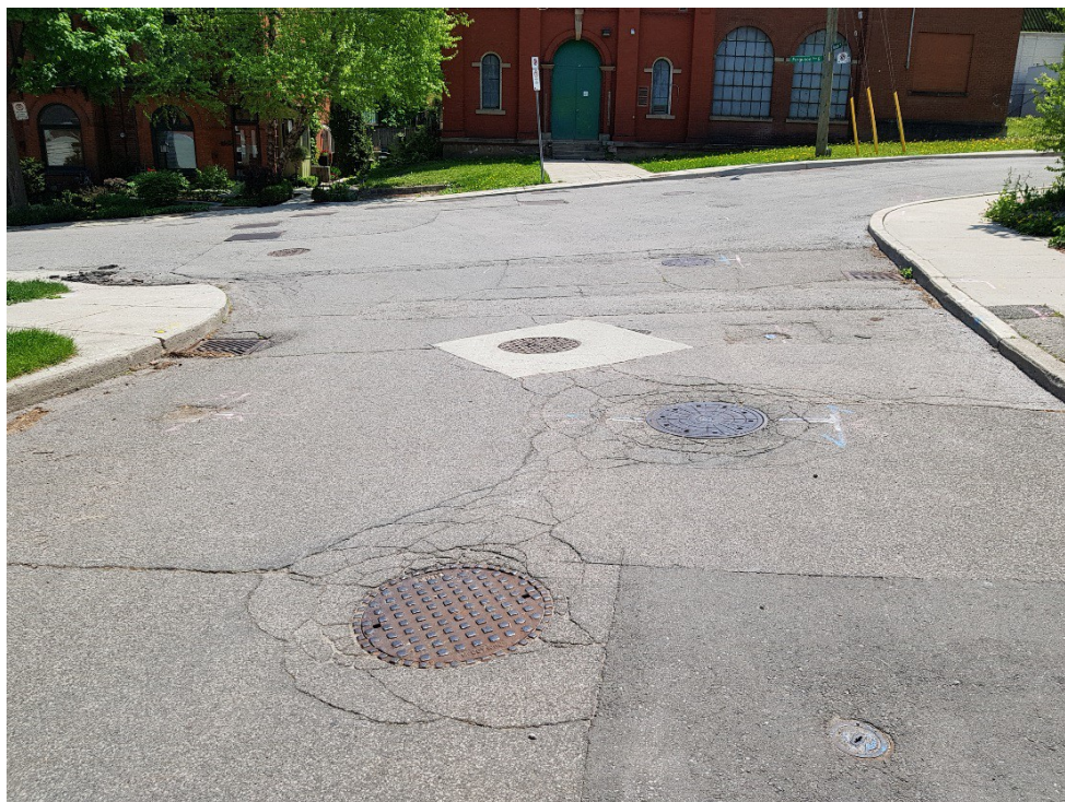
Figure 30: Numerous round and square maintenance covers west of the Ferguson Avenue Pumping Station.
