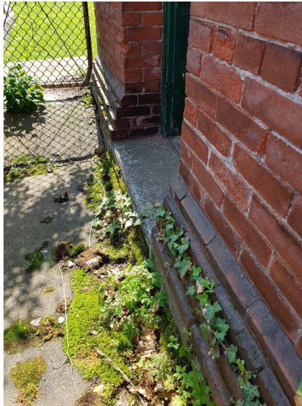
Figure 44: Brick water table at the northeast entrance.
