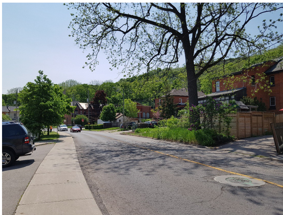
Figure 32: View of the pumping station facing southwest from east on Charlton Avenue East. The 1912-13 and 1929-30 elements of the pumping station are visible at centre.
