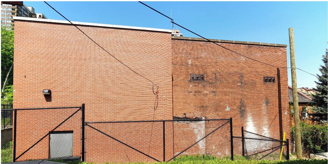
Figure 40: East façade (rectified to minimize distortion).
