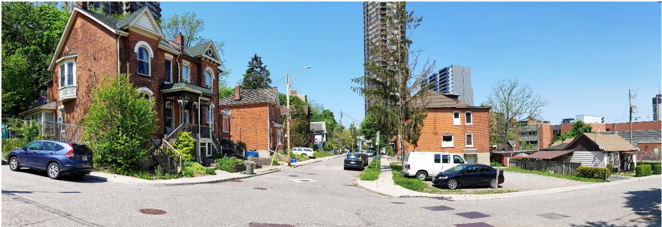
Figure 34: View facing west from the property of Foster Street. Also note the maintenance covers in the foreground.
