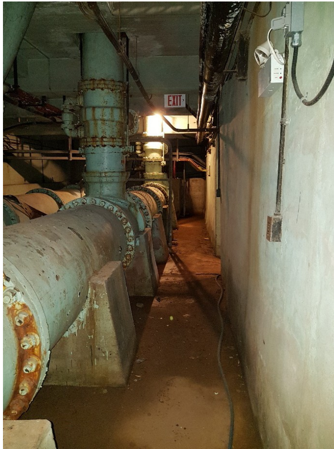
Figure 68: View facing west of the piping beneath the 1929-30 Extension.
