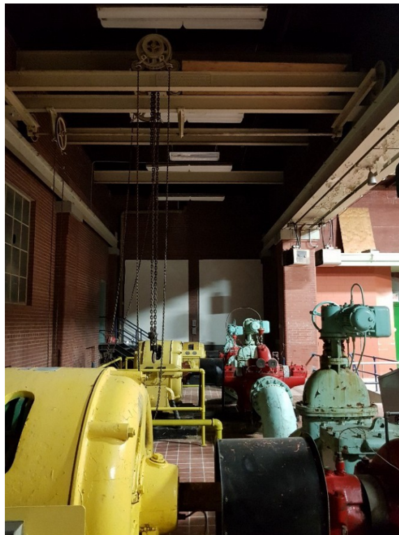
Figure 61: Interior of the 1929-30 Extension, facing west.
