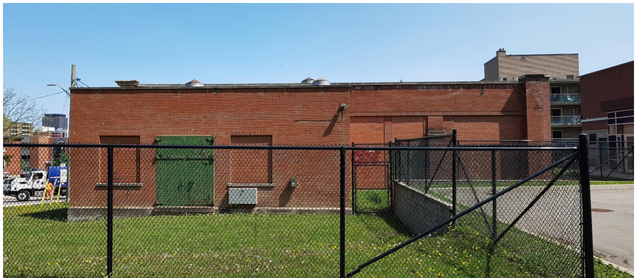
Figure 38: South façade (rectified to minimize distortion).
