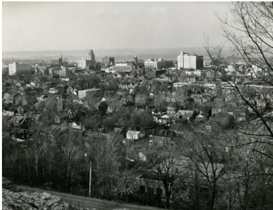
Figure 23: 1963 photo with the now fully expanded Fergusson Avenue Pumping Station in the foreground at bottom right (Local History & Public Archives Hamilton Flickr 2018).
