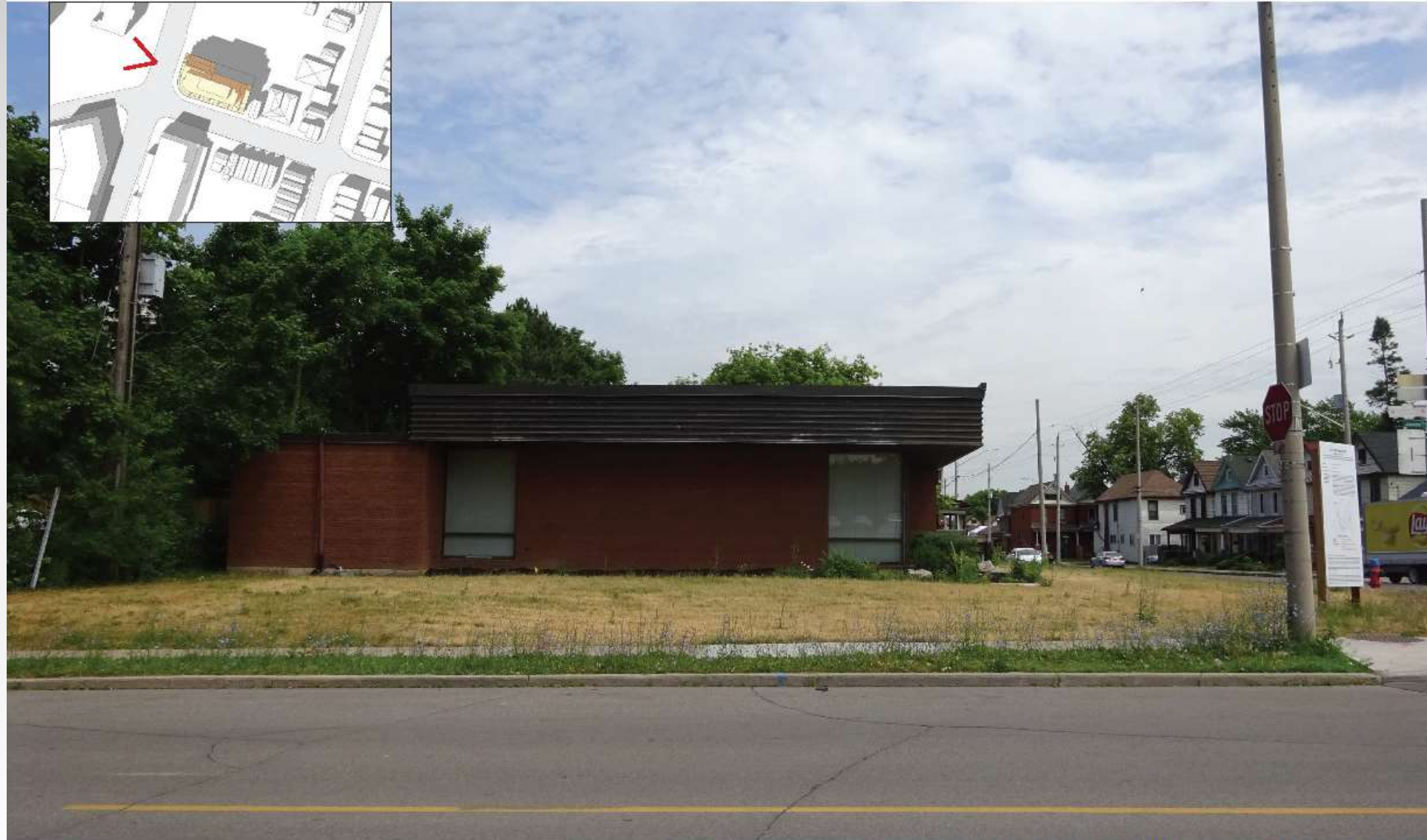
SUBJECT SITE: VIEW LOOKING EAST
