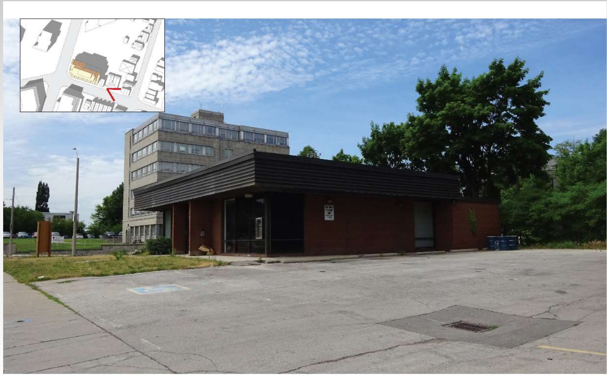
SUBJECT SITE: VIEW LOOKING WEST
