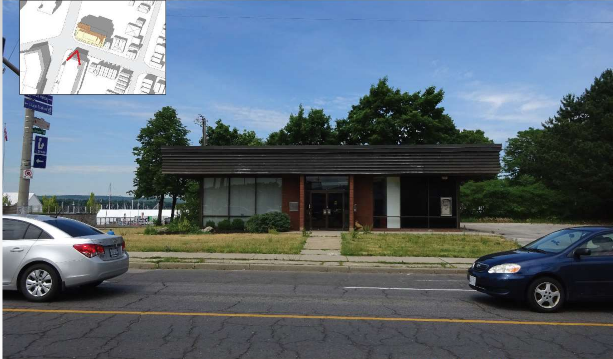
SUBJECT SITE: VIEW LOOKING NORTH
