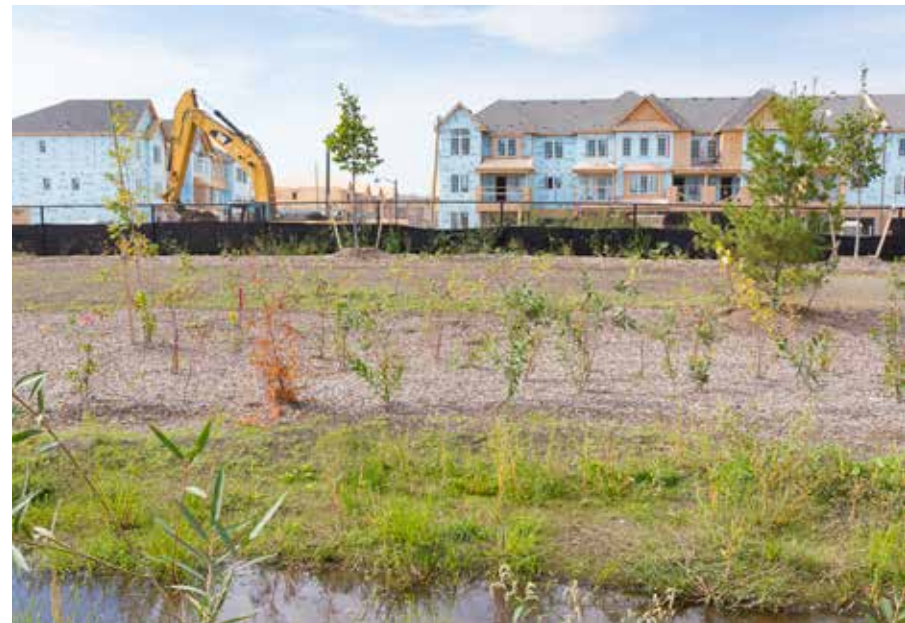
Conservation Halton regulates development adjacent to creeks, streams, rivers, wetlands and shorelines, such as this neighbourhood in North Oakville, pictured during construction.
